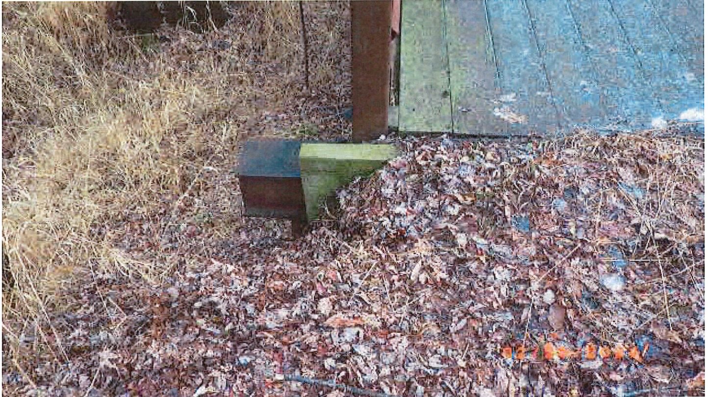
Fix Erosion NE corner.
