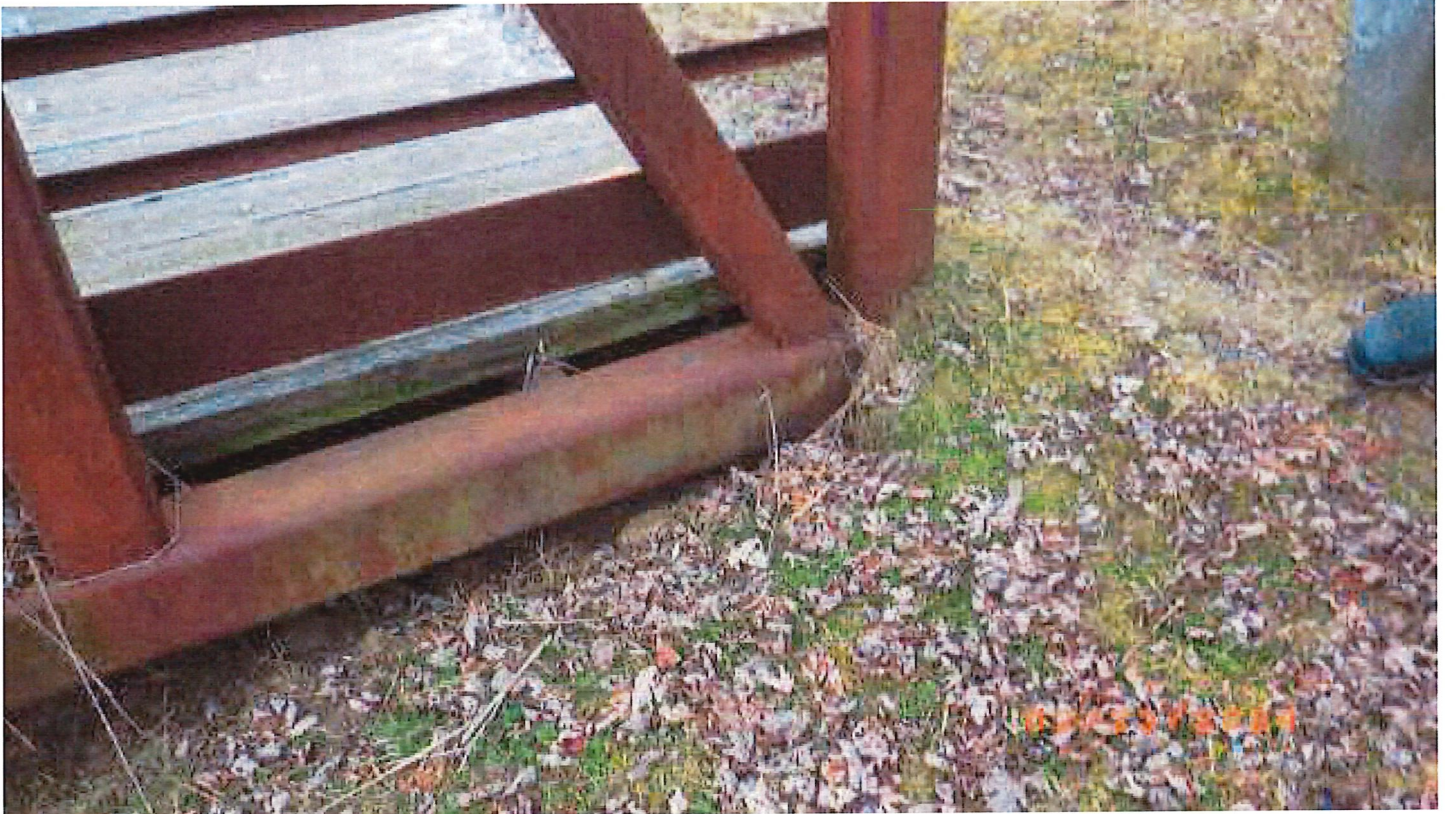
NW bearing, clean as it is buried, which is bad.
