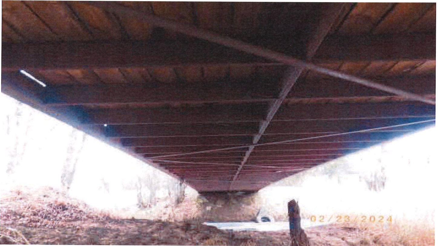
Bottom of deck, with debris in deck.
