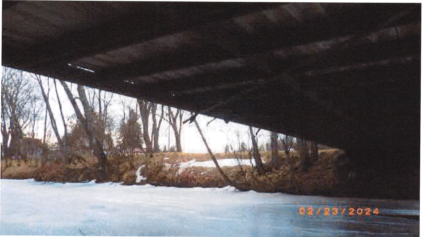
Damage cross bracing with debris in deck.
