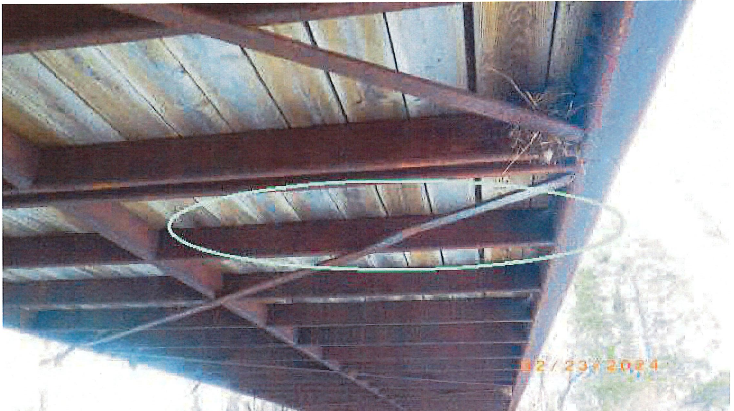
Damage cross bracing with debris in deck.
