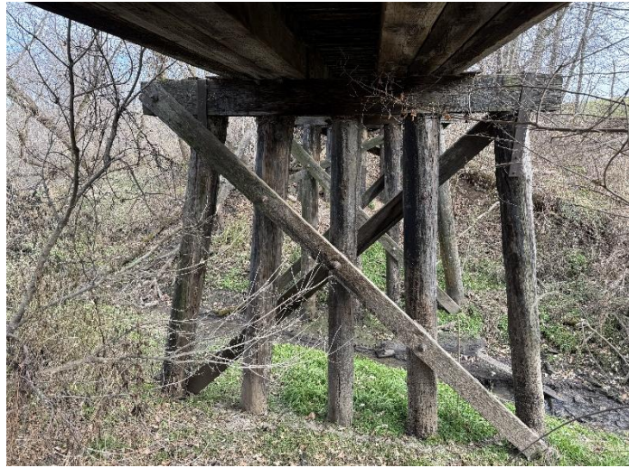
Photo 7 – Pier W2 Looking East.
