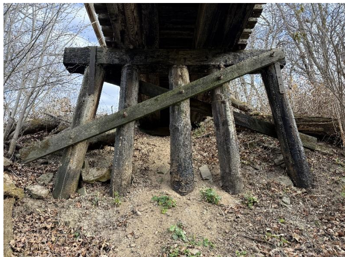
Photo 11 – Pier W4 Looking East.
