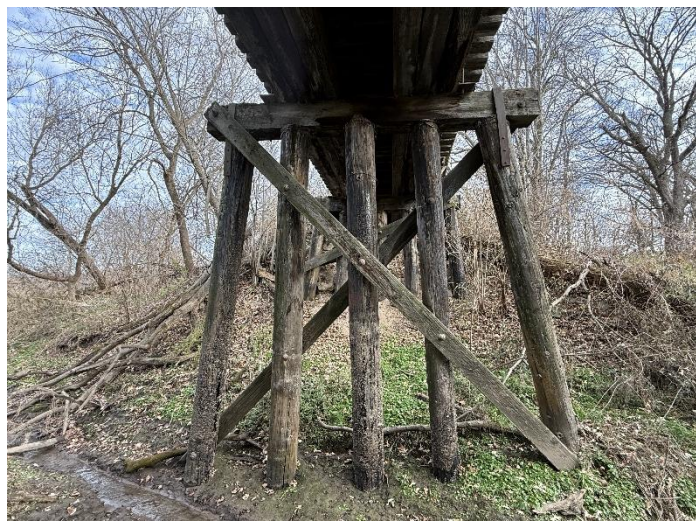
Photo 9 – Pier W3 Looking East.
