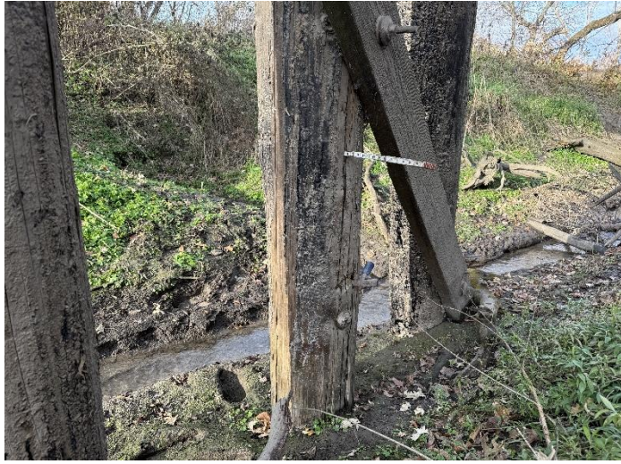
Photo 13 – Pier W3-Pile S4.
