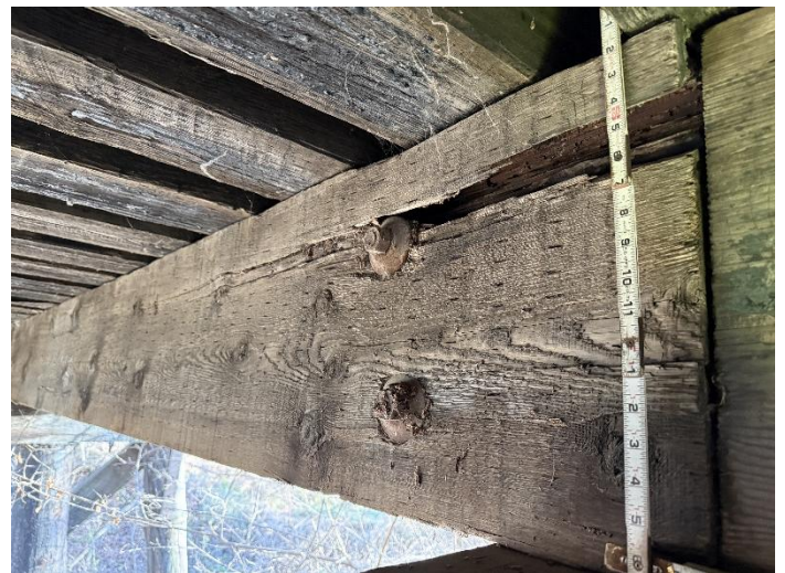
Photo 16 – S. BM-N.F.-Span 2 Over Pier W1 Looking W.
