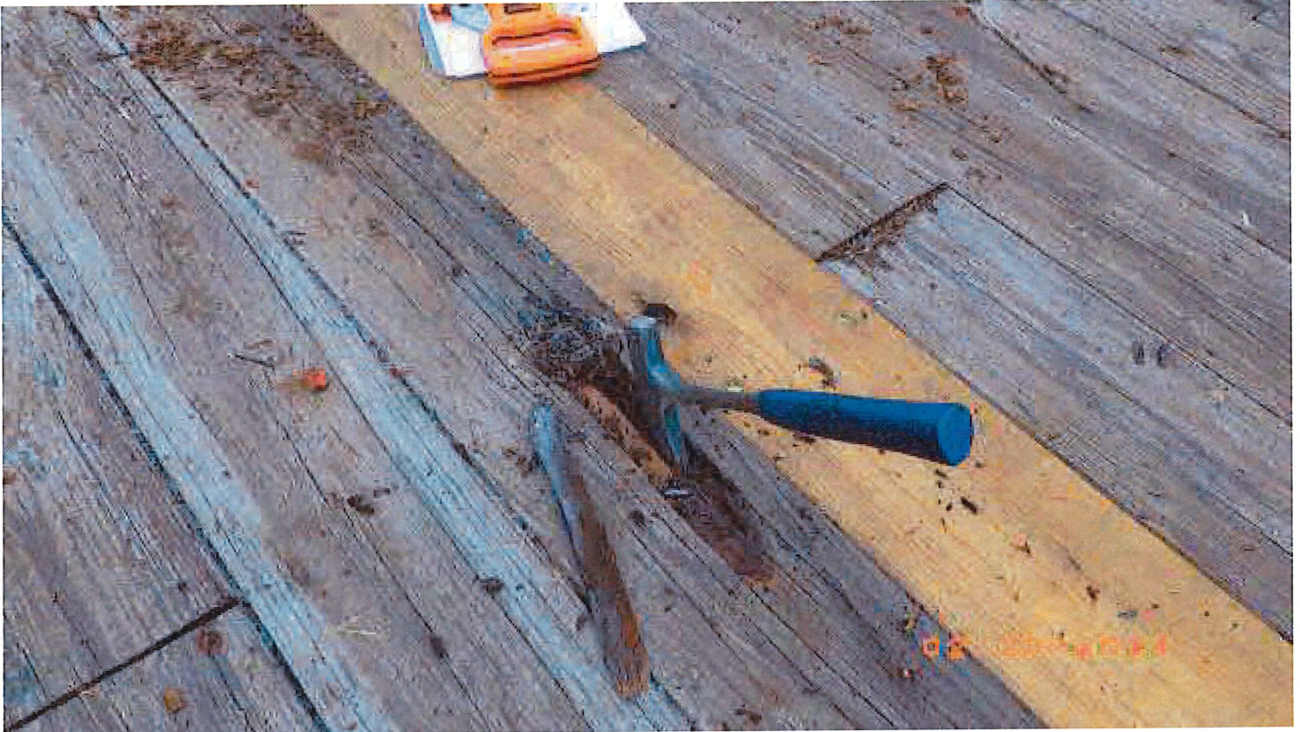
Deck Rot, measurable section loss.
