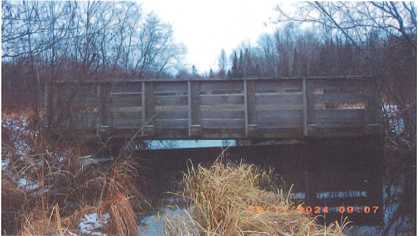
Elevation view from upstream
