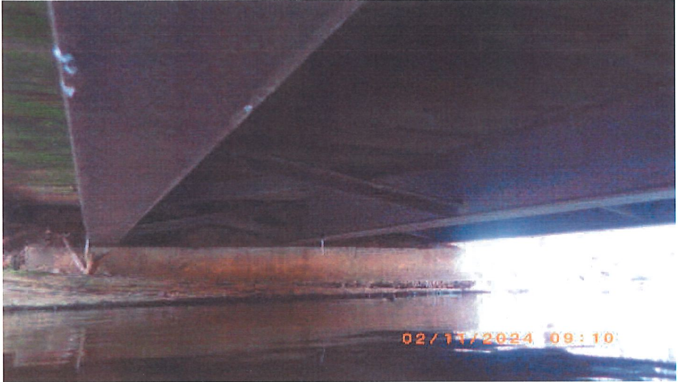
Typical underside of superstructure / x bracing at ends plus 1/4 pts
