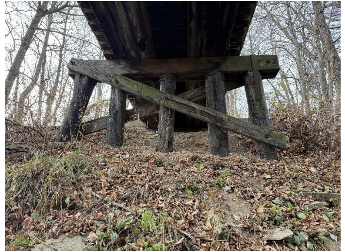
Photo 14 – Pier W1 Looking West.
