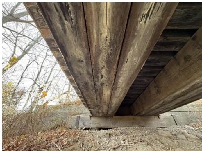
Photo 17 – West Span-South Beam Looking East.
