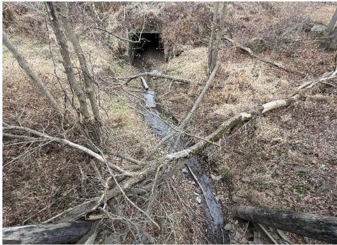
Photo 3 – Upstream Looking South.
