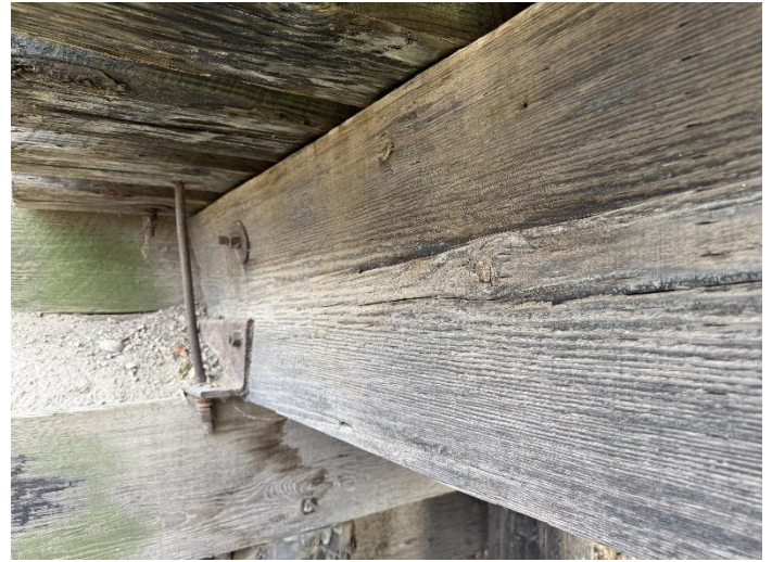
Photo 8 – North Beam/North Face Over E. Abutment.
