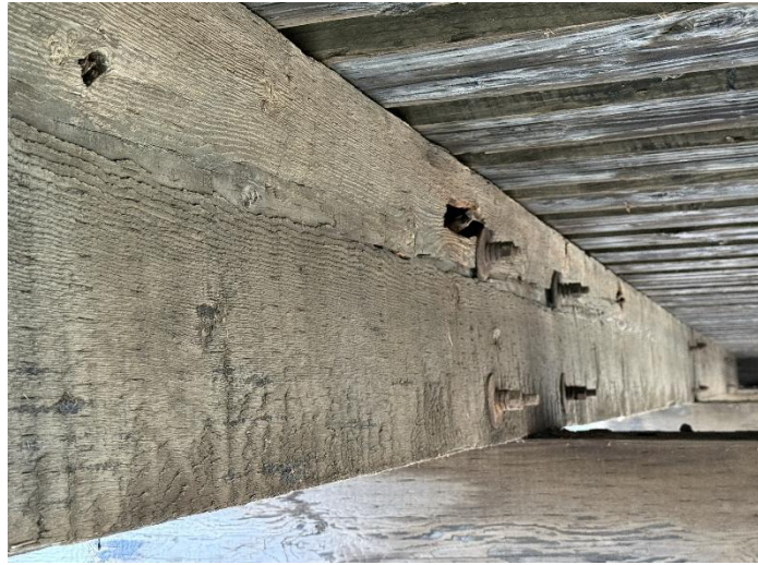
Photo 7 – South Beam/North Face Over East Pier.
