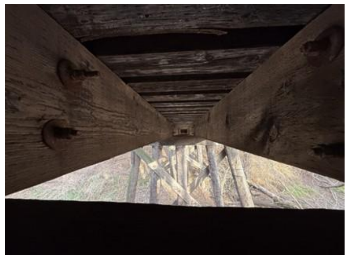
Photo 18 – Span W2 Looking East.
