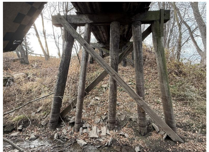
Photo 12 – Pier W2 Looking West.
