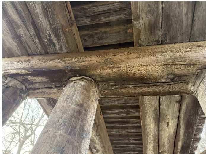
Photo 9 – Pier W3 Cap-Piles S2-S4.
