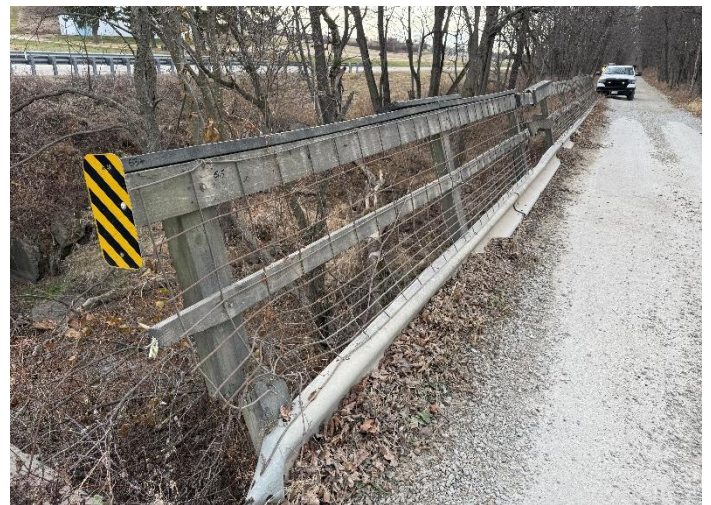
Photo 6 – South Rail Looking West.
