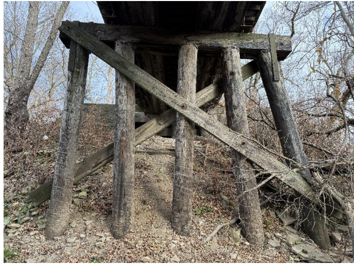
Photo 13 – Pier W3 Looking East.
