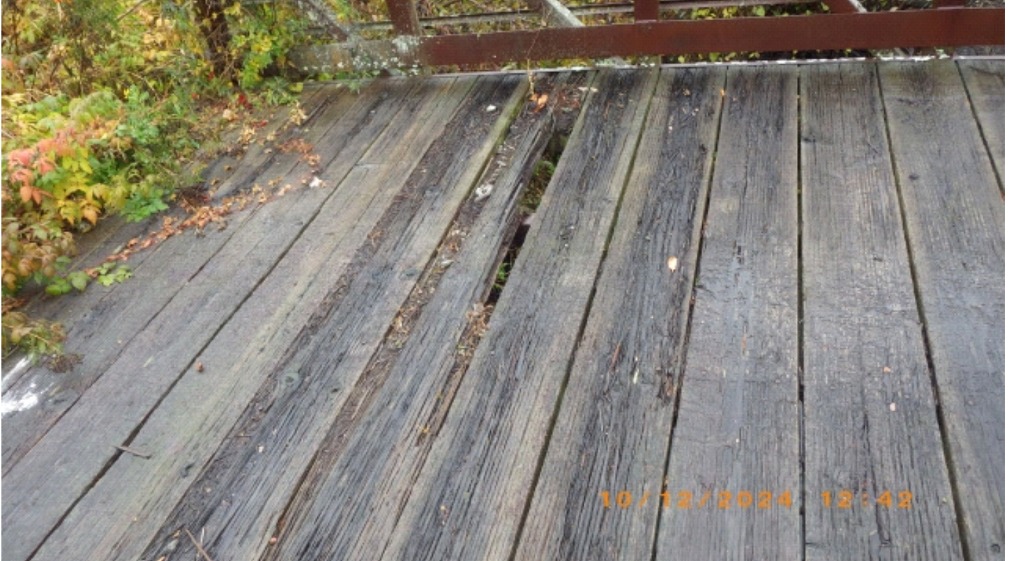
CS4 rotten deck planks
