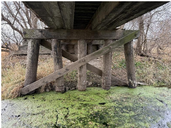
Photo 15 – West Pier Looking West.
