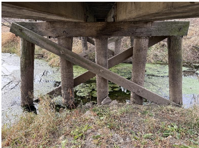
Photo 17 – East Pier Looking West.
