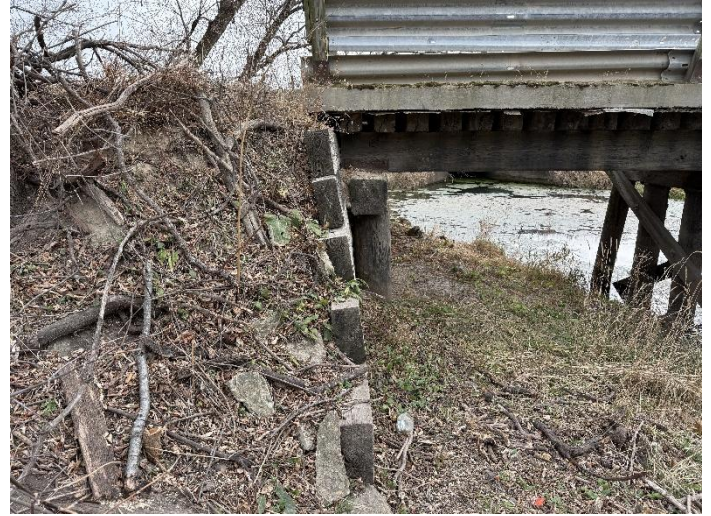
Photo 20 – East Abutment Looking South.
