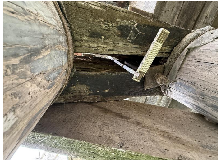
Photo 12 – West Pier Cap-Piles W5-W4.
