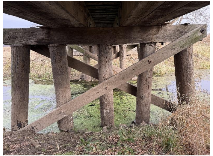
Photo 14 – West Pier Looking East.
