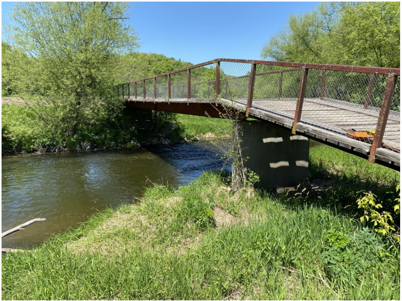
Shows the I-Beam on this side also plated together.
