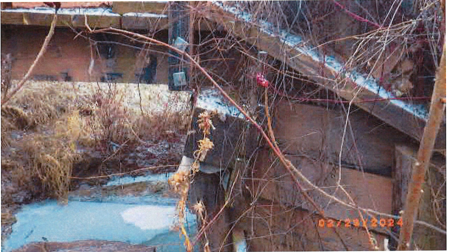
Rotated West Pile cap, looking South
