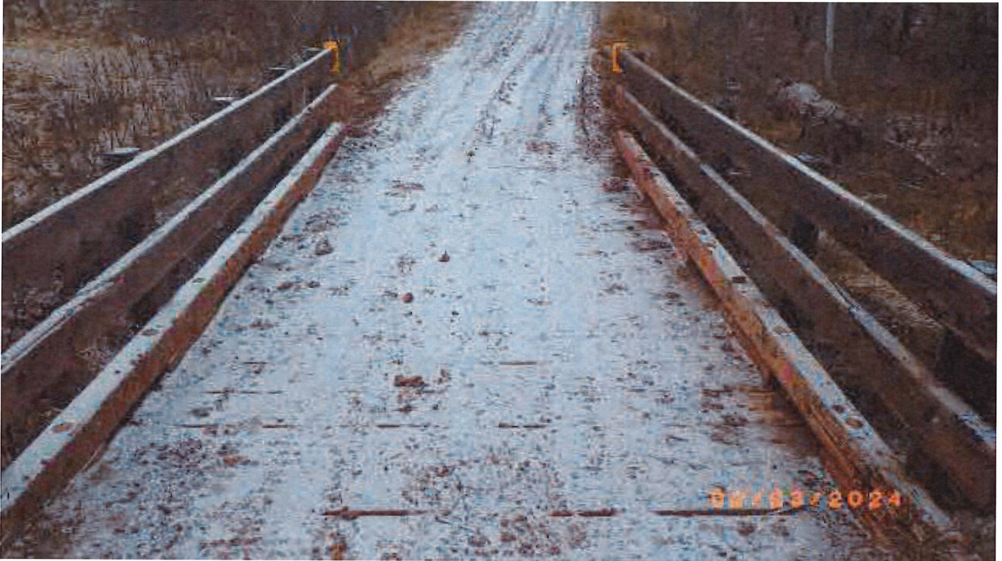
Top of deck and rails.
