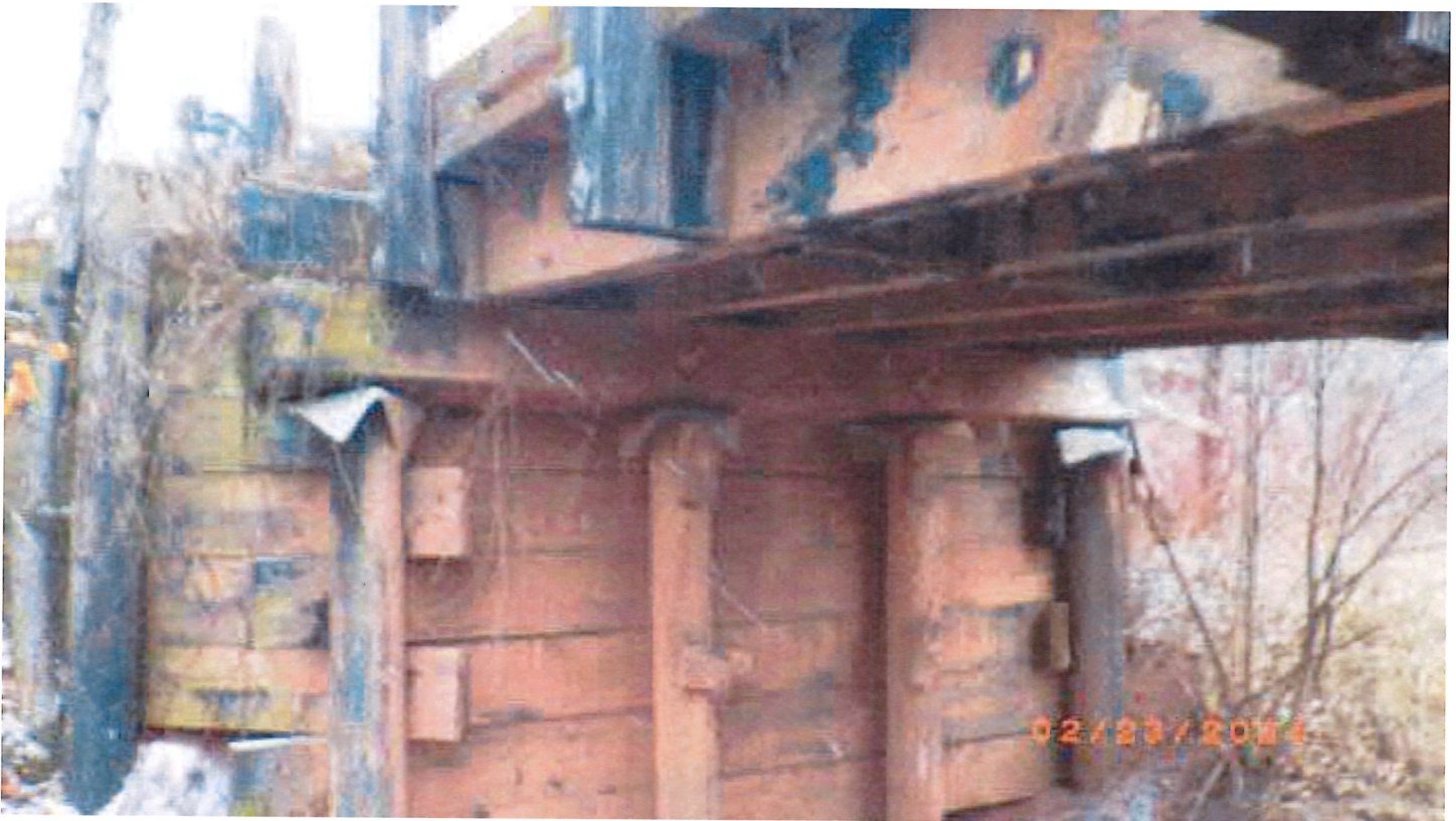
East Pile cap not touching 90% of the length.
