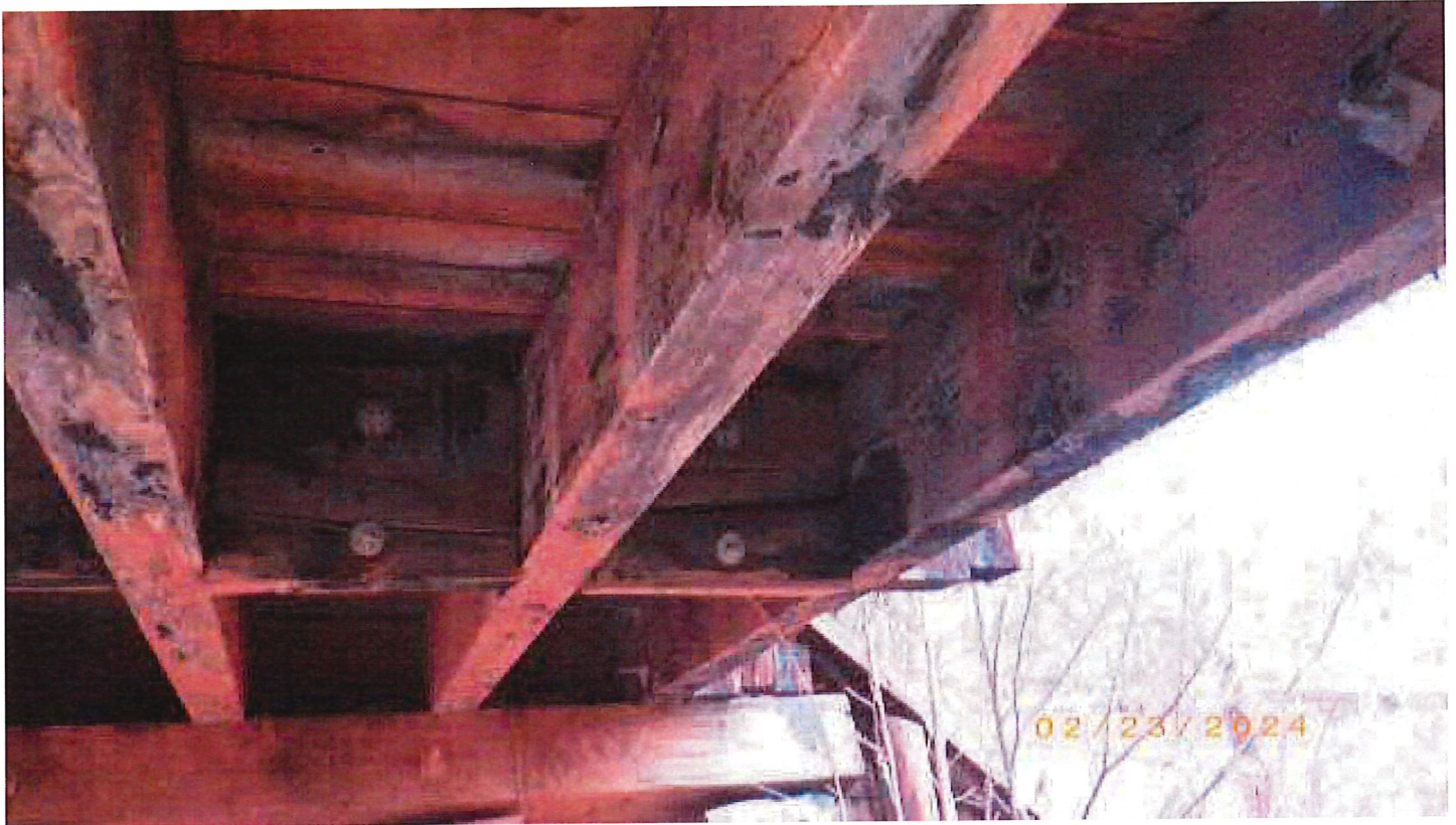
Busted Diaphragm, East line, South end.
