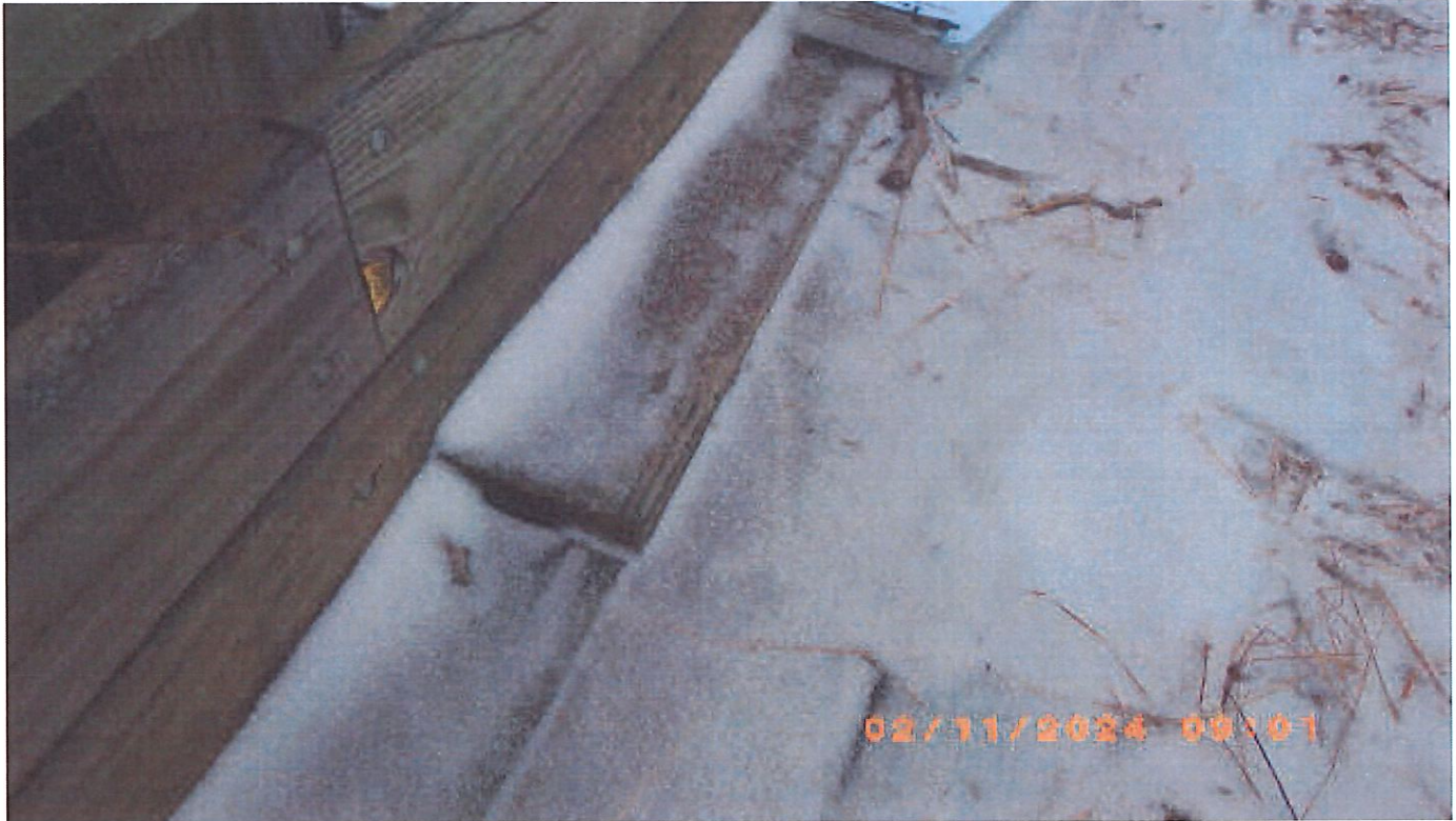
Wear plank loose and coming up
