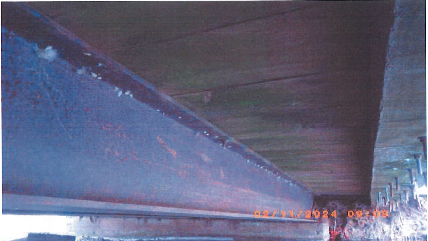
Typical underside of deck / green mold
