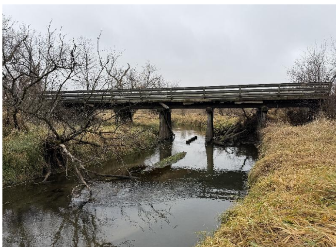
Photo 5 – Side View Looking South.
