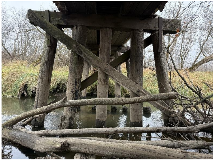
Photo 13 – Pier W2 Looking East.
