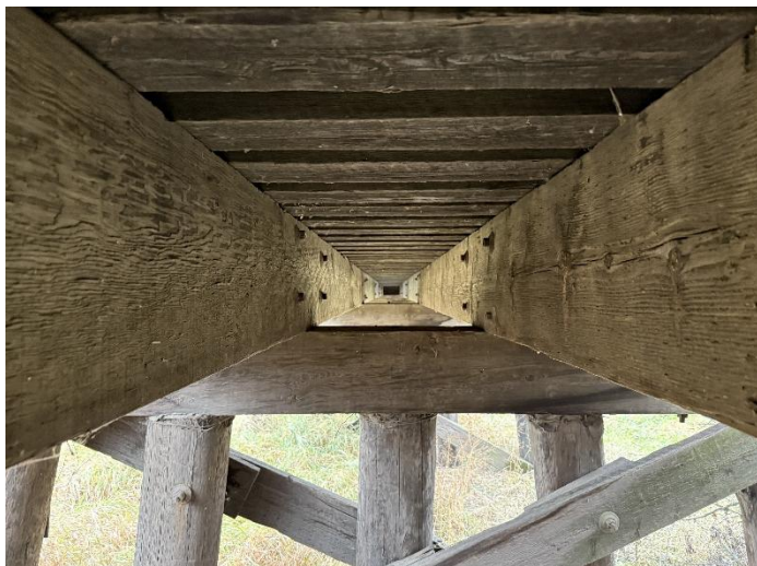
Photo 29 – Underside Looking West Near Pier W5.
