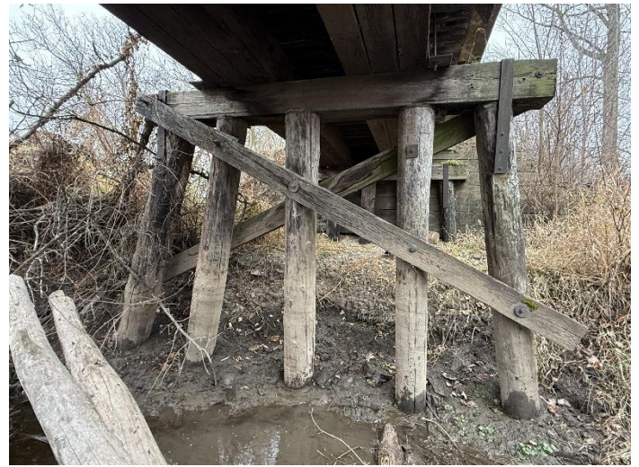
Photo 14 – Pier W1 Looking East.
