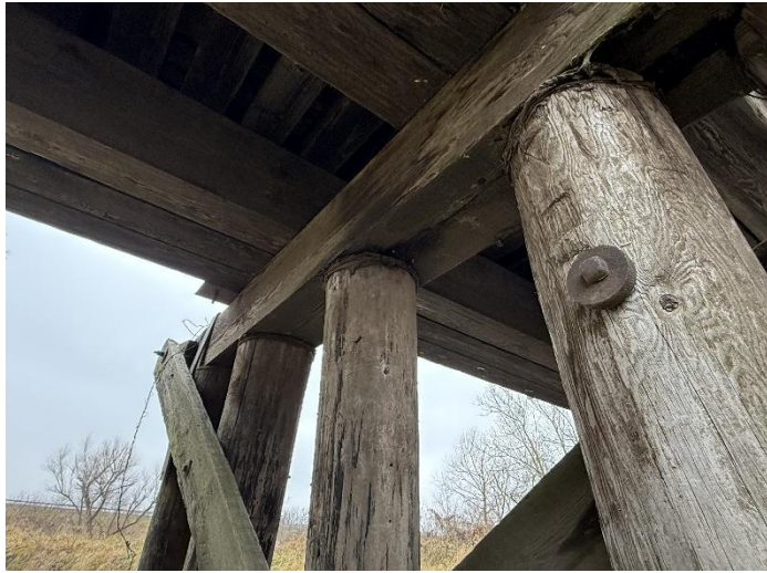
Photo 25 – Pier W4-Piles S1-S4.
