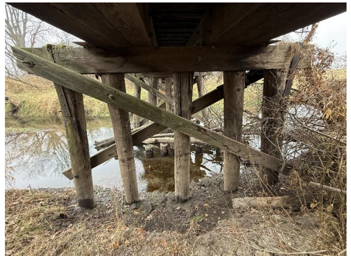
Photo 10 – Pier W1 Looking East.
