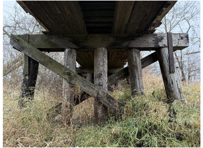
Photo 26 – Pier W5 Looking East.
