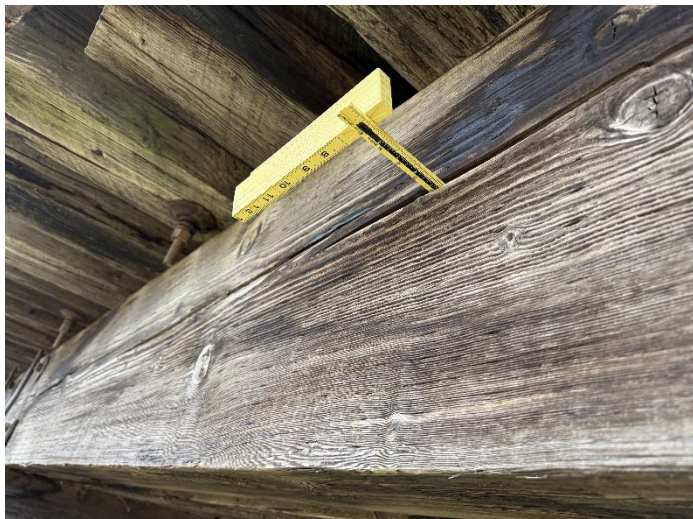
Photo 27 – Span W5-South Beam.
