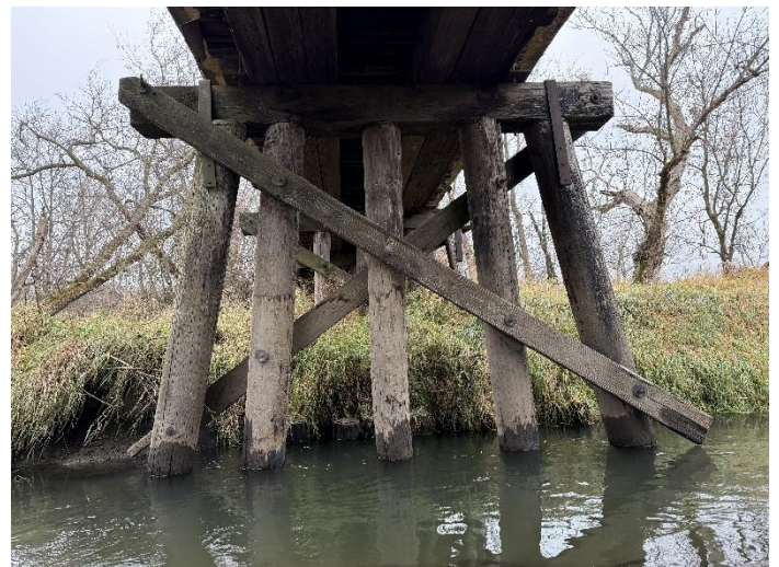
Photo 18 – Pier W3 Looking East.
