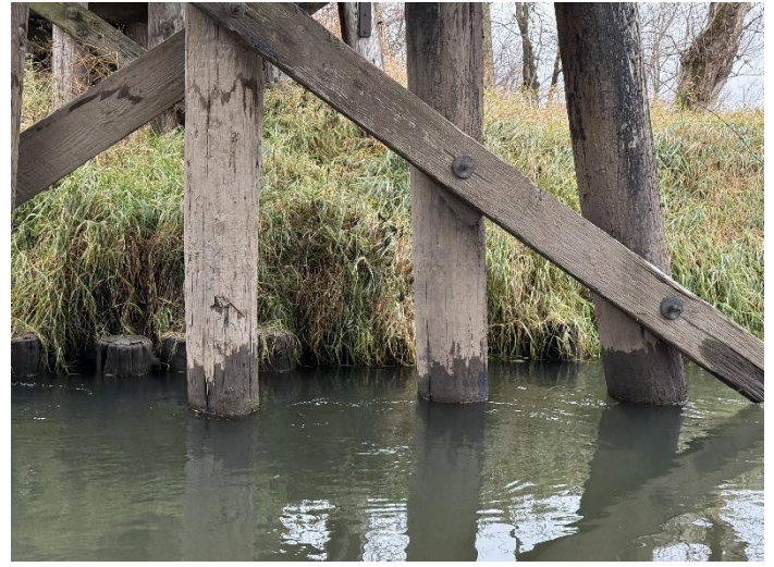
Photo 20 – Pier W3 Looking East Piles W3-W1.
