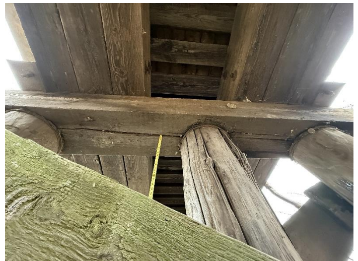
Photo 12 – Pier W1-Cap Over Pile S3.
