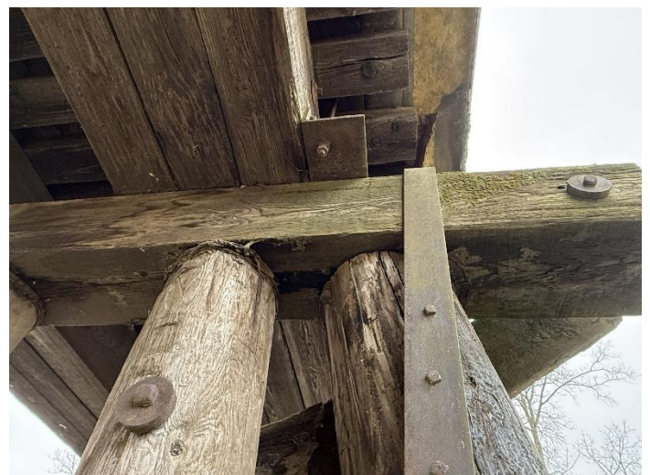
Photo 24 – Pier W4-Piles S4-S5.
