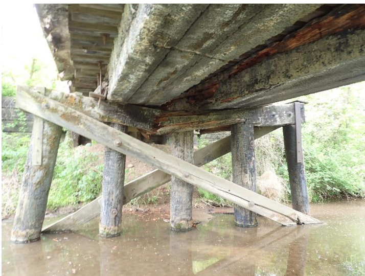
Photo 8 – Pier E1 Looking East
