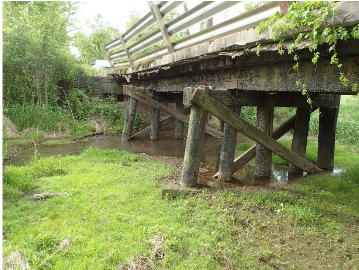
Photo 2 – Side View Looking Southeast
