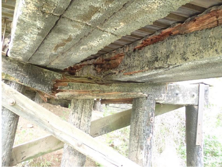
Photo 9 – Pier E1 Looking East
