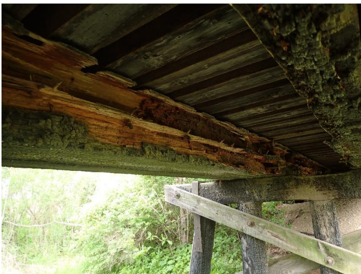
Photo 5 – Span E3 Looking West
