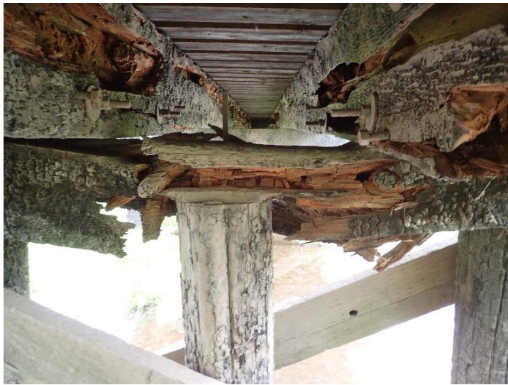
Photo 10 – Pier E1 Looking West
