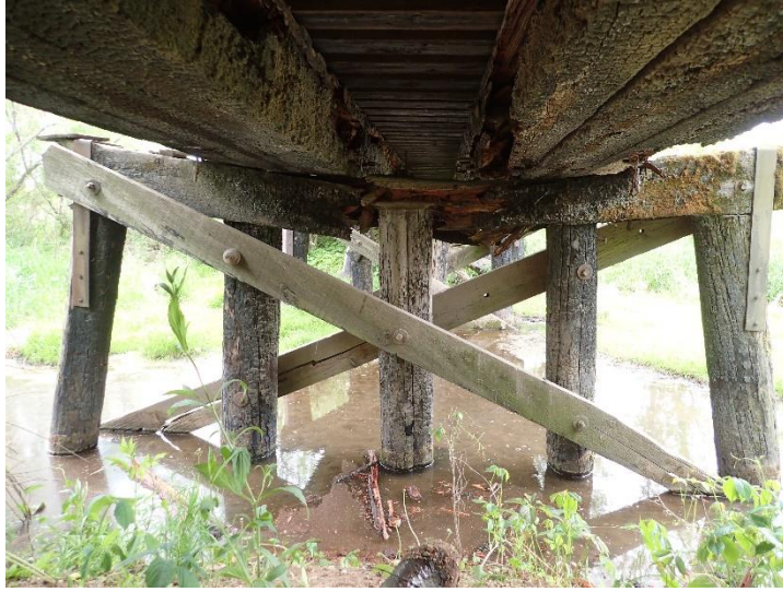
Photo 12 – Pier E1 Looking West
