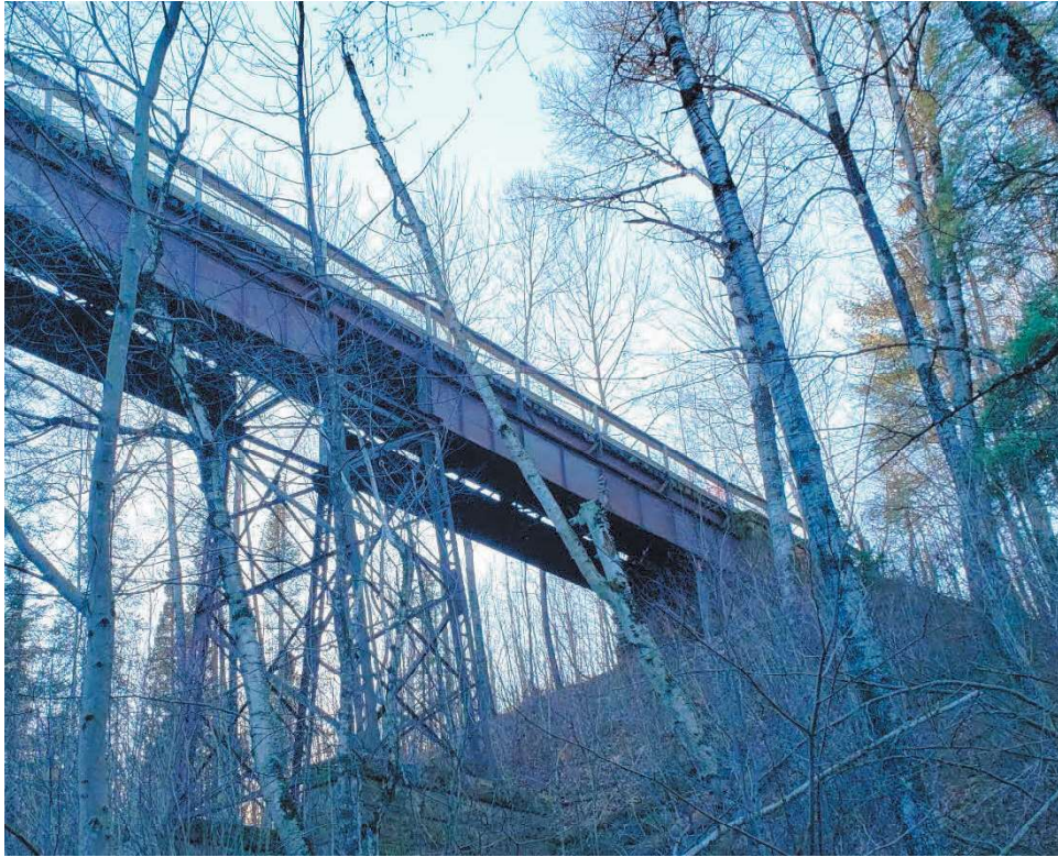
Picture: 01/24 Span 1 Deck Plate Girders. SW Facing.
