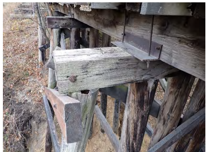
Photo 32 – Pier W3 Looking West.
