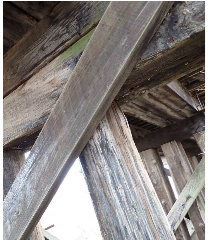
Photo 54 – Pier W7-Pile S5.
