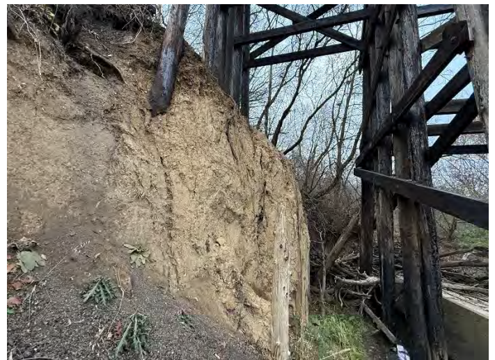
Photo 14 – West Embankment Looking North.
