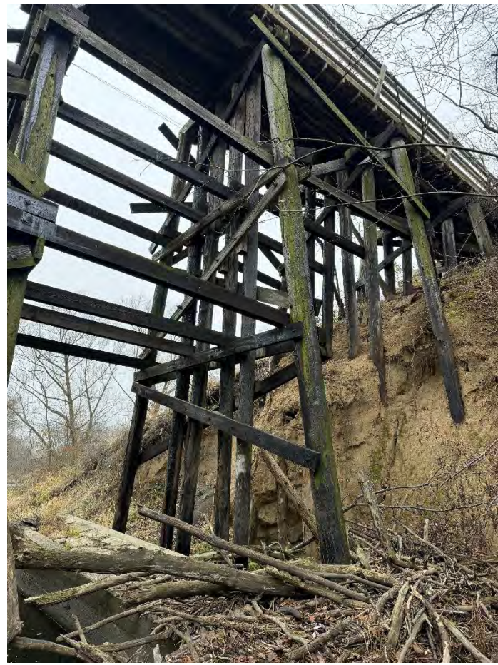
Photo 11 – West Embankment Looking Southwest .
