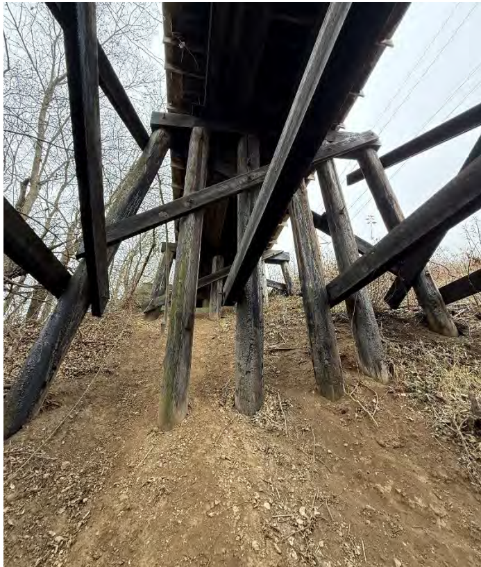
Photo 59 – Pier W9 Looking East.
