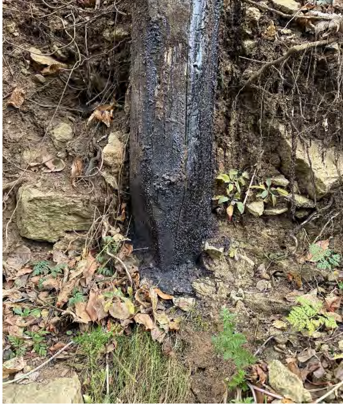
Photo 49 – Pier W7-Pile S2.
