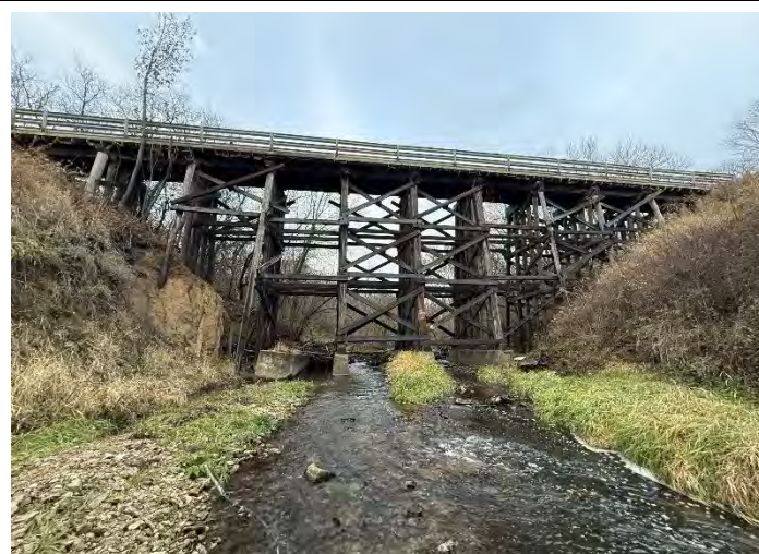
Photo 5 – Side View Looking North.
