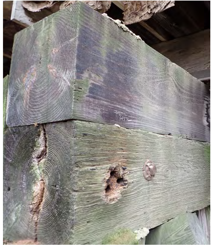
Photo 58 – Pier W8 Cap-North End.
