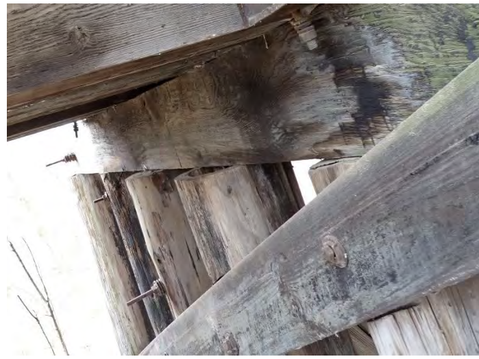
Photo 27 – Pier W1 Looking Southwest.
