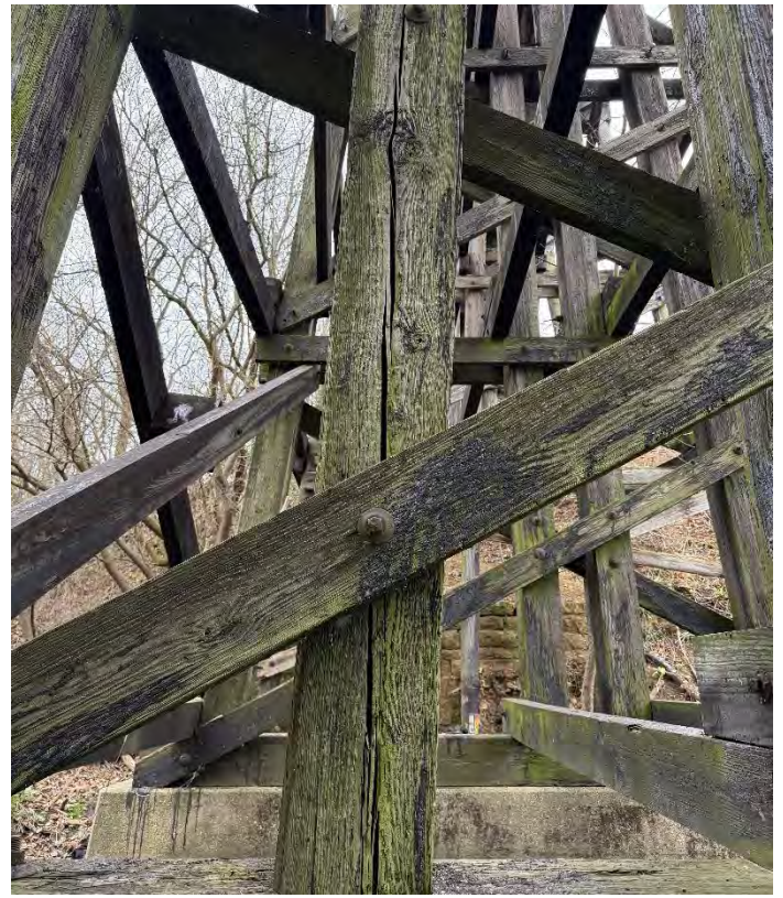
Photo 38 – Pier W5-Pile S5 Looking East.
