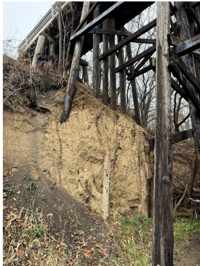
Photo 9 – West Embankment Looking East.
