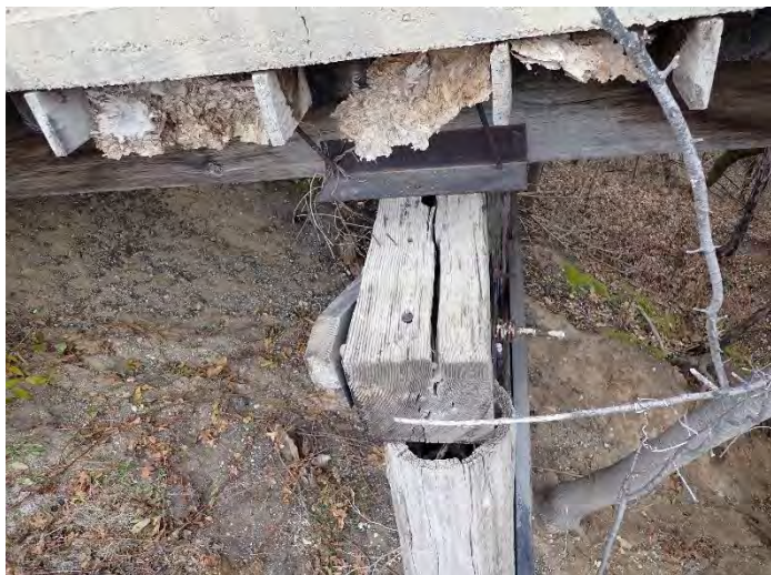
Photo 25 – Pier W1 Cap-South End.
