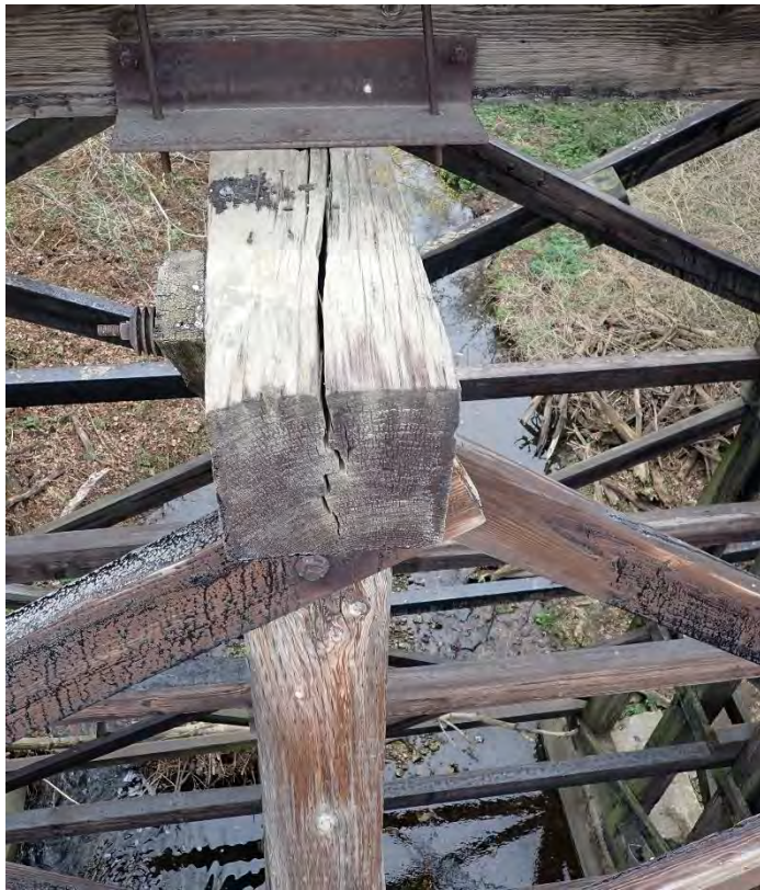
Photo 39 – Pier W5 Looking North.
