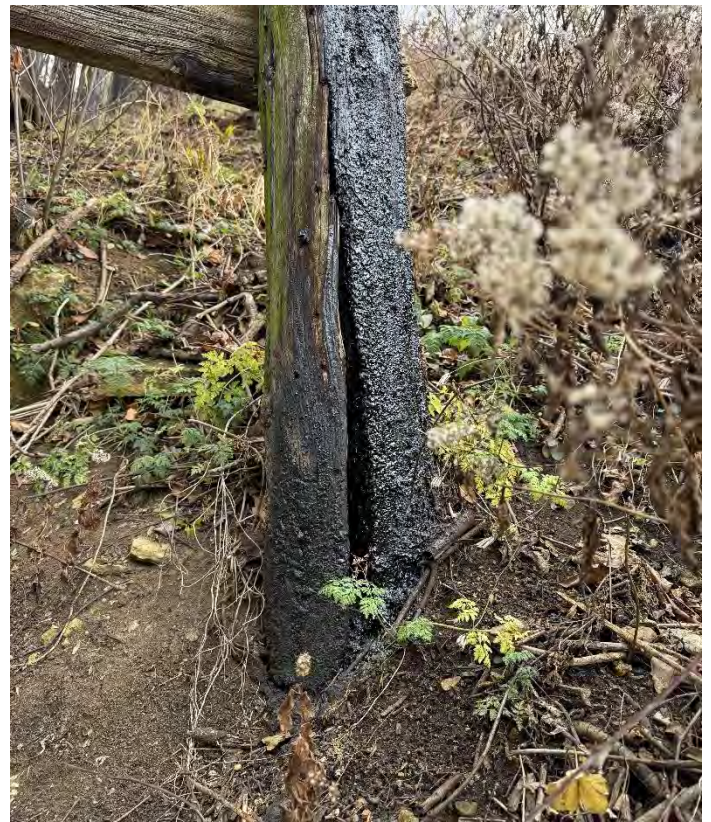
Photo 48 – Pier W7-Pile S1.
