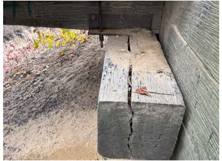
Photo 16 – West Abutment Cap Looking South.
