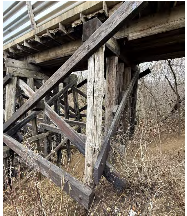
Photo 62 – Pier W9 Looking North.
