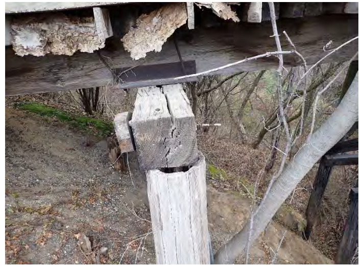
Photo 28 – Pier W1 Looking North.
