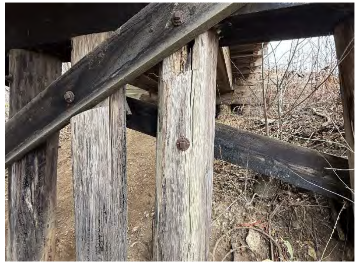
Photo 68 – Pier W10-Pile S2.
