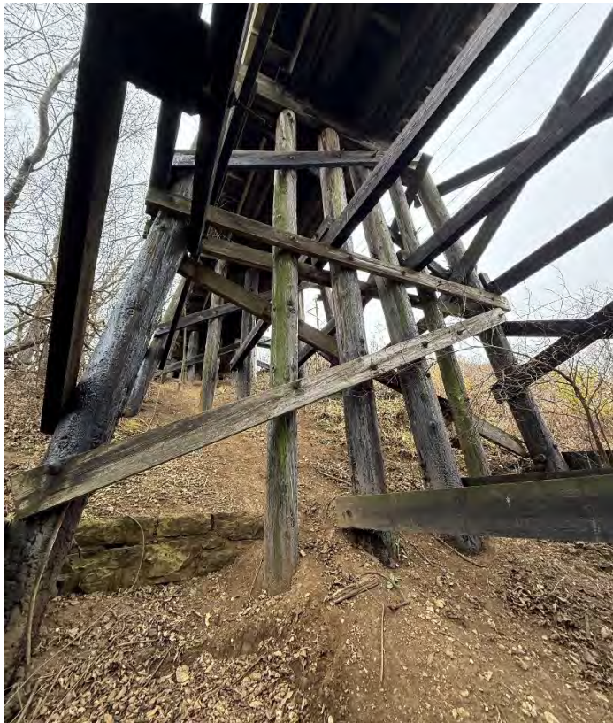
Photo 55 – Pier W8 Looking East.
