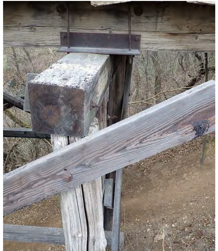
Photo 64 – Pier W9-Pile S1.
