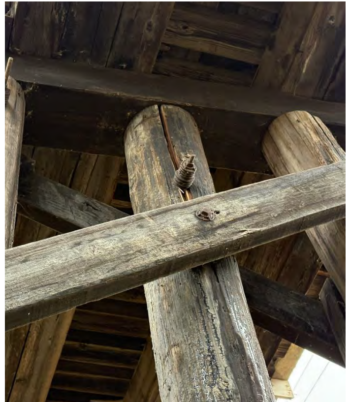
Photo 60 – Pier W9-Pile S4.
