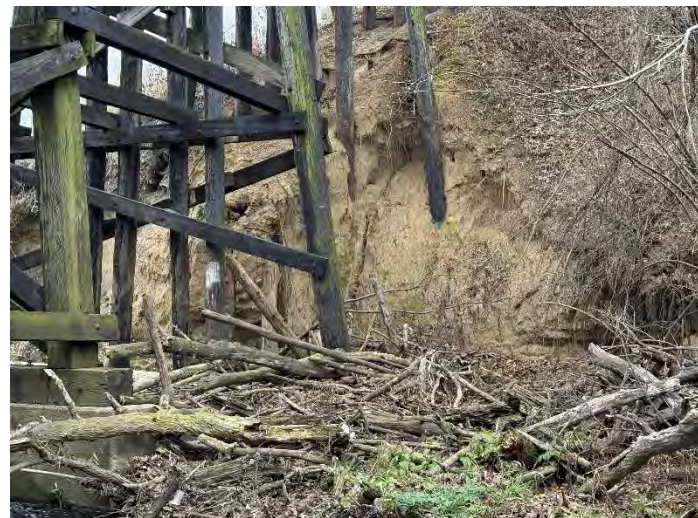
Photo 13 – Northwest Embankment Looking East.
