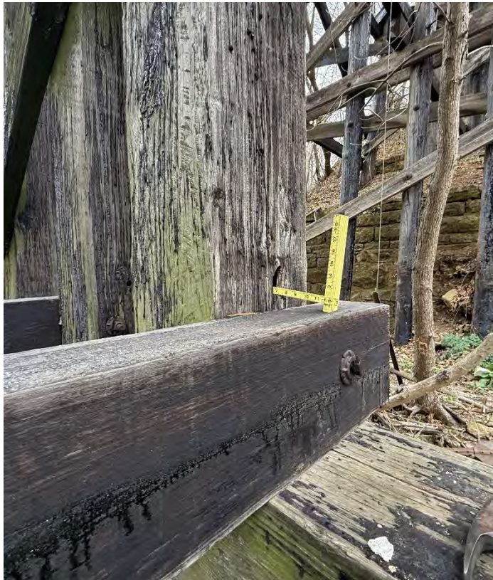
Photo 43 – Pier W6-Pile S3.
