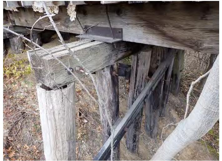
Photo 24 – Pier W1 Looking Northwest.
