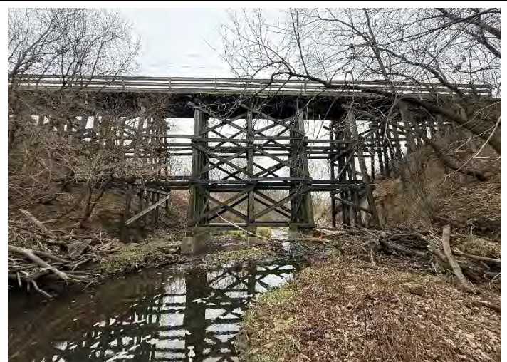
Photo 6 – Side View Looking South.
