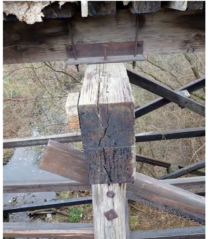
Photo 52 – Pier W7 Looking North.
