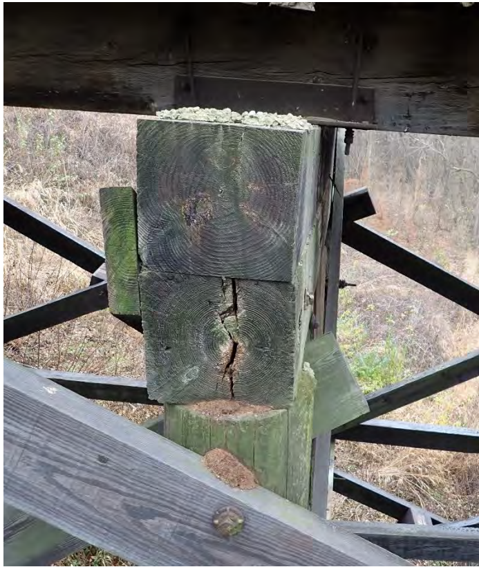
Photo 57 – Pier W8 Cap-North End.
