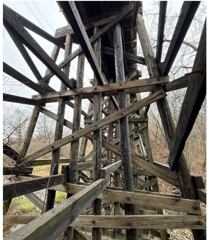
Photo 56 – Pier W8 Looking West.
