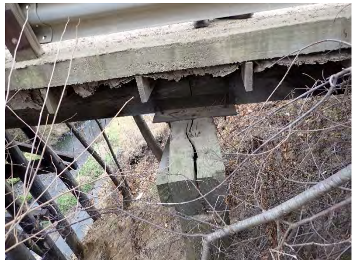
Photo 26 – Pier W1 Cap-North End.
