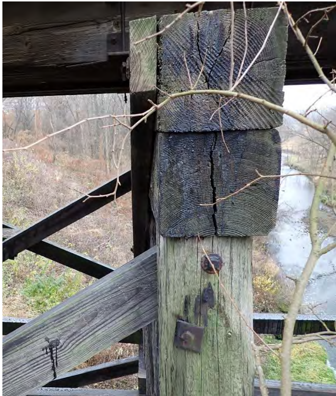
Photo 51 – Pier W7 Looking South.
