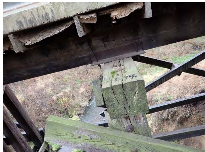
Photo 31 – Pier W3 Looking South.
