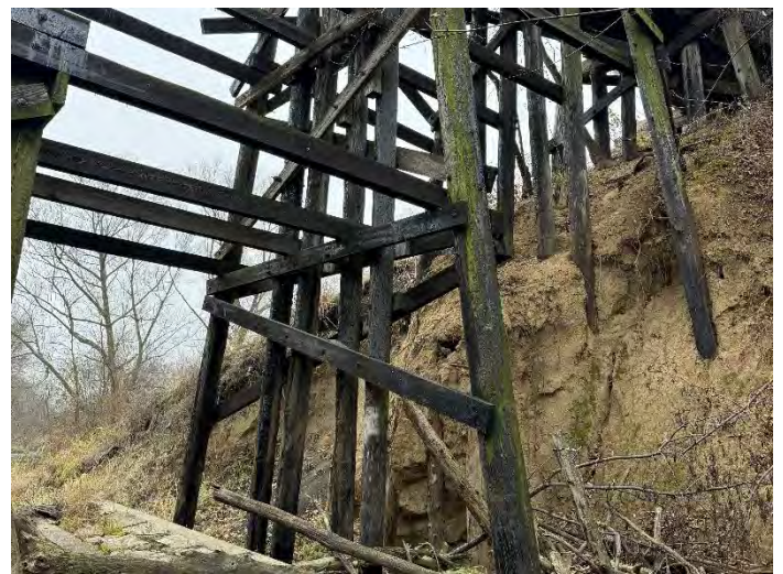
Photo 30 – Pier2 W3-W2 Looking Southwest.
