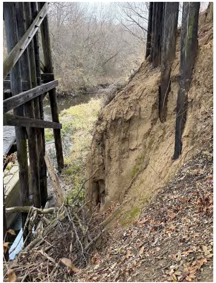
Photo 12 – East Embankment Looking South.
