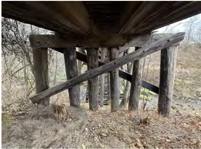
Photo 23 – Pier W1 Looking East.
