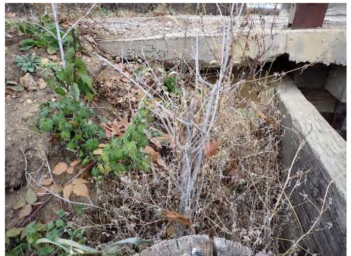
Photo 20 – West Approach Looking North.
