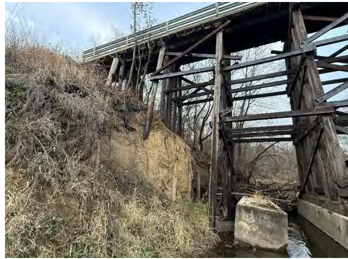
Photo 7 – West Embankment Looking North.
