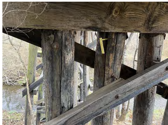
Photo 29 – Pier W1-Pile S5-S3.
