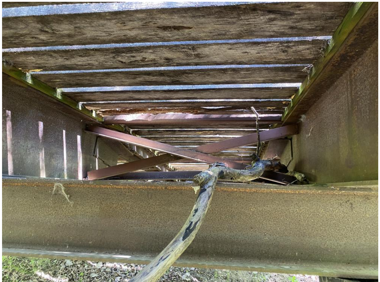
Ramp Attachment and crossmembers on inside
