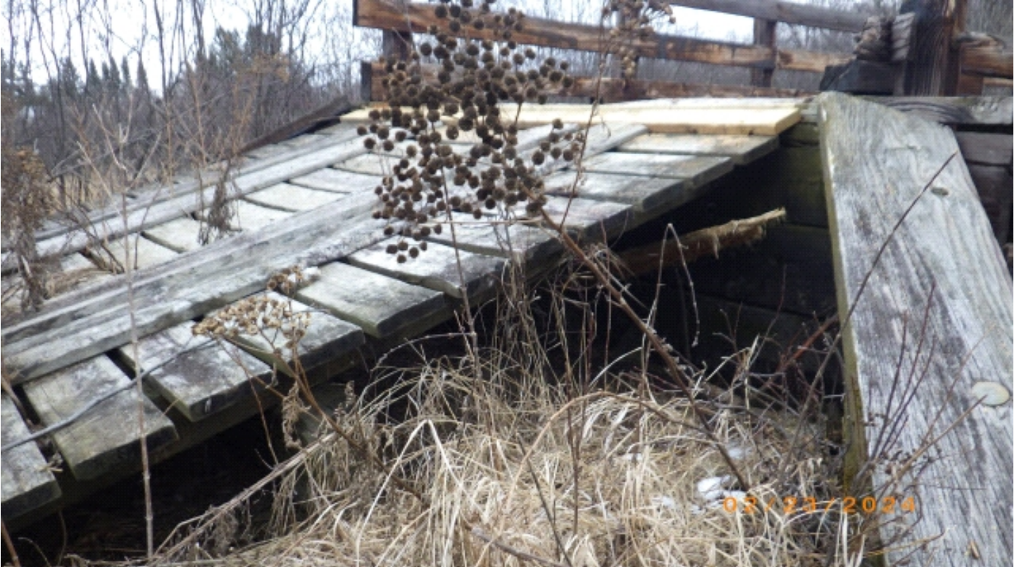
West approach span
