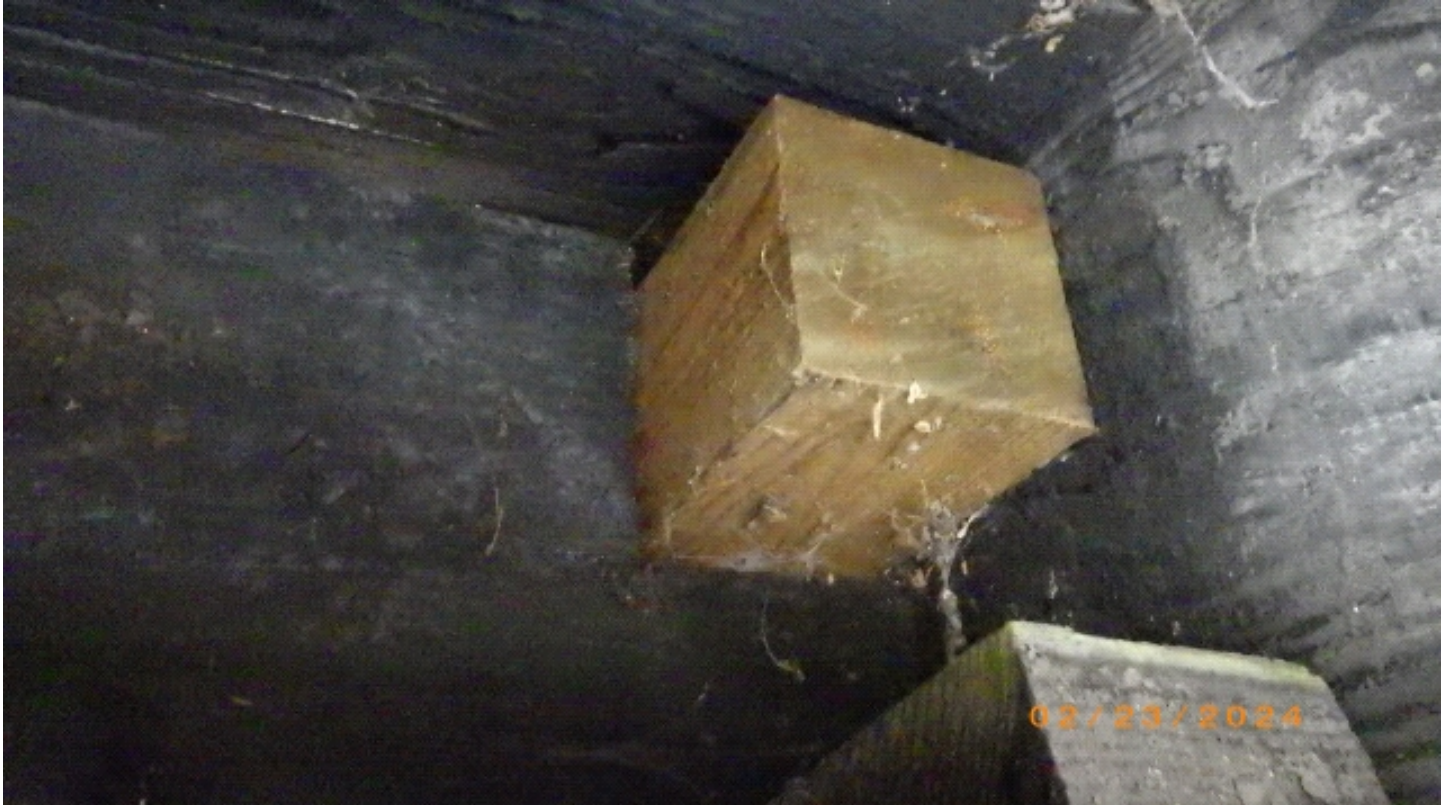
Approach span sitting on backing boards.
