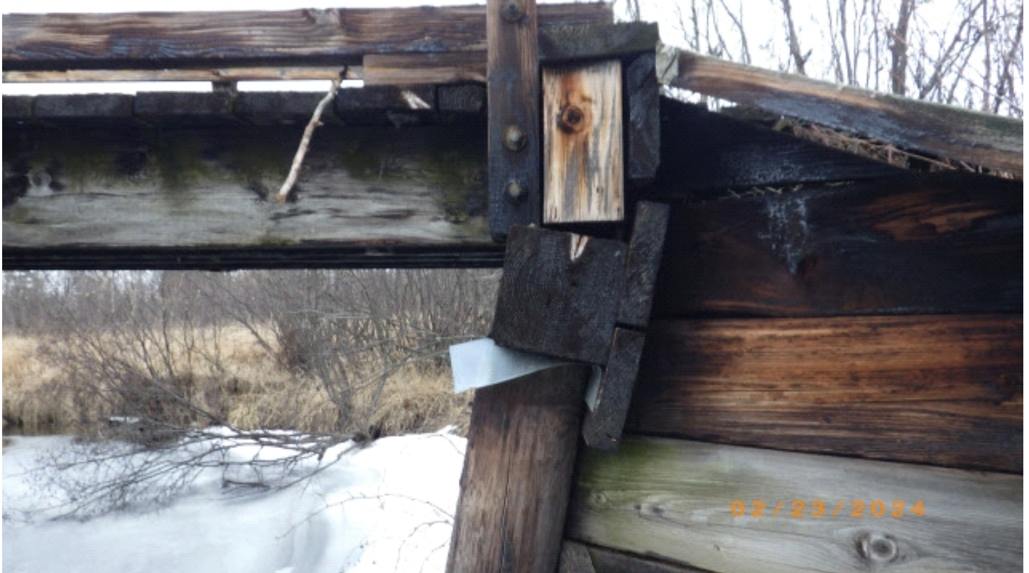
Rotating pile cap.
