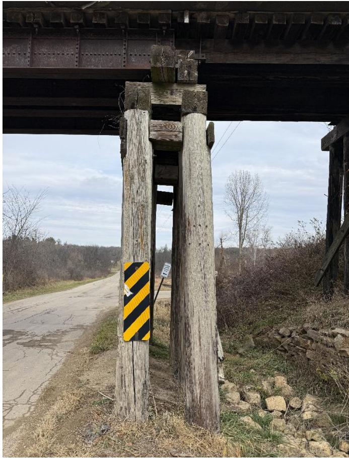
Photo 29 – Pier W4 Looking North.
