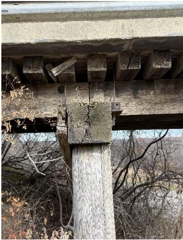
Photo 21 – Pier W1 Cap Looking North.
