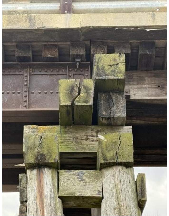
Photo 30 – Pier W3 Looking South.
