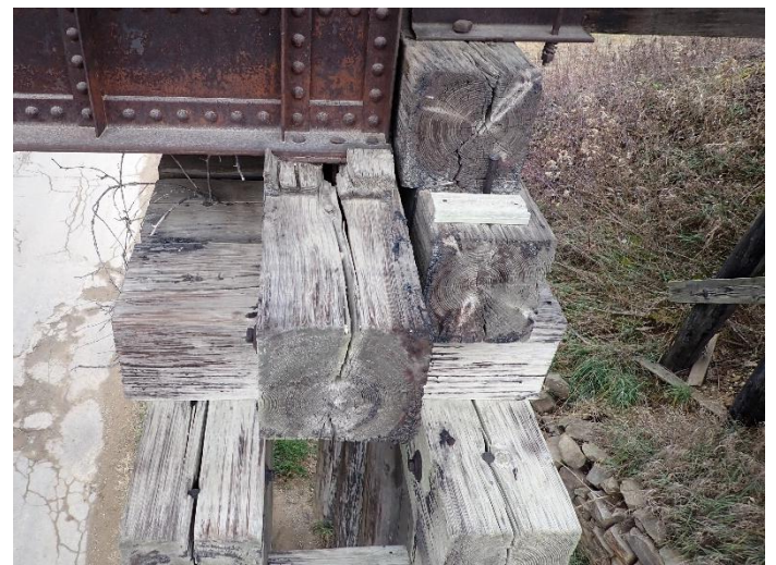
Photo 46 – Pier W4-South End.
