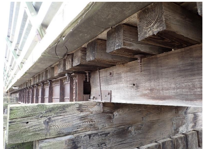
Photo 48 – Span W5-South Beam Looking East.
