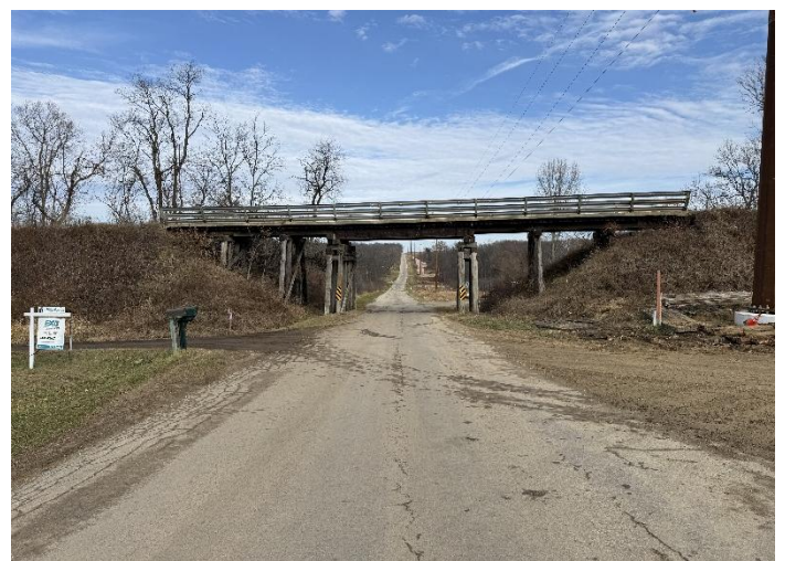
Photo 6 – Side View Looking North.
