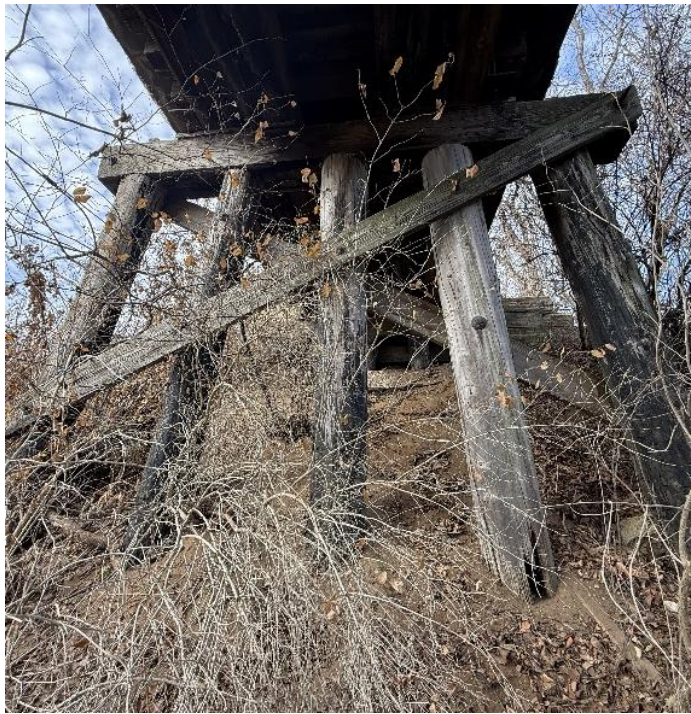
Photo 9 – Pier W1 Looking West.
