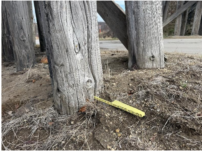
Photo 25 – Pier W3-E. Row-Pile S5.
