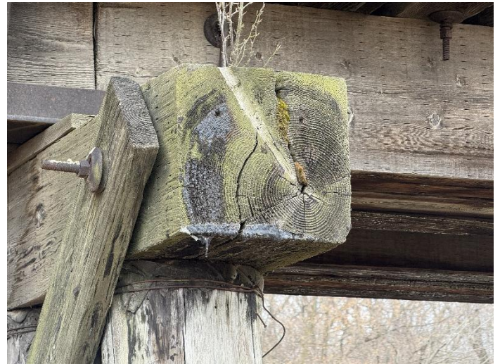
Photo 32 – Pier W5 Looking South.
