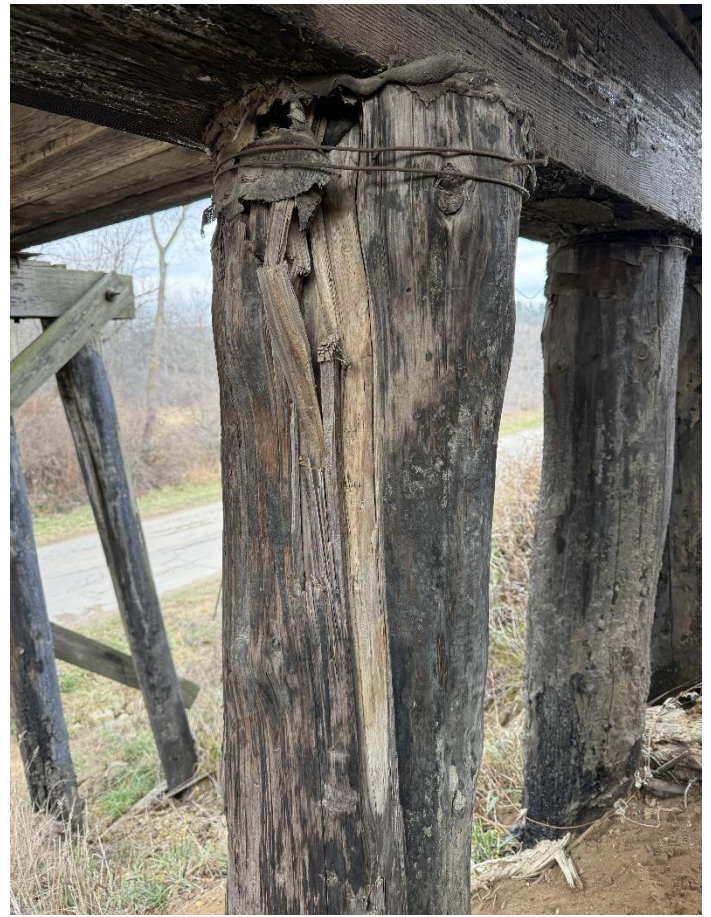
Photo 34 – Pier W6-Pile S3.
