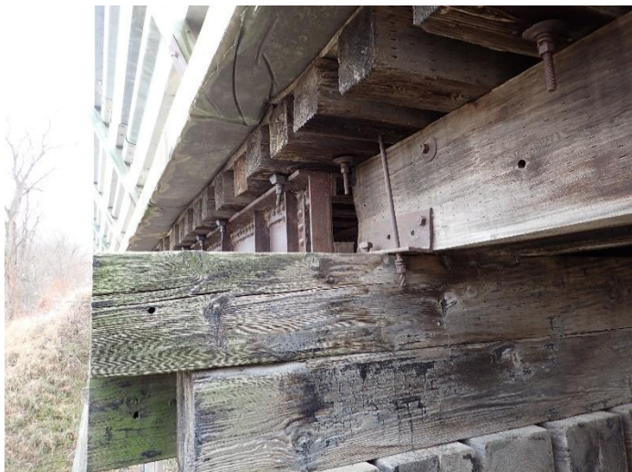
Photo 41 – Span W3-South Beam Looking East.
