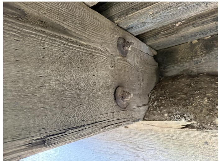
Photo 18 – Span W1-S. Beam-N. Face Over W. Abut.
