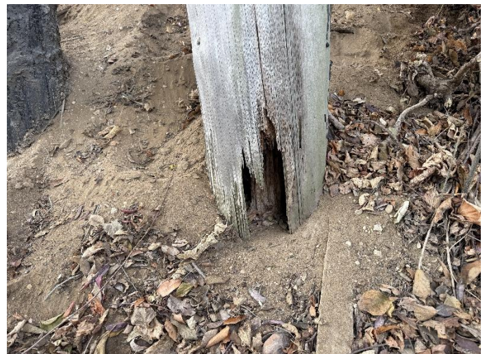
Photo 20 – Pier W1-Pile S4.
