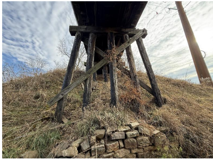
Photo 15 – Pier W5 Looking East.
