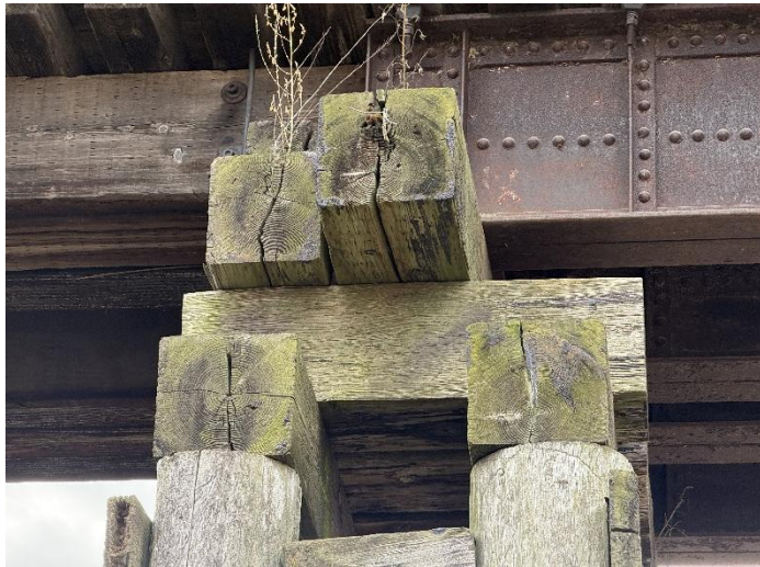
Photo 31 – Pier W4 Looking South.
