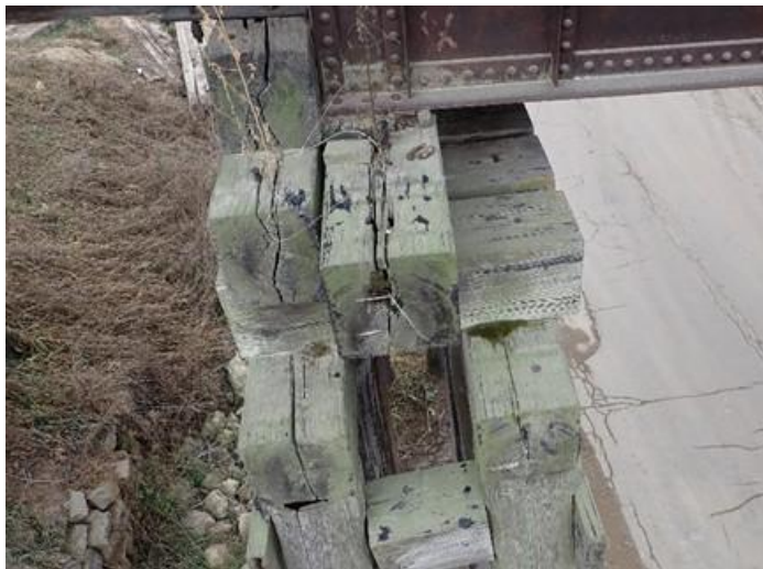
Photo 39 – Pier W4 Looking South.
