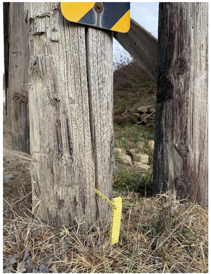
Photo 28 – Pier W4-E. Row-Pile S1.
