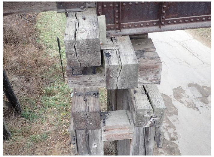
Photo 44 – Pier W3 Looking North.
