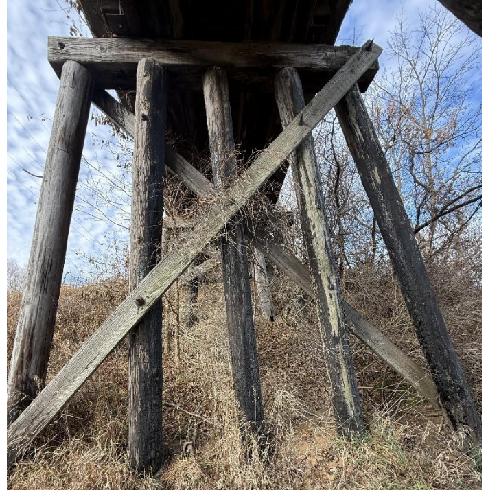
Photo 10 – Pier W2 Looking West.
