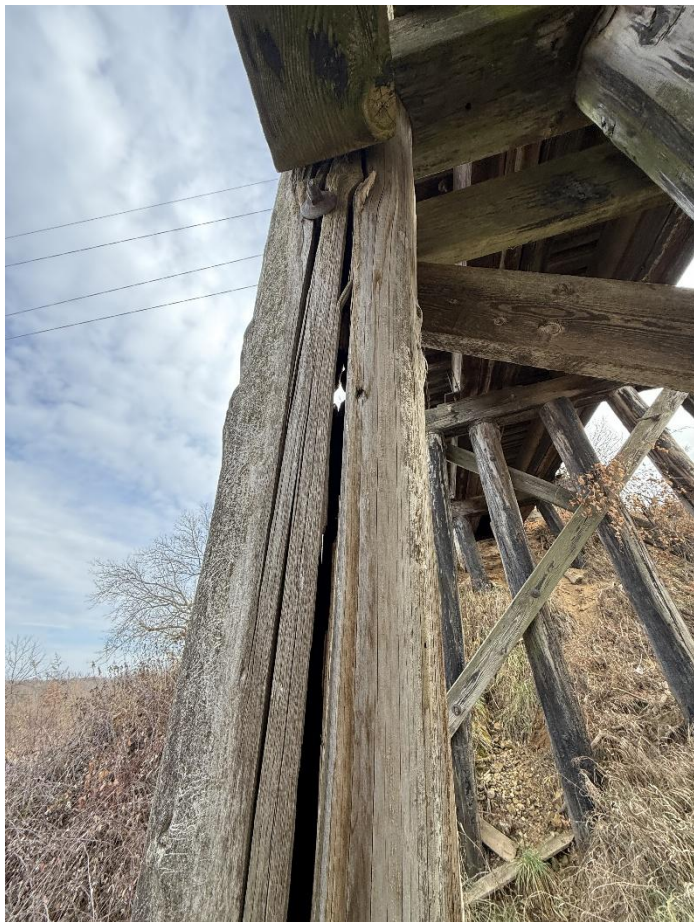
Photo 27 – Pier W4-E. Row-Pile S5.
