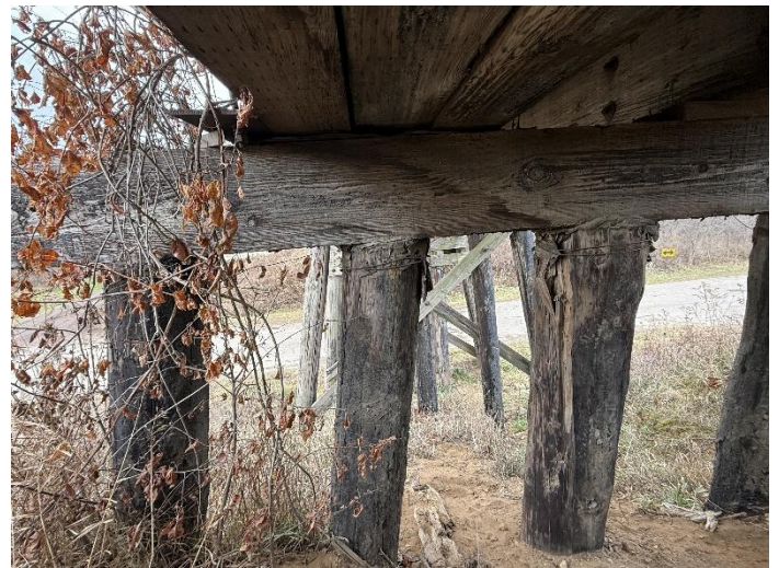
Photo 36 – Pier W6-Piles S1-S3 Looking West.
