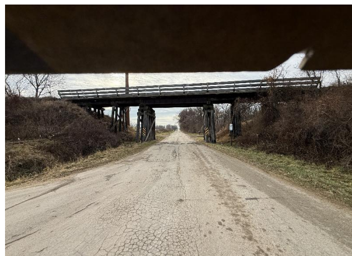
Photo 5 – Side View Looking South.
