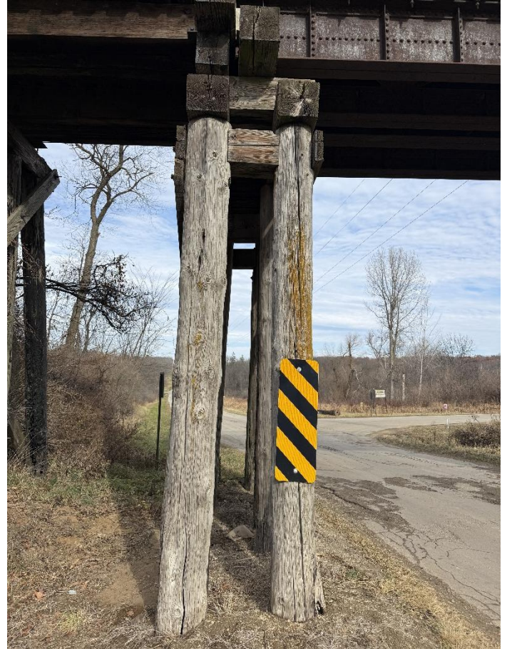
Photo 22 – Pier W3 Looking North.
