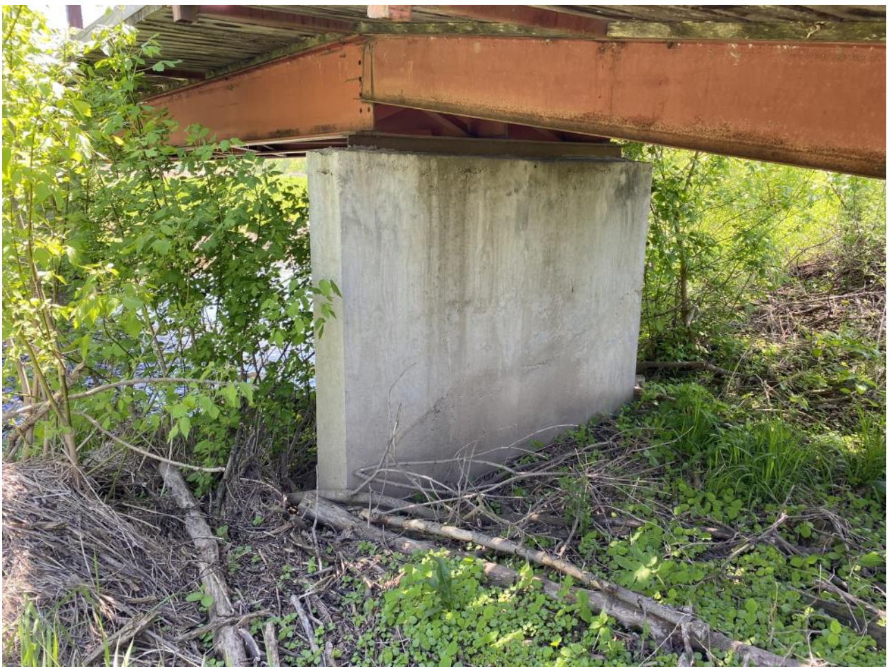
Set high on narrow concrete abutments. Rip rap missing so bridge has little protection
