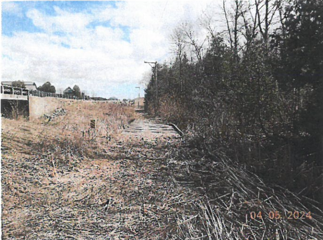
West Approach Looking East
