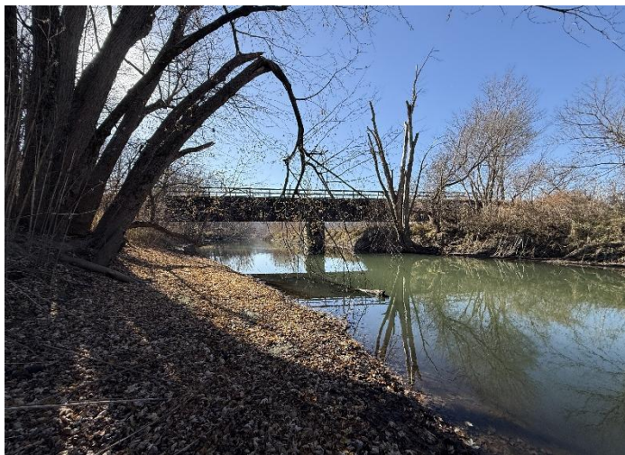
Photo 5 – Side View Looking South.
