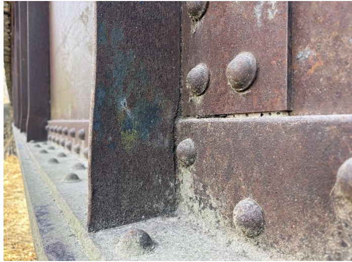
Photo 19 – West Span-North Beam.
