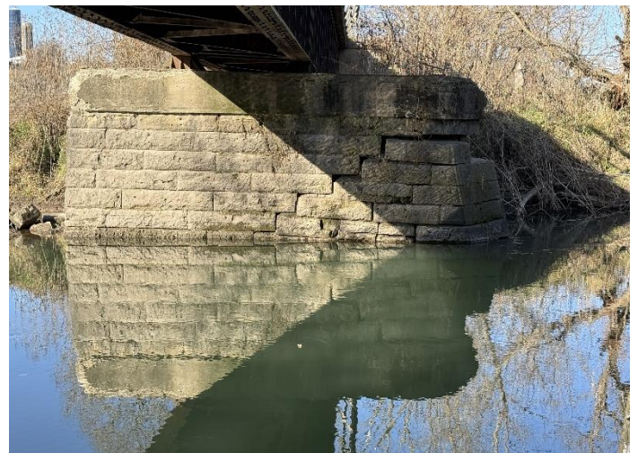
Photo 6 – Pier Looking West.
