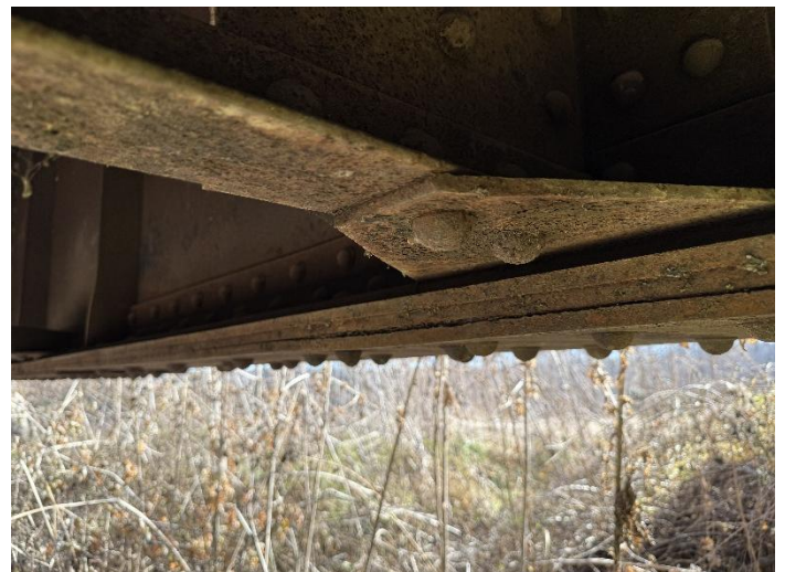
Photo 18 – West Span-South Beam.
