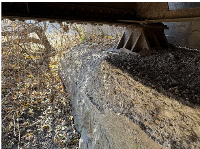
Photo 17 – West Abutment-South Bearing.
