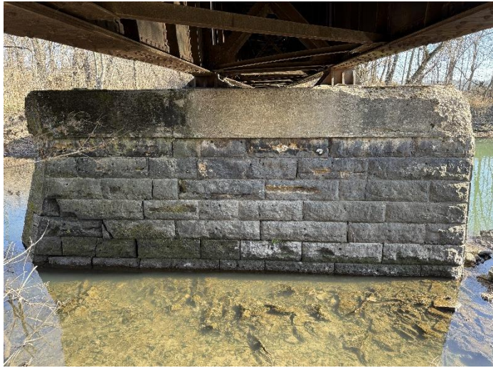
Photo 13 – Pier Looking East.
