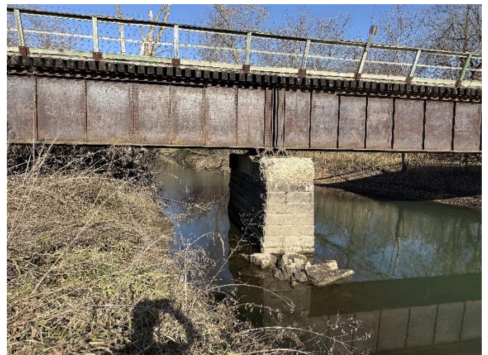
Photo 12 – Pier Looking North.
