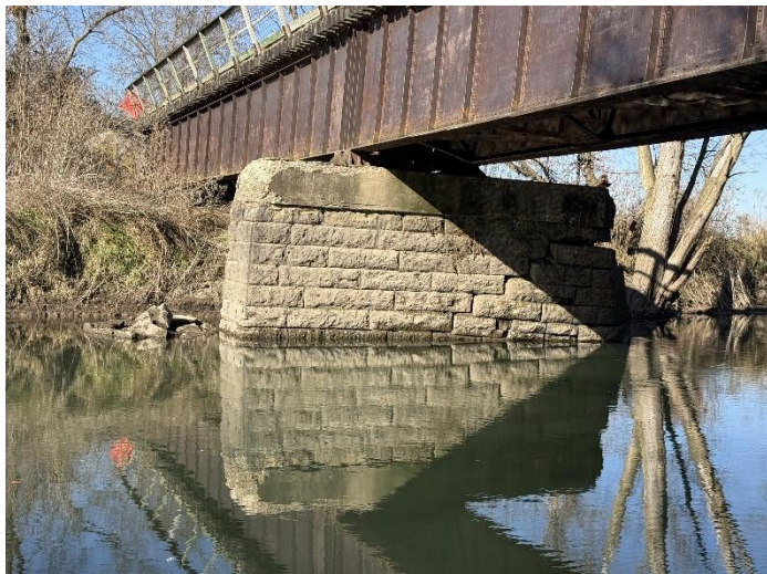
Photo 9 – Pier Looking West .
