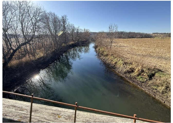
Photo 4 – Downstream Looking South.
