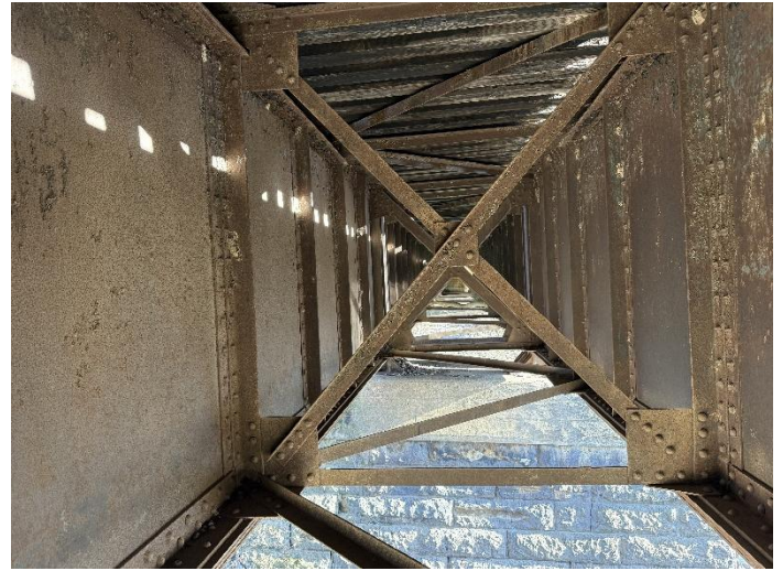
Photo 20 – West Span Looking East.
