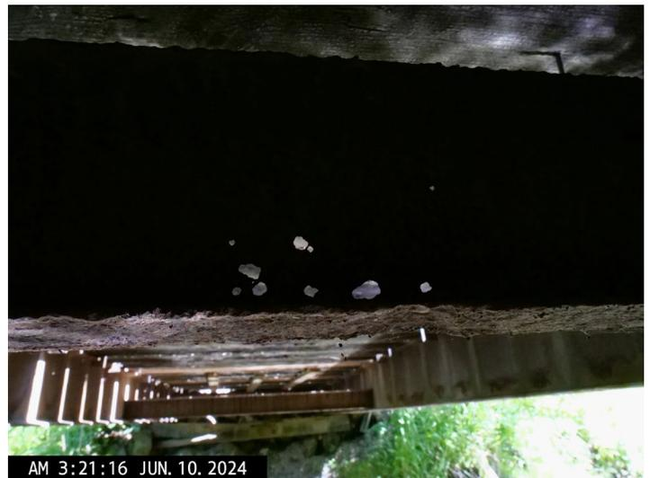
North I Beam Diaphragm with metal section loss & Holes
