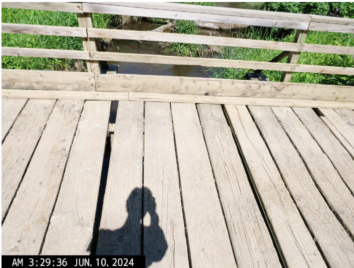
Timber Plank Gaps Looking Upstream to East
