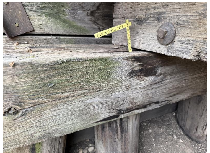
Photo 36 – East Abutment-North End.
