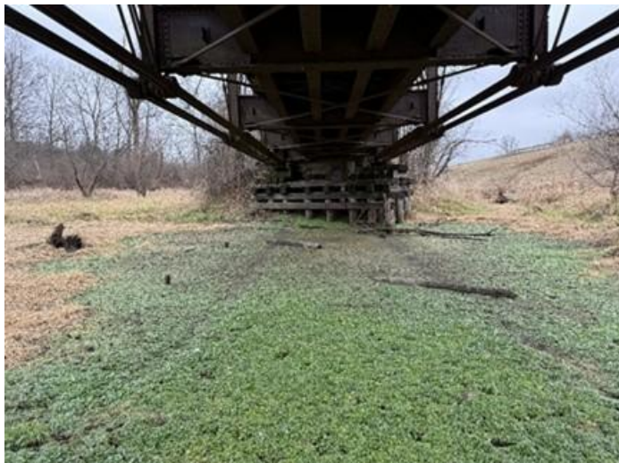
Photo 33 – Pier W4 Looking East.
