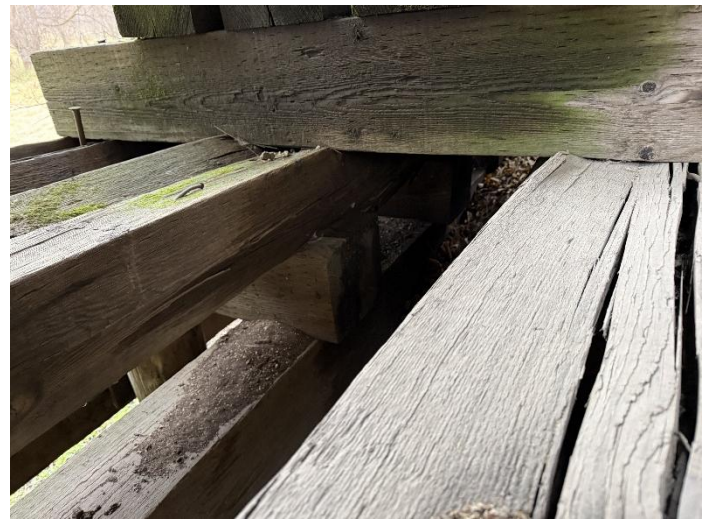
Photo 10 – Pier W4 Looking North-Cribbing.
