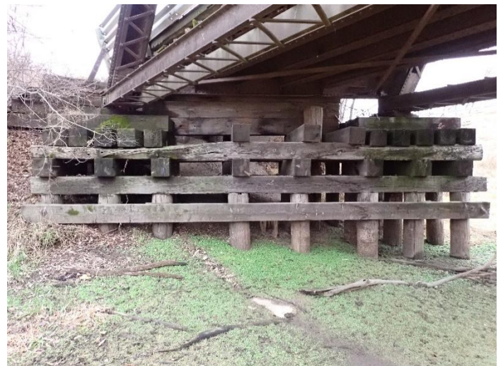
Photo 18 – Pier W4 Looking West.
