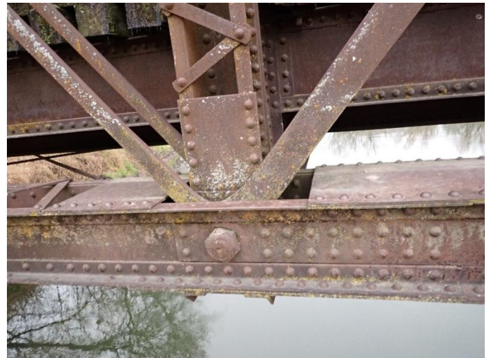
Photo 44 – Span W1-South Truss L3.
