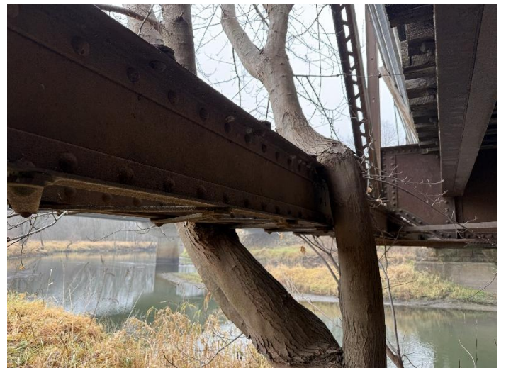
Photo 40 – Span W2-South Truss L4-L5.
