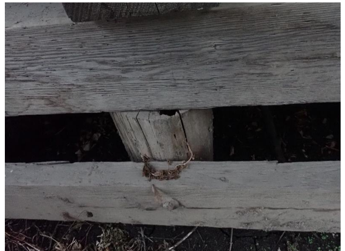
Photo 28 – Pier W3 Looking West.
