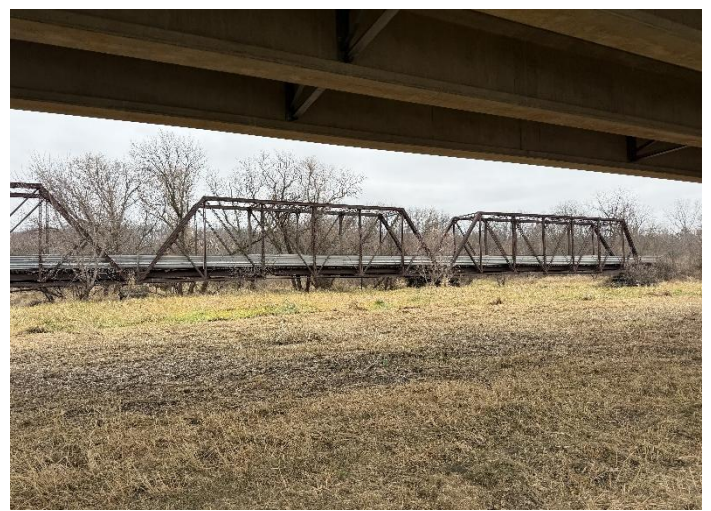
Photo 6 – Side View Looking North-East Spans.
