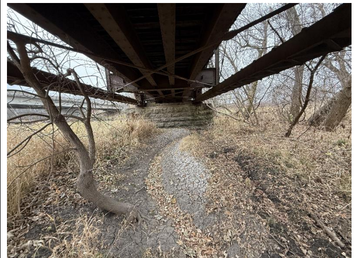
Photo 24 – Pier W2 Looking West.
