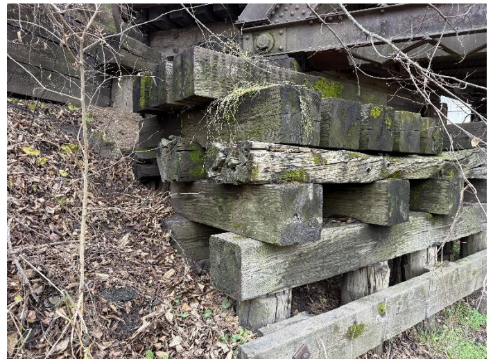
Photo 16 – Pier W4 Looking West-North Bearing.
