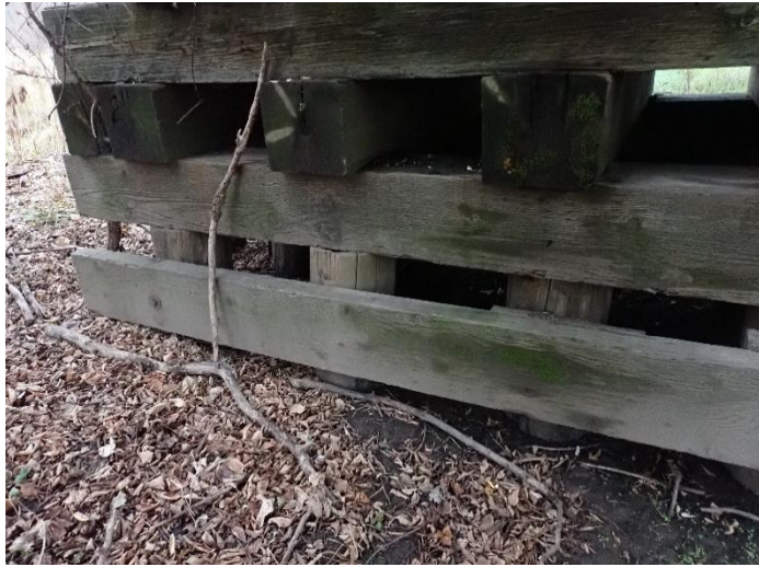
Photo 31 – Pier W3 Looking East.
