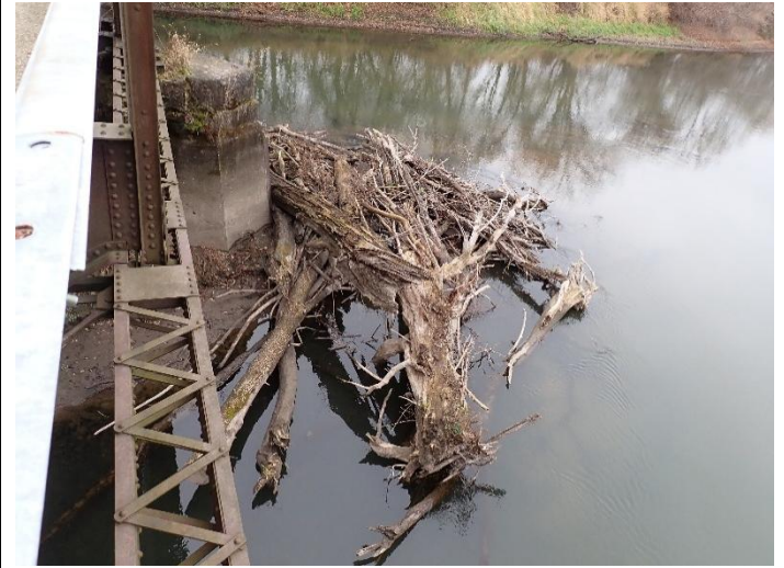
Photo 20 – Pier W1 – Upstream (North) End.
