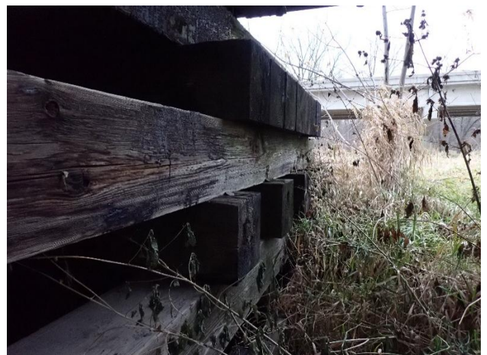
Photo 30 – Pier W3 Looking South.
