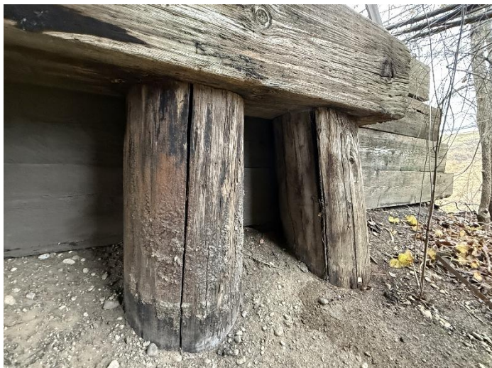
Photo 35 – East Abutment-Piles S2-S1.
