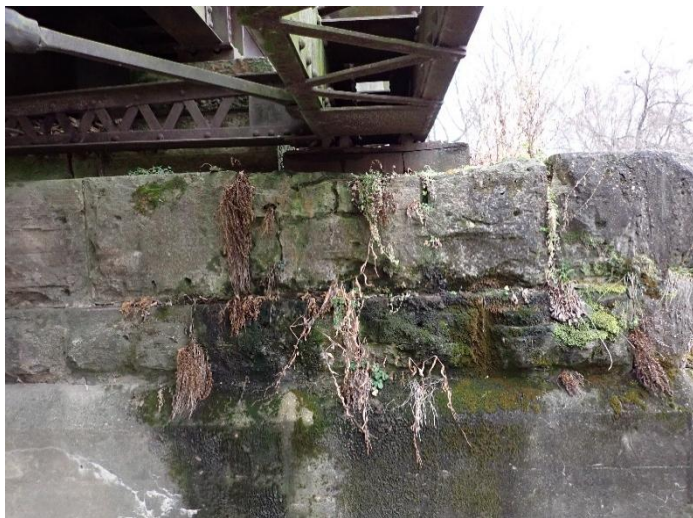
Photo 41 – Pier W1 Looking West.
