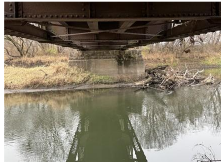
Photo 22 – Pier W1 Looking West.
