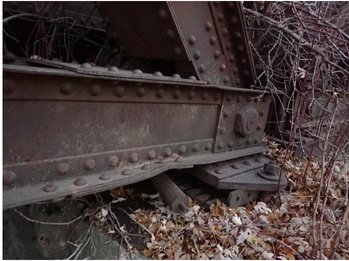
Photo 37 – Span W2-SE. Bearing Over Pier W2.
