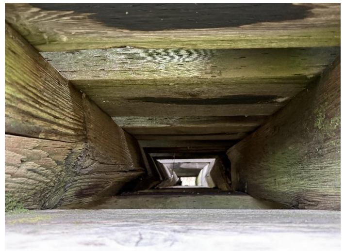
Photo 12 – Pier W4 Looking North-Cribbing.
