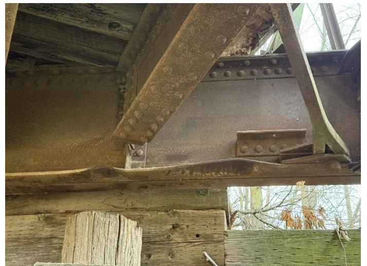
Photo 42 – Span W4-Floor Beam 7 (East).
