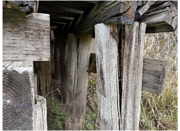
Photo 8 – Pier W4 Looking North.
