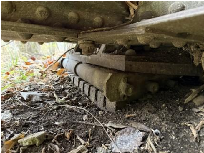
Photo 39 – Span W1-S. Bearing Over W. Abutment.
