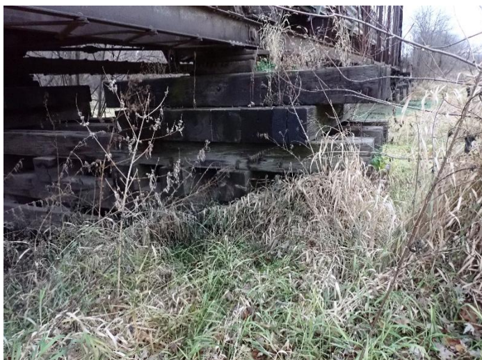
Photo 29 – Pier W3 Looking East.
