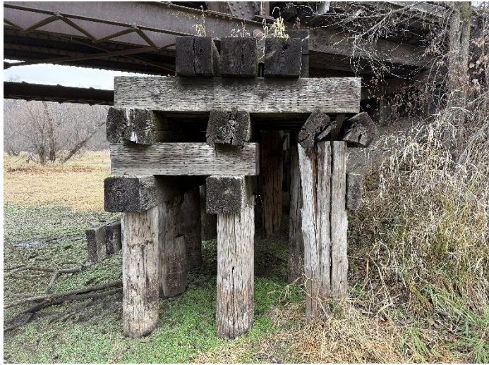
Photo 7 – Pier W4 Looking North.
