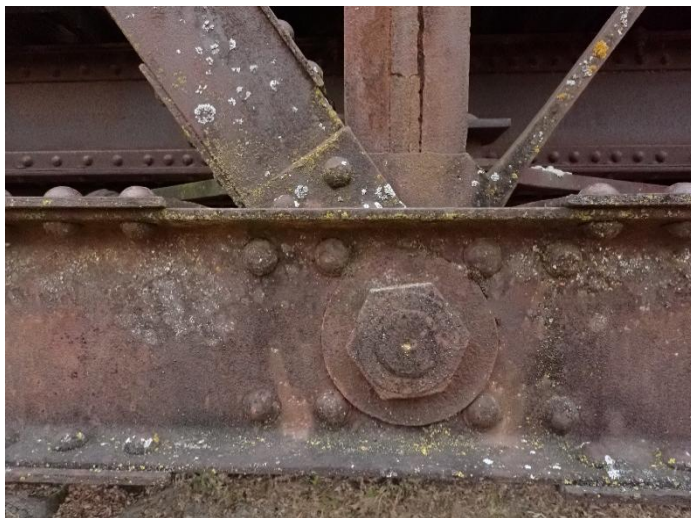
Photo 47 – Span W3-South Truss L1.
