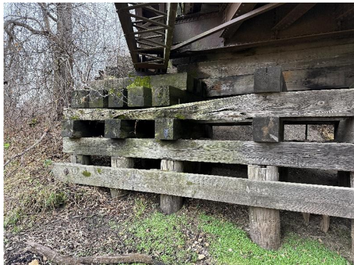
Photo 15 – Pier W4 Looking West-North Bearing.
