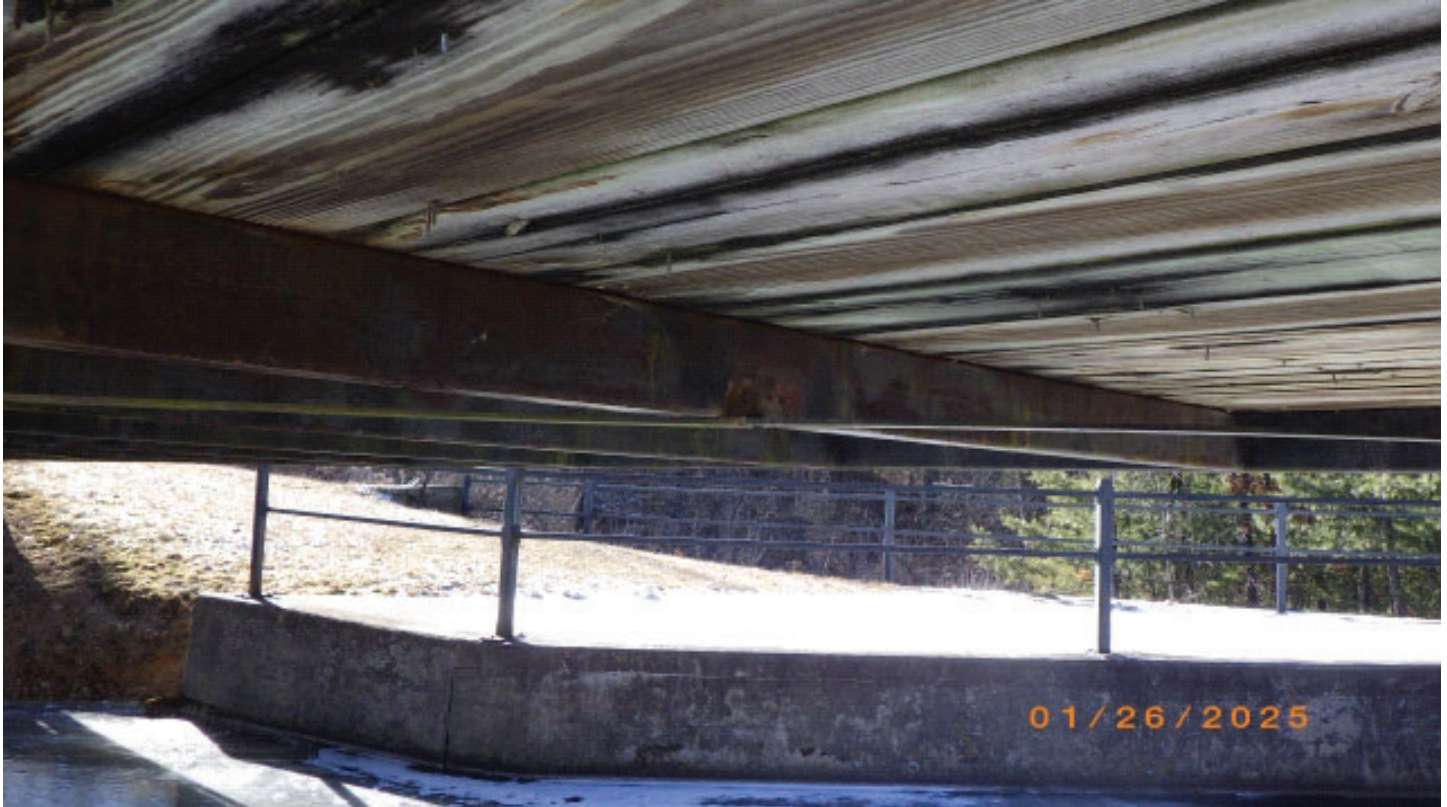
Corrosion in diagonals and floor beams.
