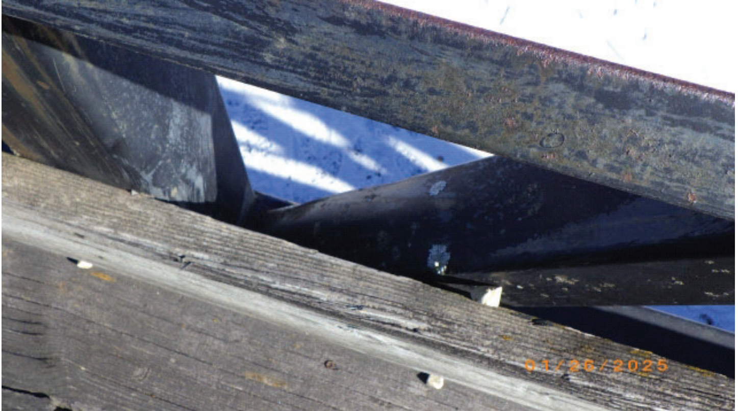
9th diagonal from South, East Truss, bulged at bottom chord. Most likely moisture.
