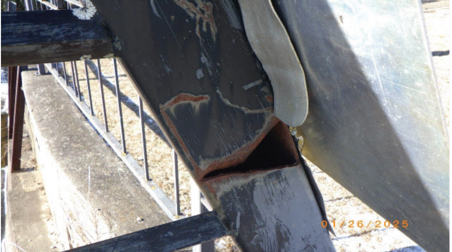
Large gouge NE Diagonal
