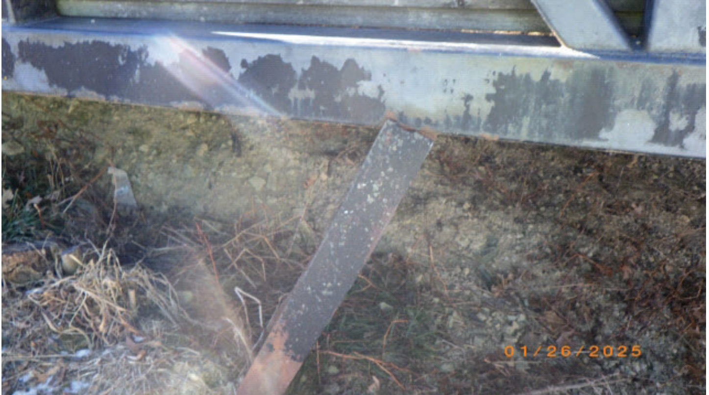
Odd brace, SE corner, dent in bottom chords.
