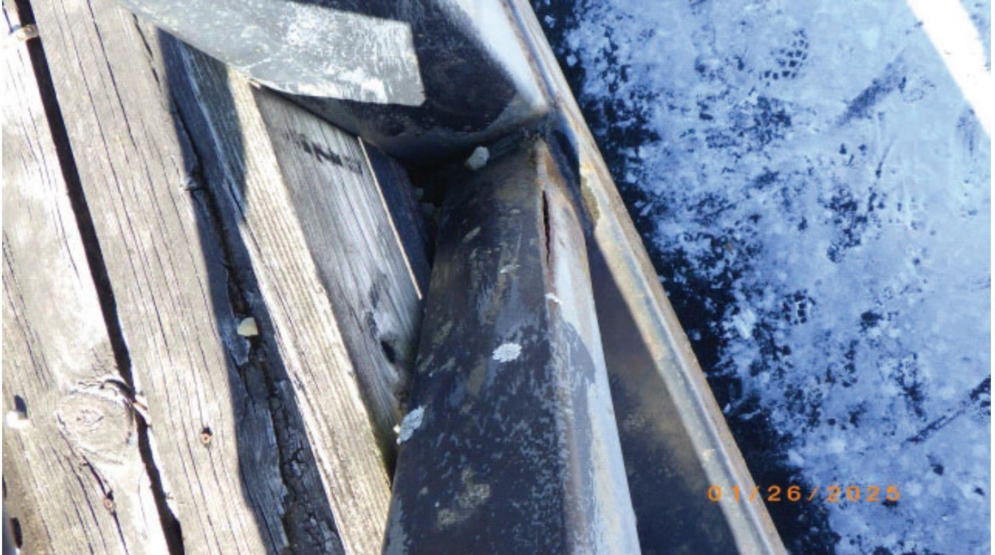
Crack in same 9th diagonal.
