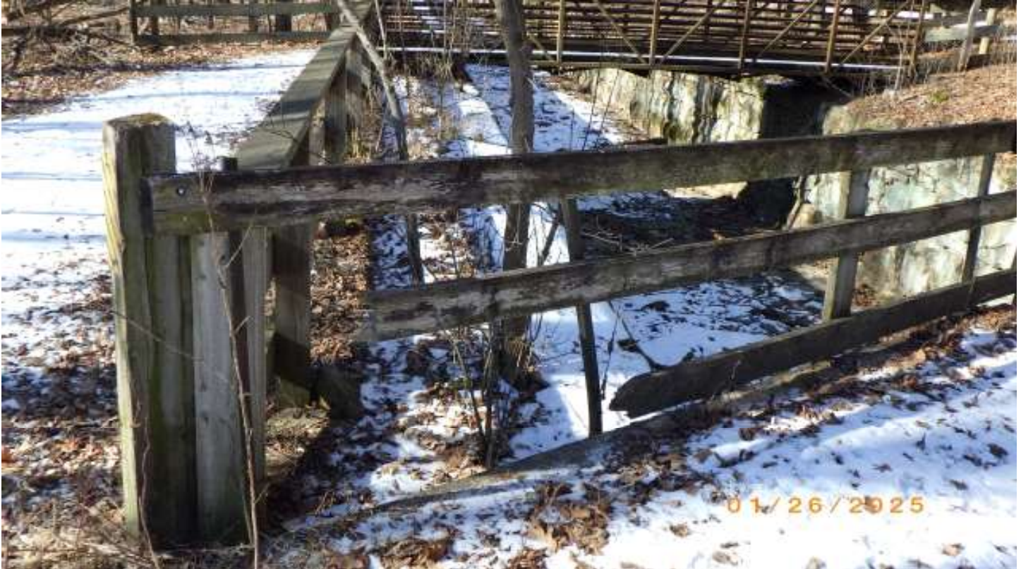
Missing Railing.
