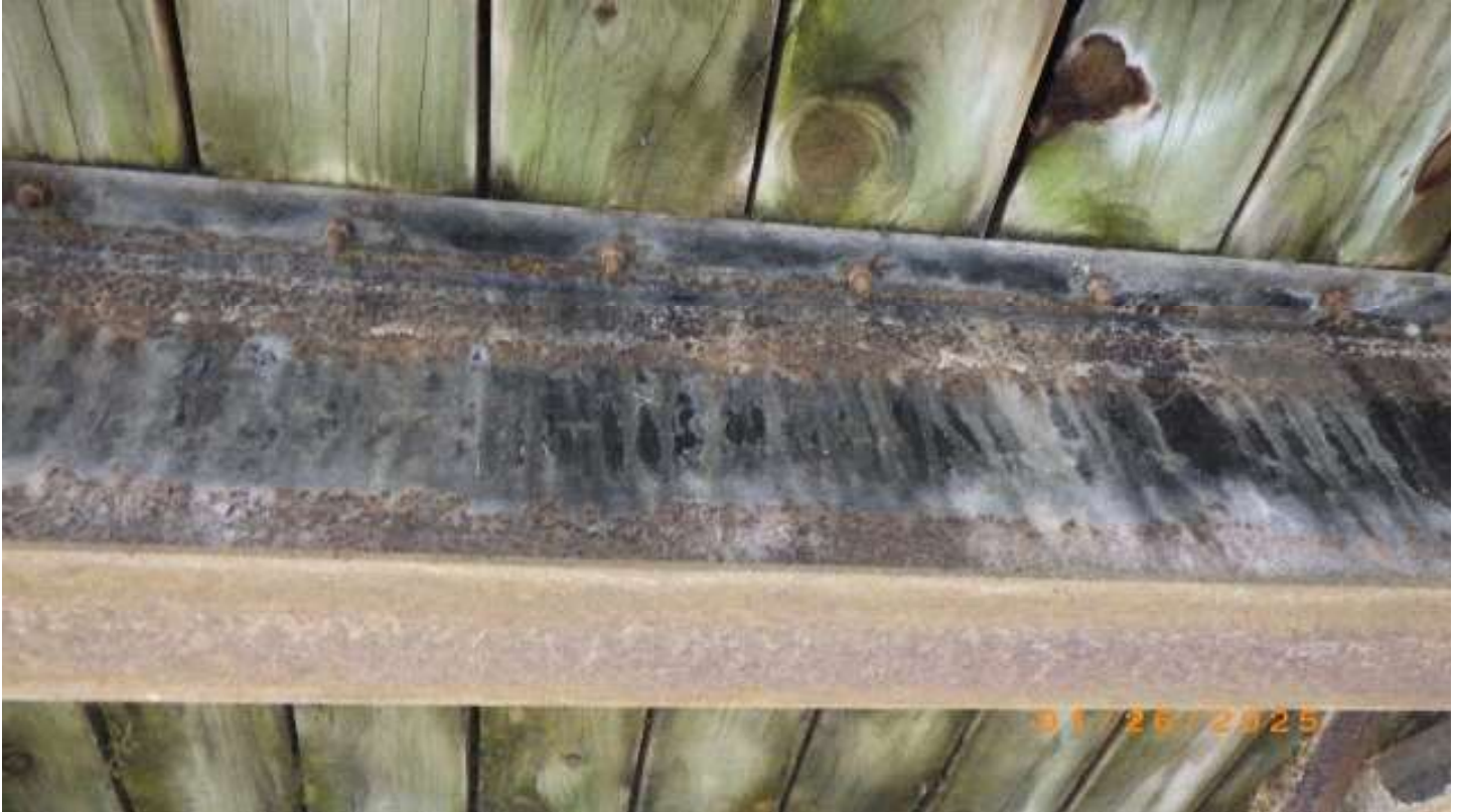
CS3 Corrosion of girders, staining of deck boards.
