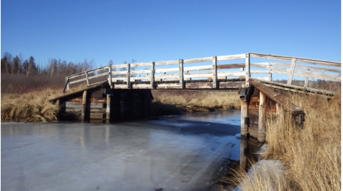
Elevation view from upstream
