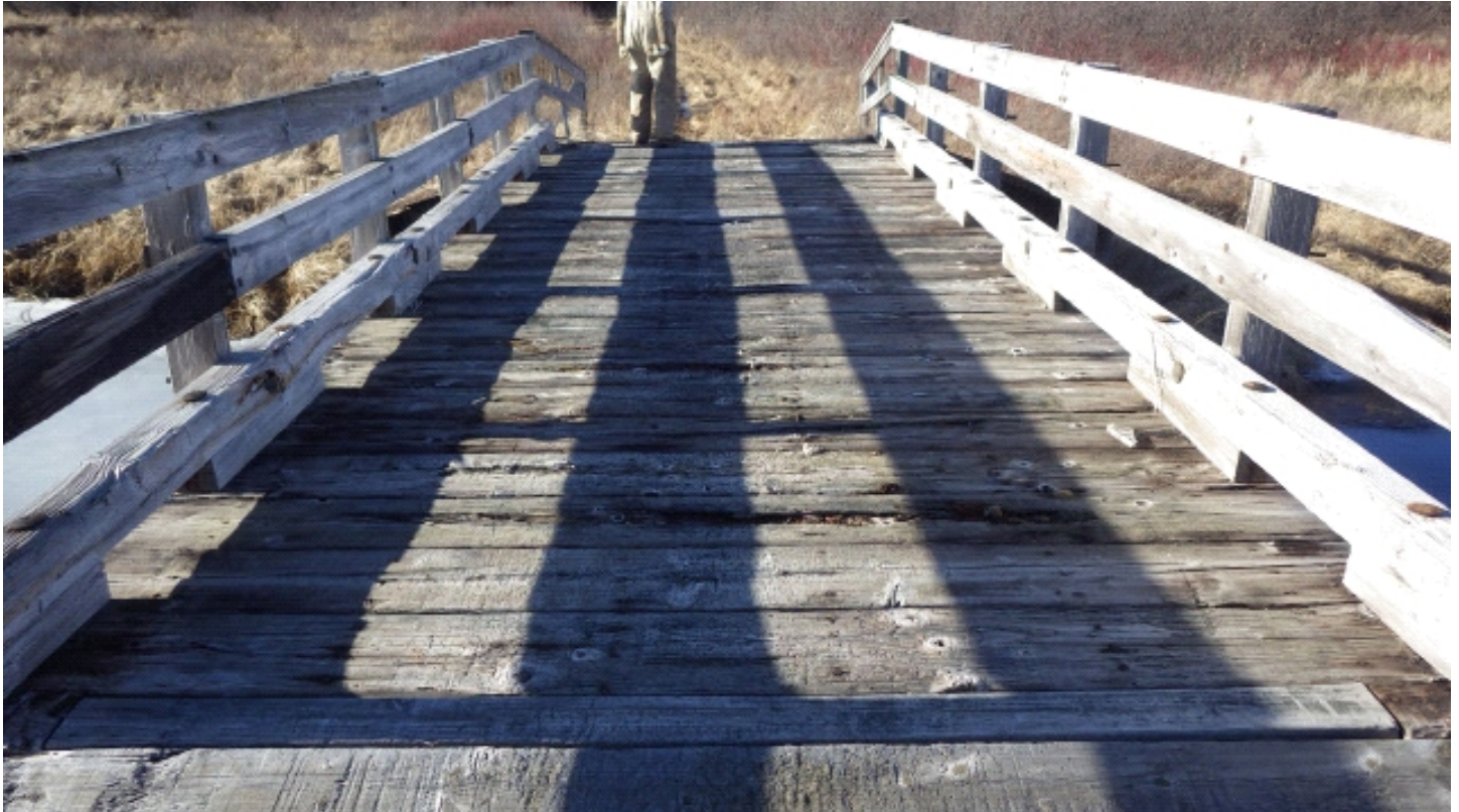
Top of deck and rails
