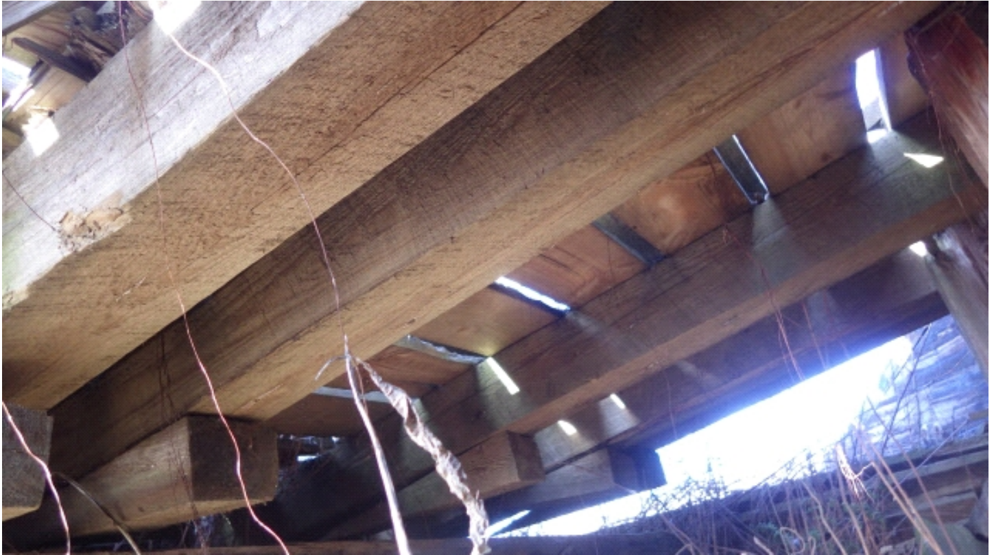
Underside of approach ramps
