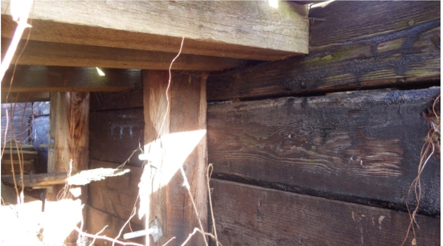
Approach ramp girders bearing on backwall.
