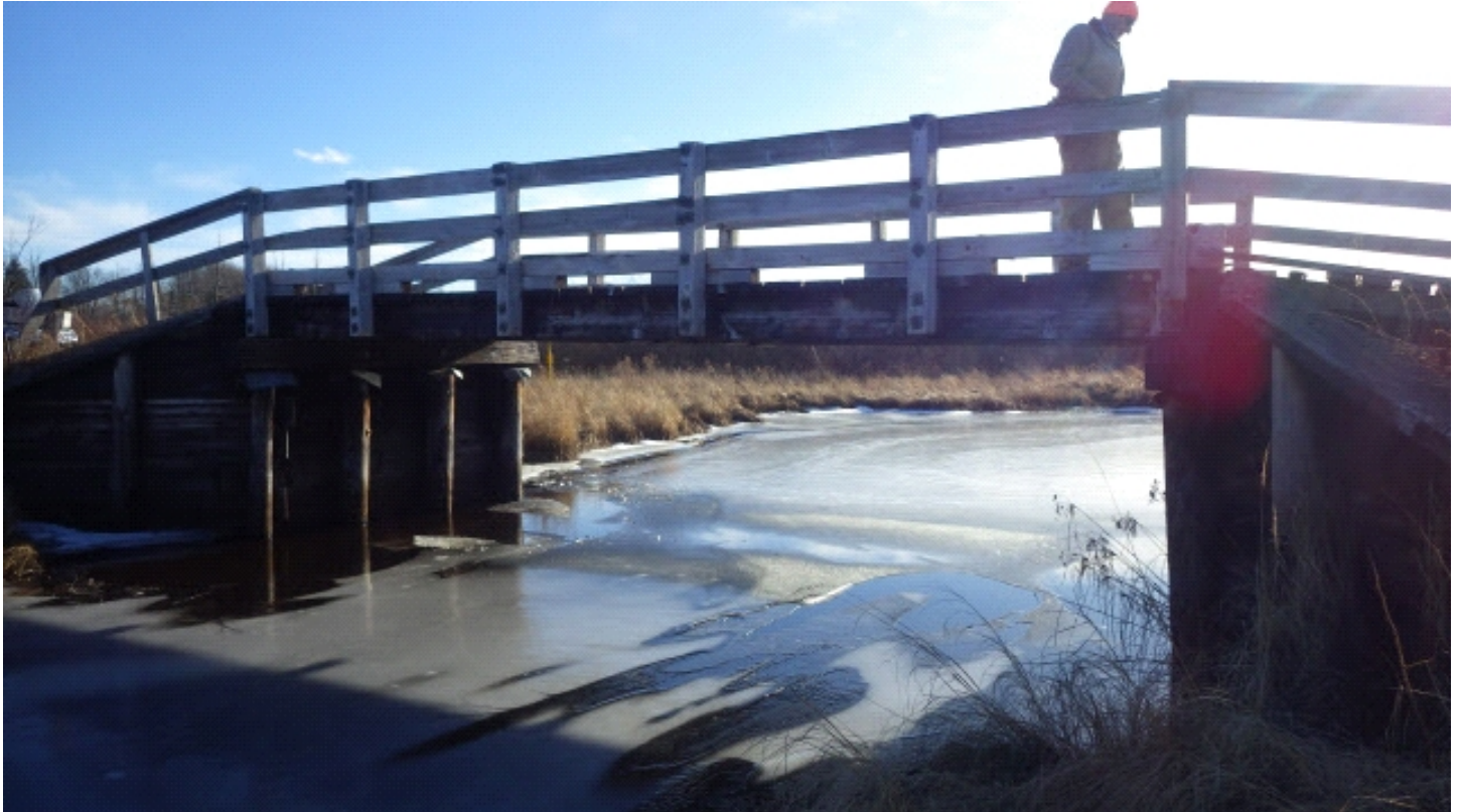
Elevation view from downstream
