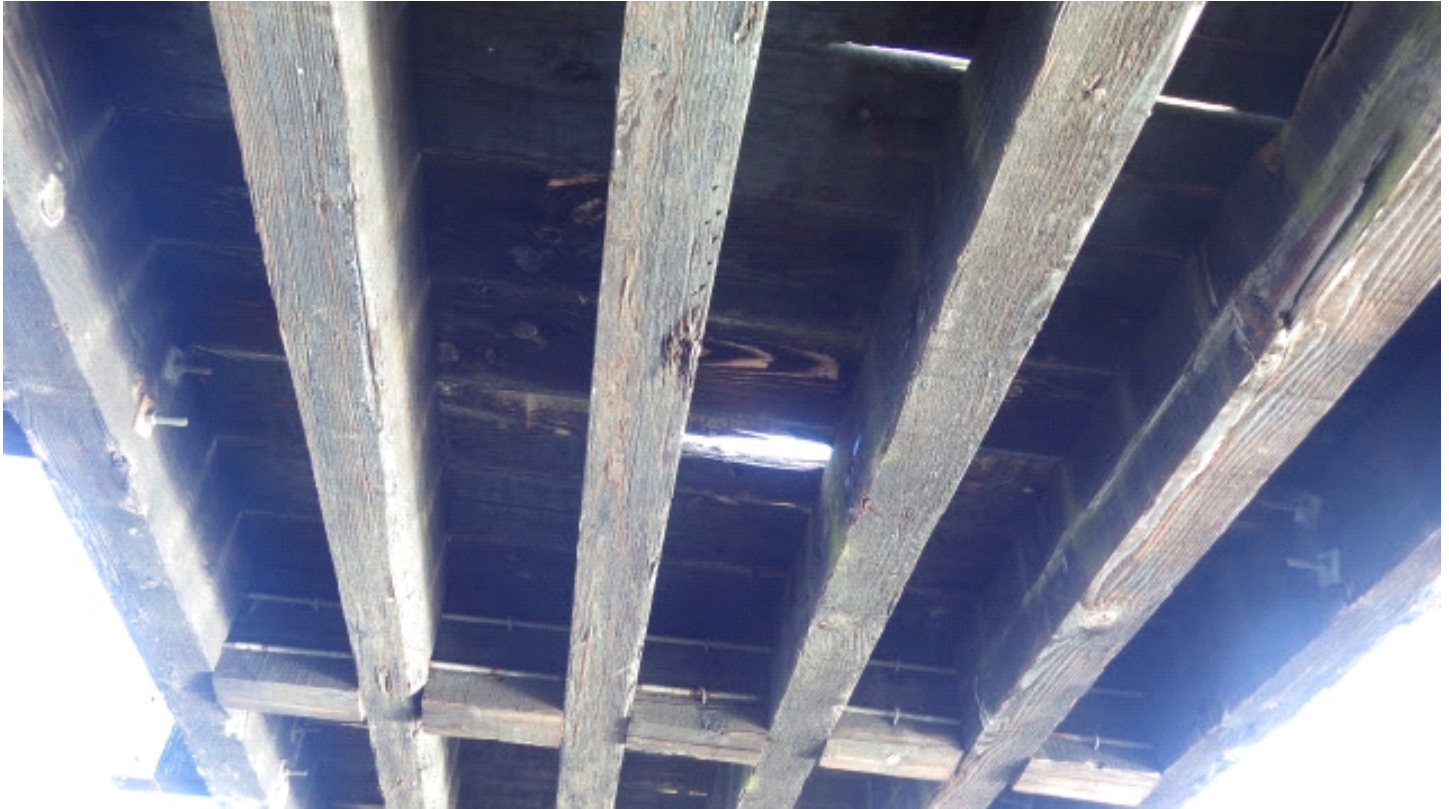
Underside of deck and superstructure
