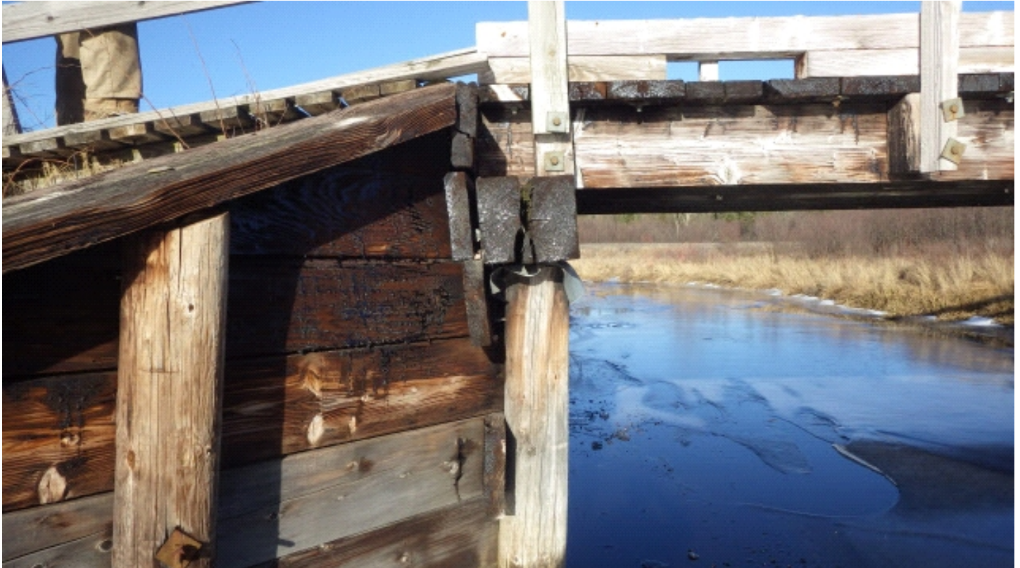
West end of north pile cap
