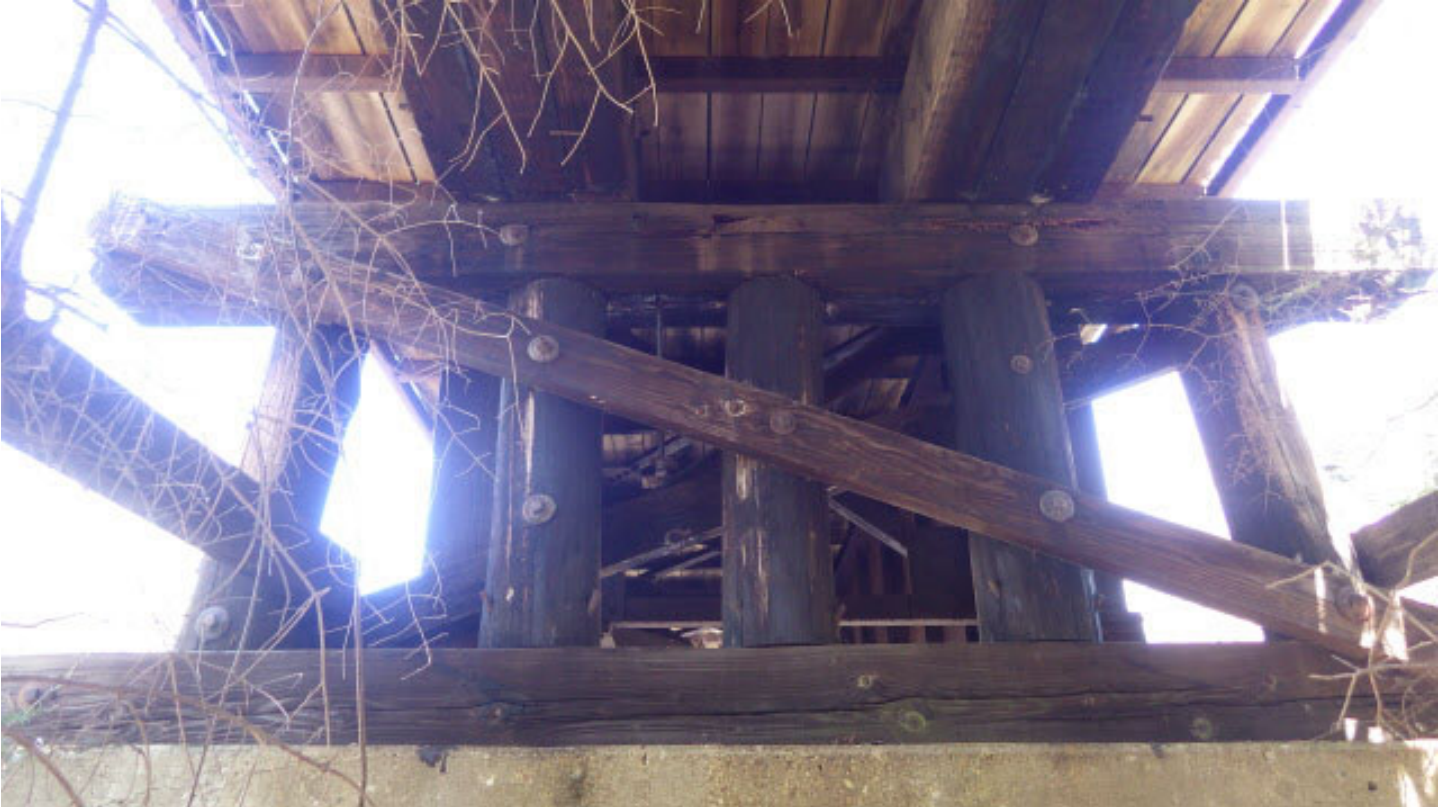
Pier #3, timber cap rotten / crushing
