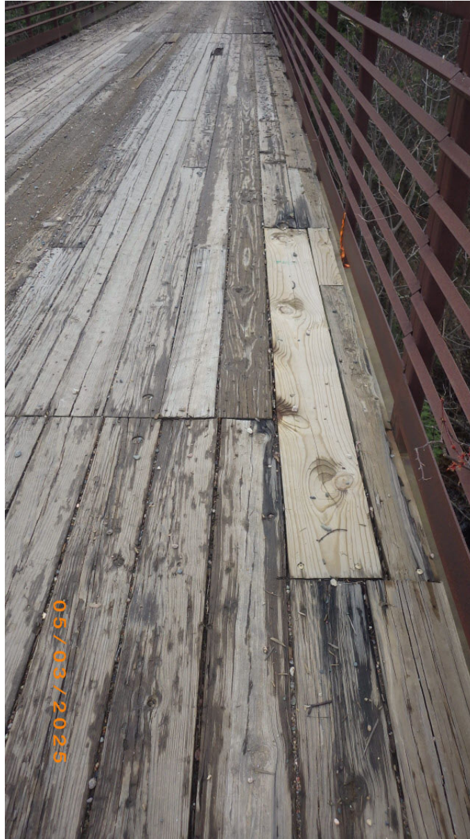
Patched hole at east edge of span 7
