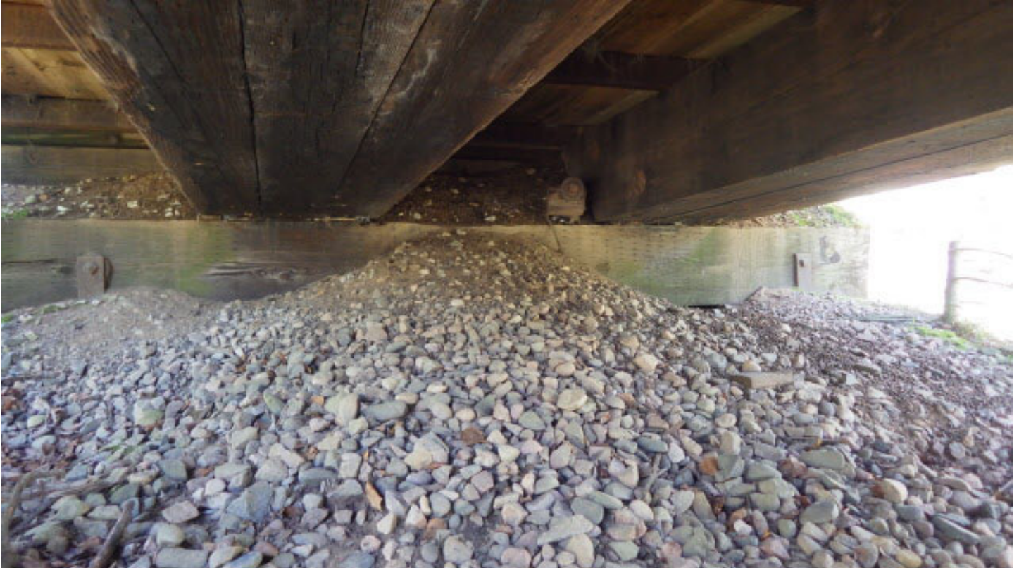
North abutment cap ends rotten
