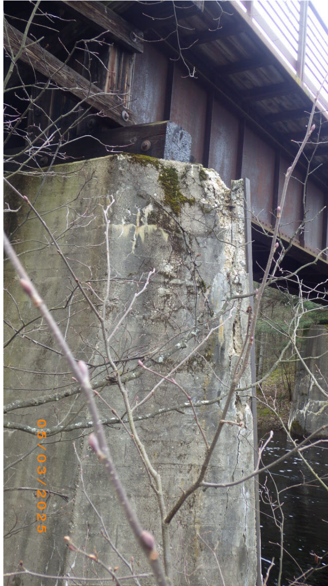
Pier #4 with very large spalls on top corners and CS3 cracking with efflorescence throughout
