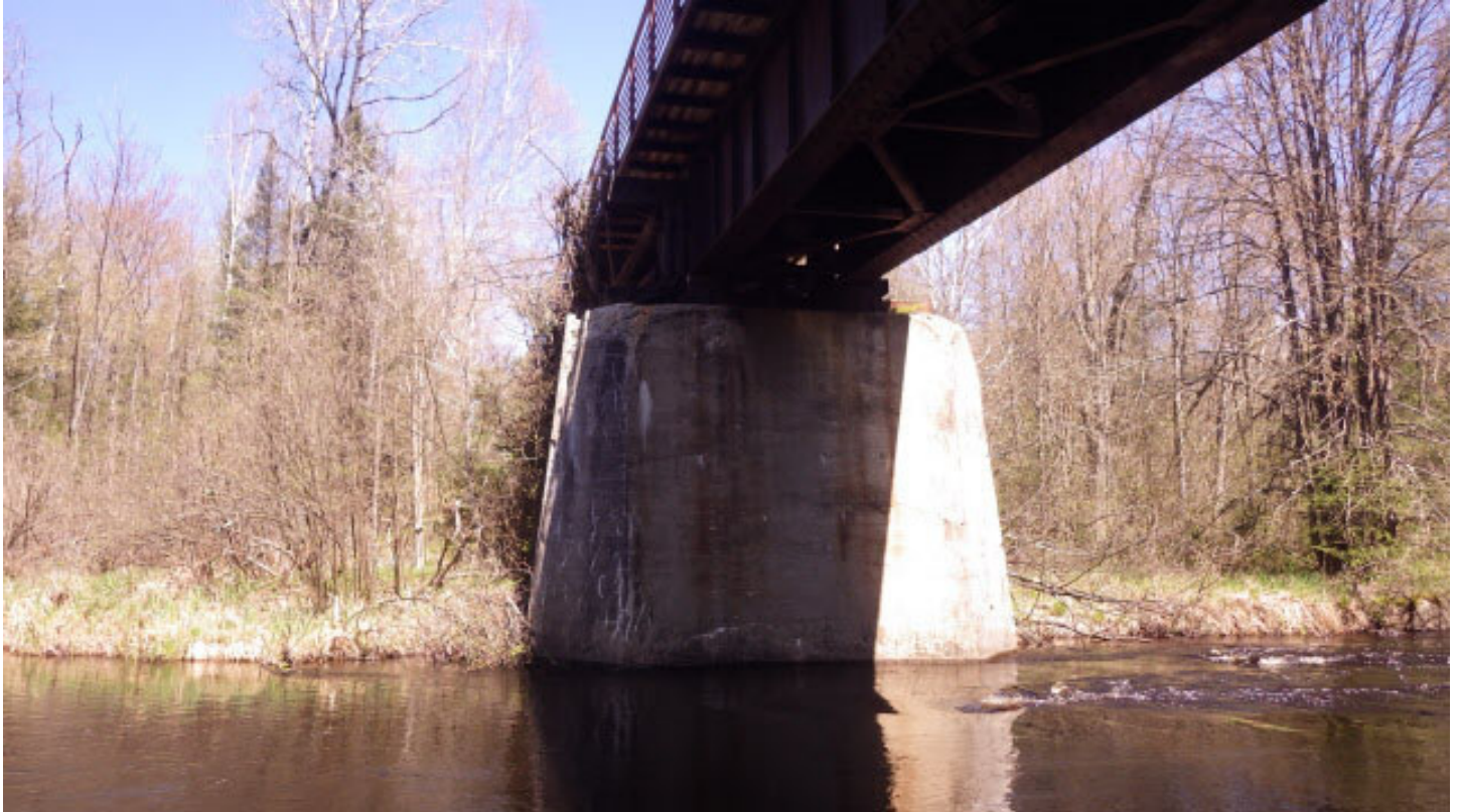
Pier #4 with very large spalls on top corners and CS3 cracking with efflorescence throughout
