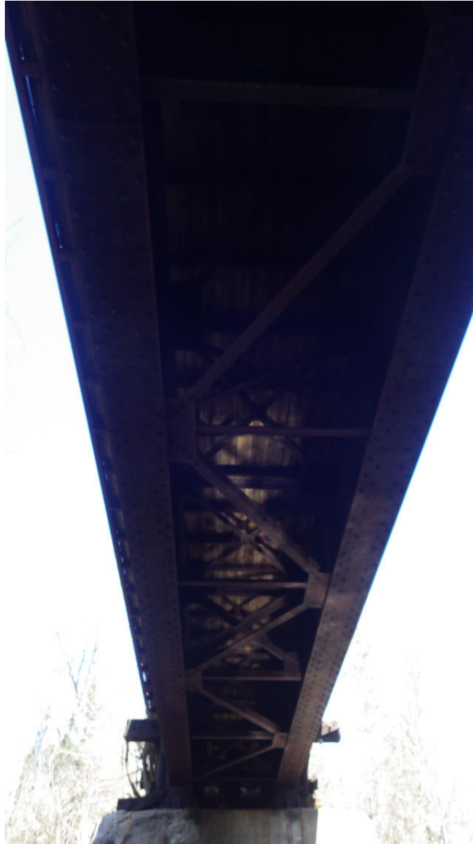
Steel main span in fair condition
