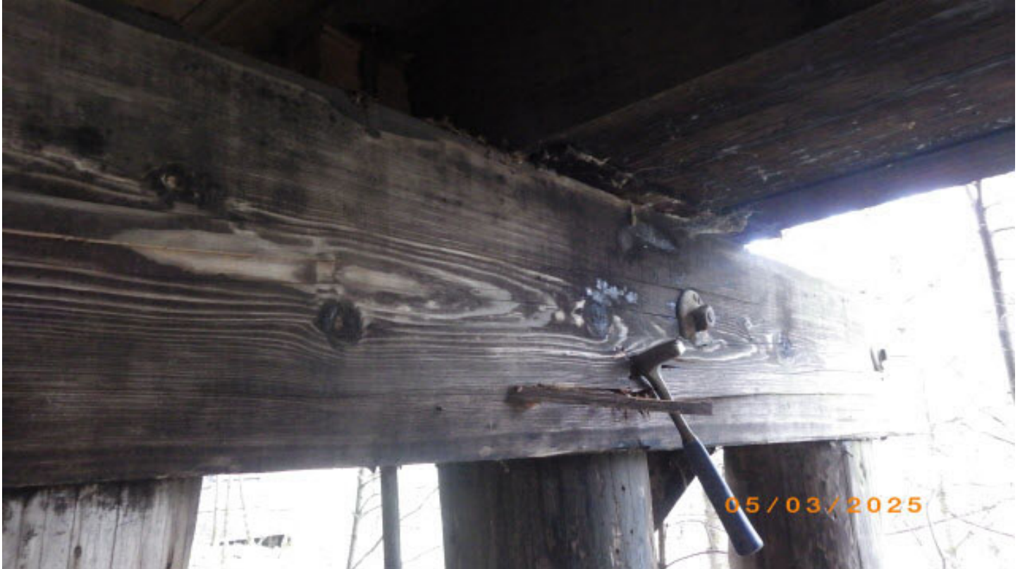
Bent #1, cap rotten / crushing
