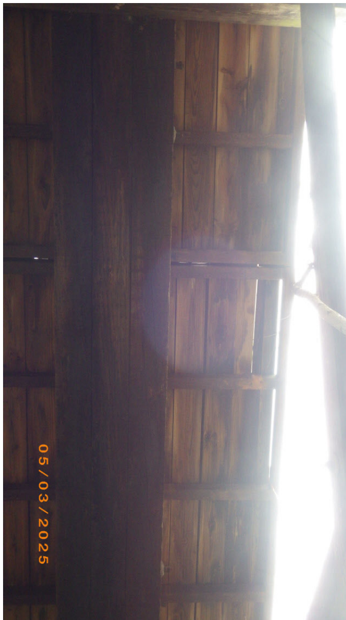
Underside of deck at hole in east edge of span 7. Note other rotten areas.
