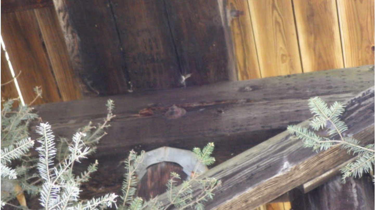
Bent #9 cap is rotten / crushing (close-up)
