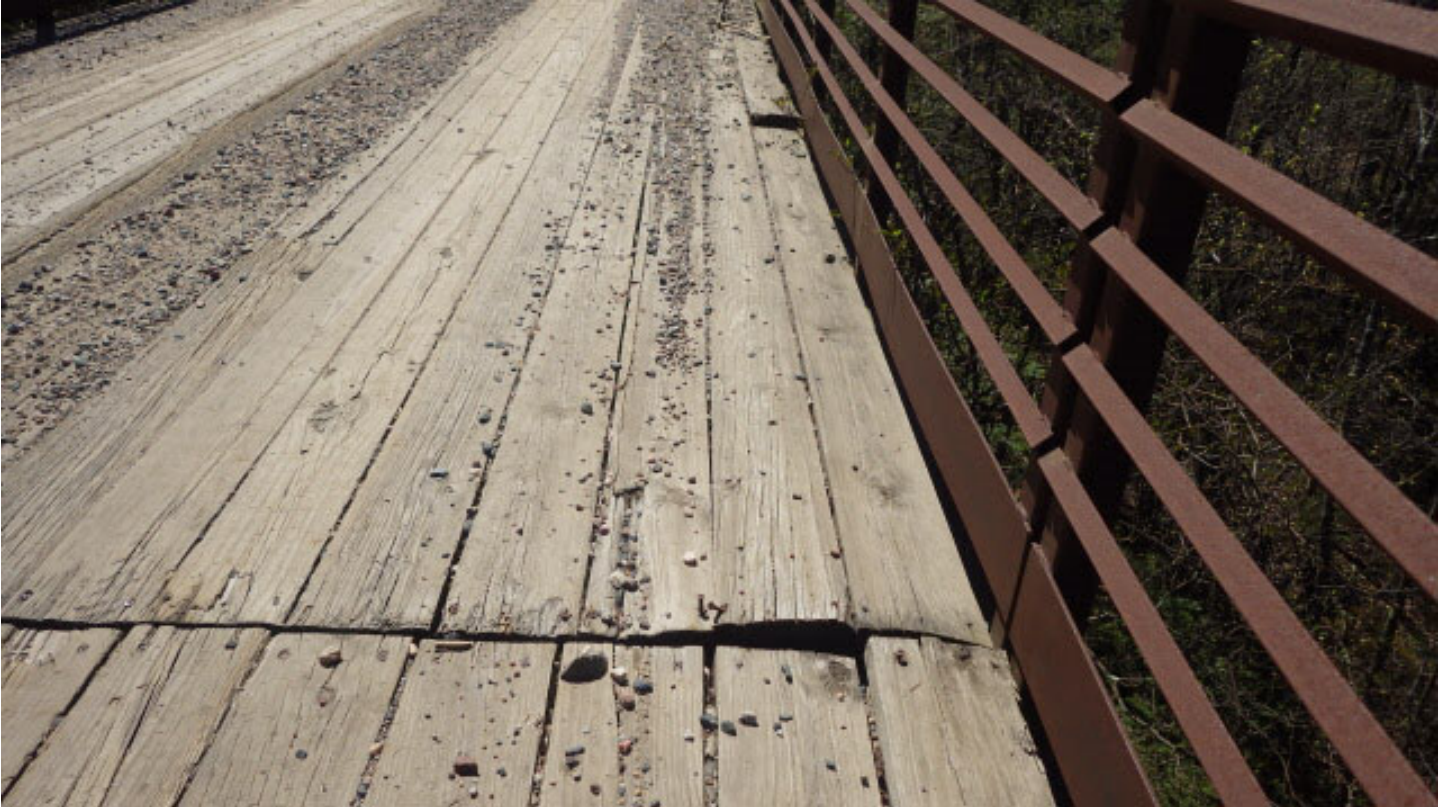
Running planks with ends sticking up 1"+
