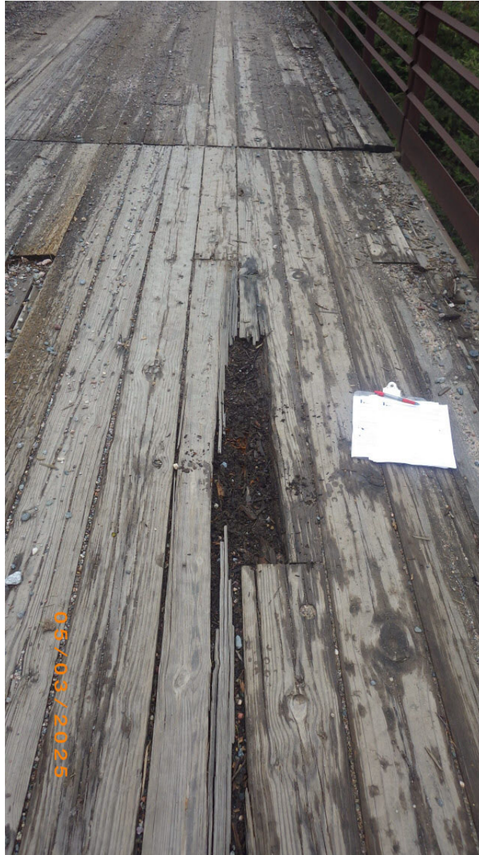
Missing / rotten wear planks
