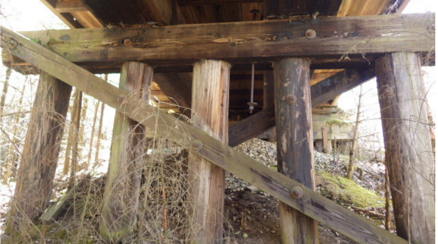
Bent #1, cap rotten / crushing
