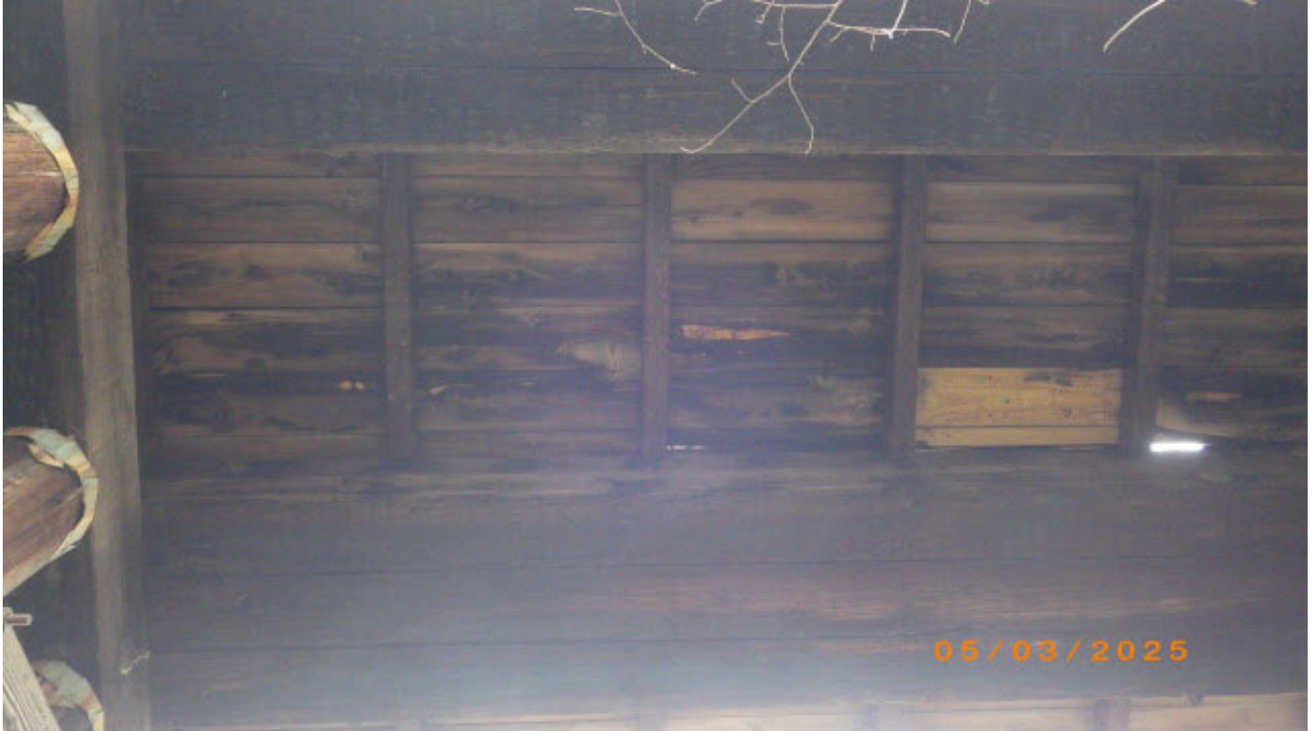
Underside of deck at hole in center of bridge. Note other rotten areas.
