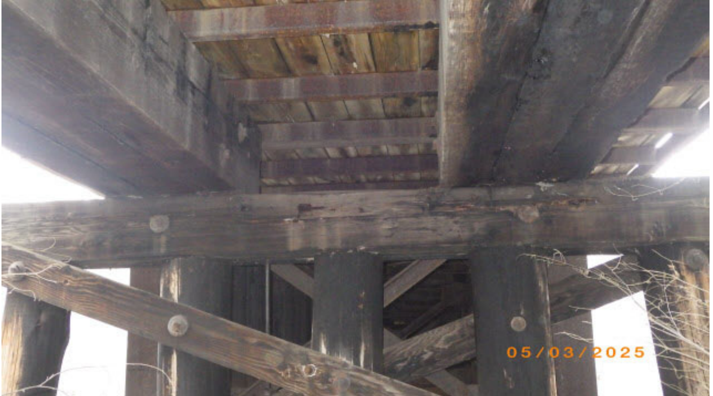
Pier #3, timber cap rotten / crushing (close-up)
