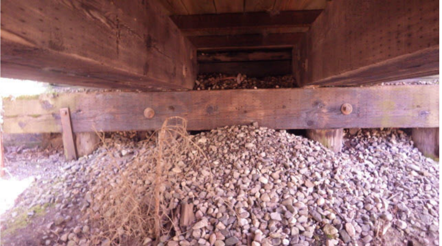
South abutment rotten piling
