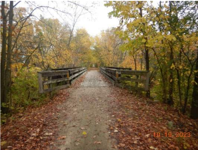
South approach looking north.
