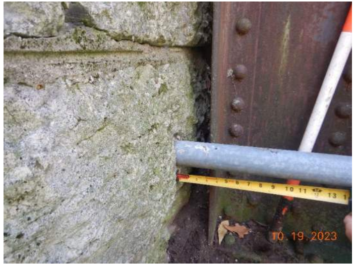
Through girder with minimal gap at backwall in NW quadrant
