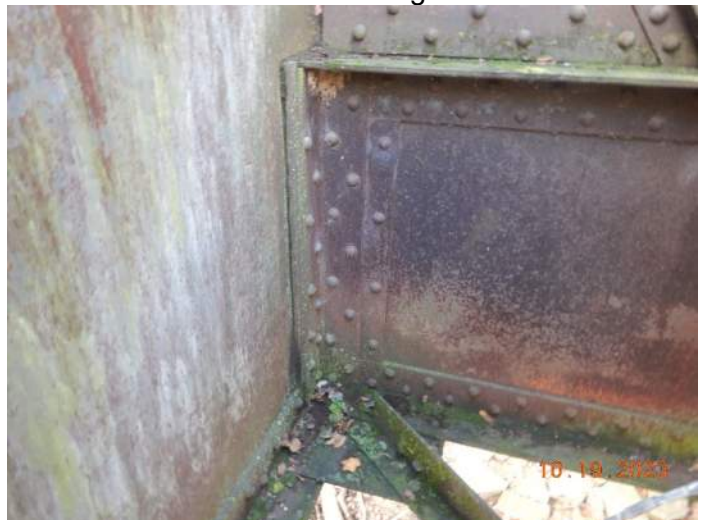
Typical through girder, floor beam, lateral bracing connection.
