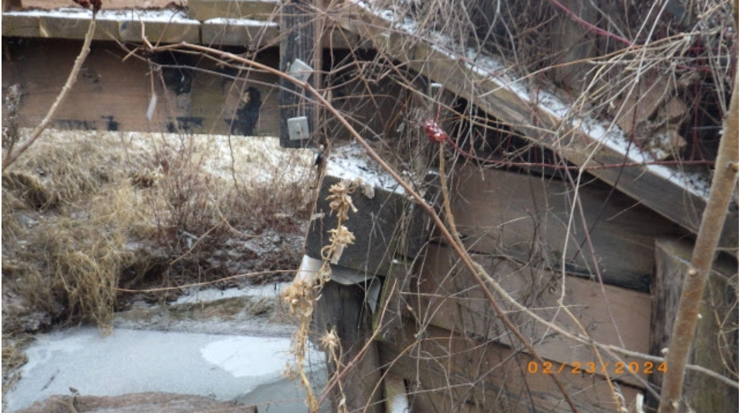
Rotated West Pile cap, looking South
