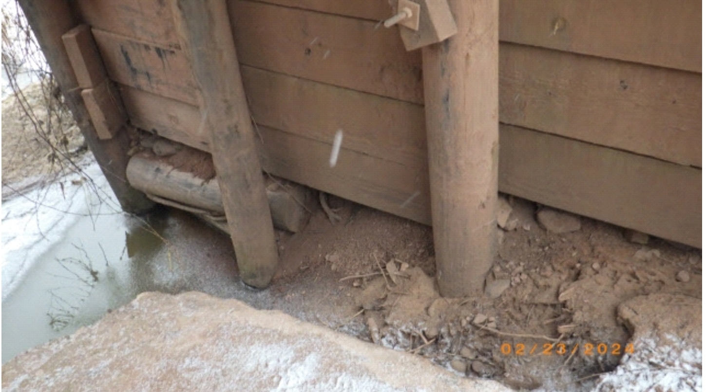
Bottom of West Abutment
