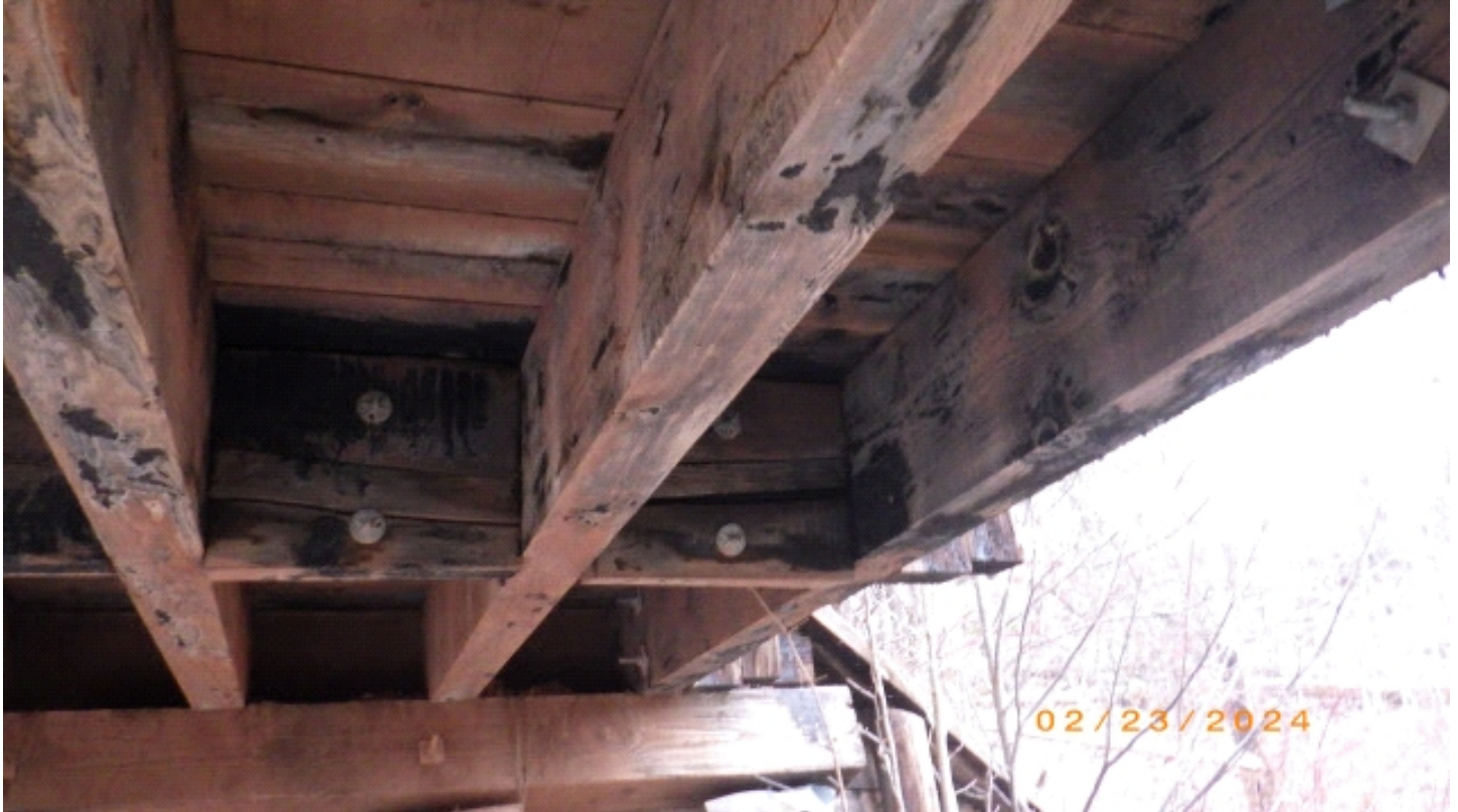
Busted Diaphragm, East line, South end.
