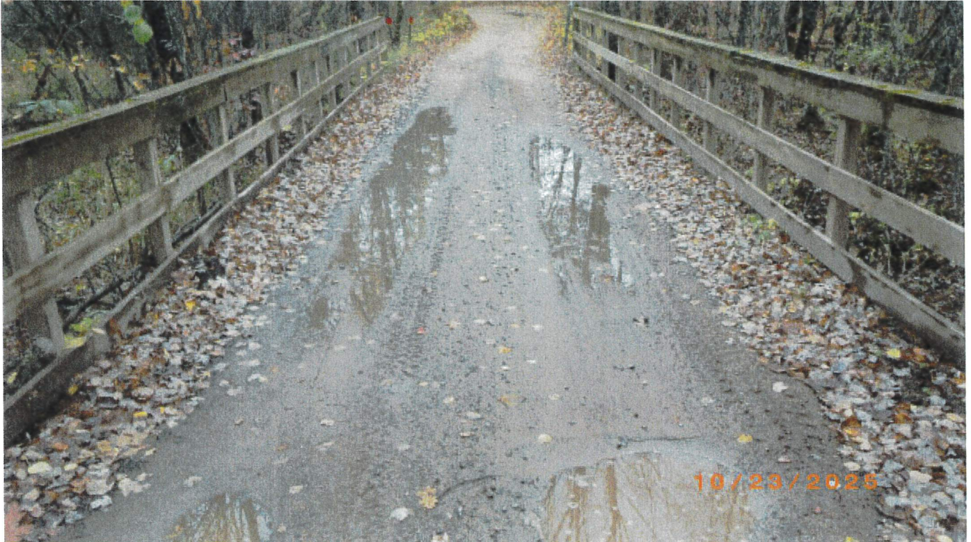
Top of deck
