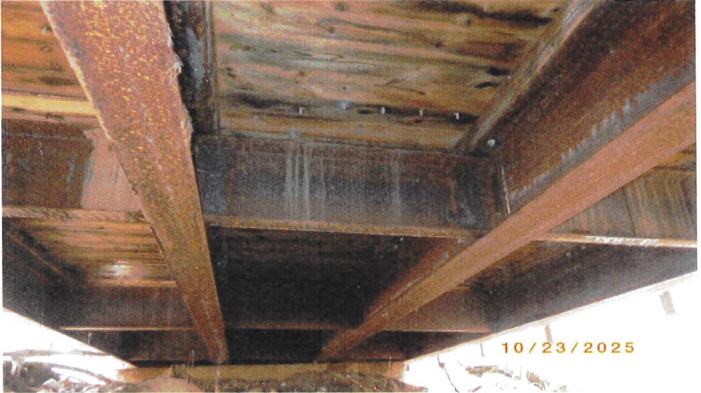
Typical deck / superstructure underside
