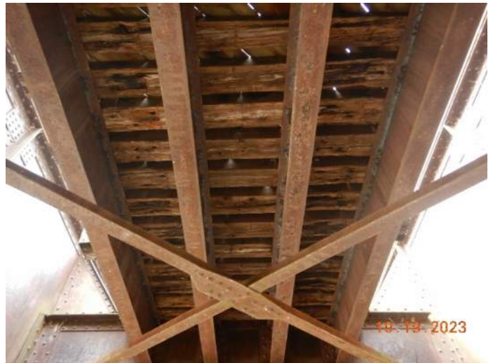
Typical deck underside.
