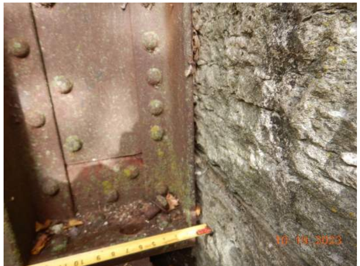
Through girder tight against backwall in NE quadrant.
