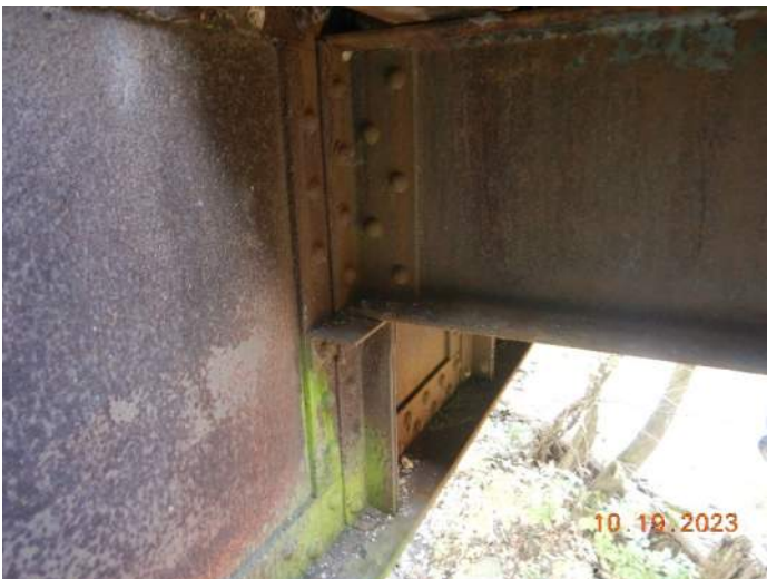
Typical floor beam to stringer connection.
