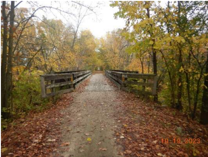
South approach looking north.
