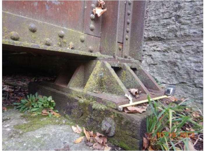
Overview of bearing (NE shown).
