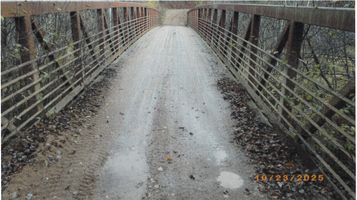
Top of deck
