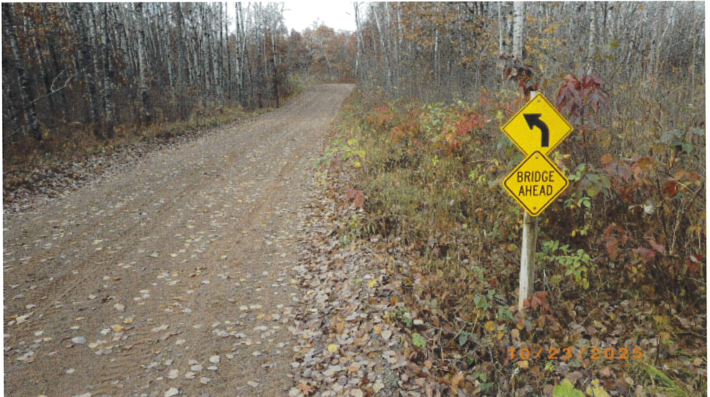
East bridge ahead sign, CS2 map cracked
