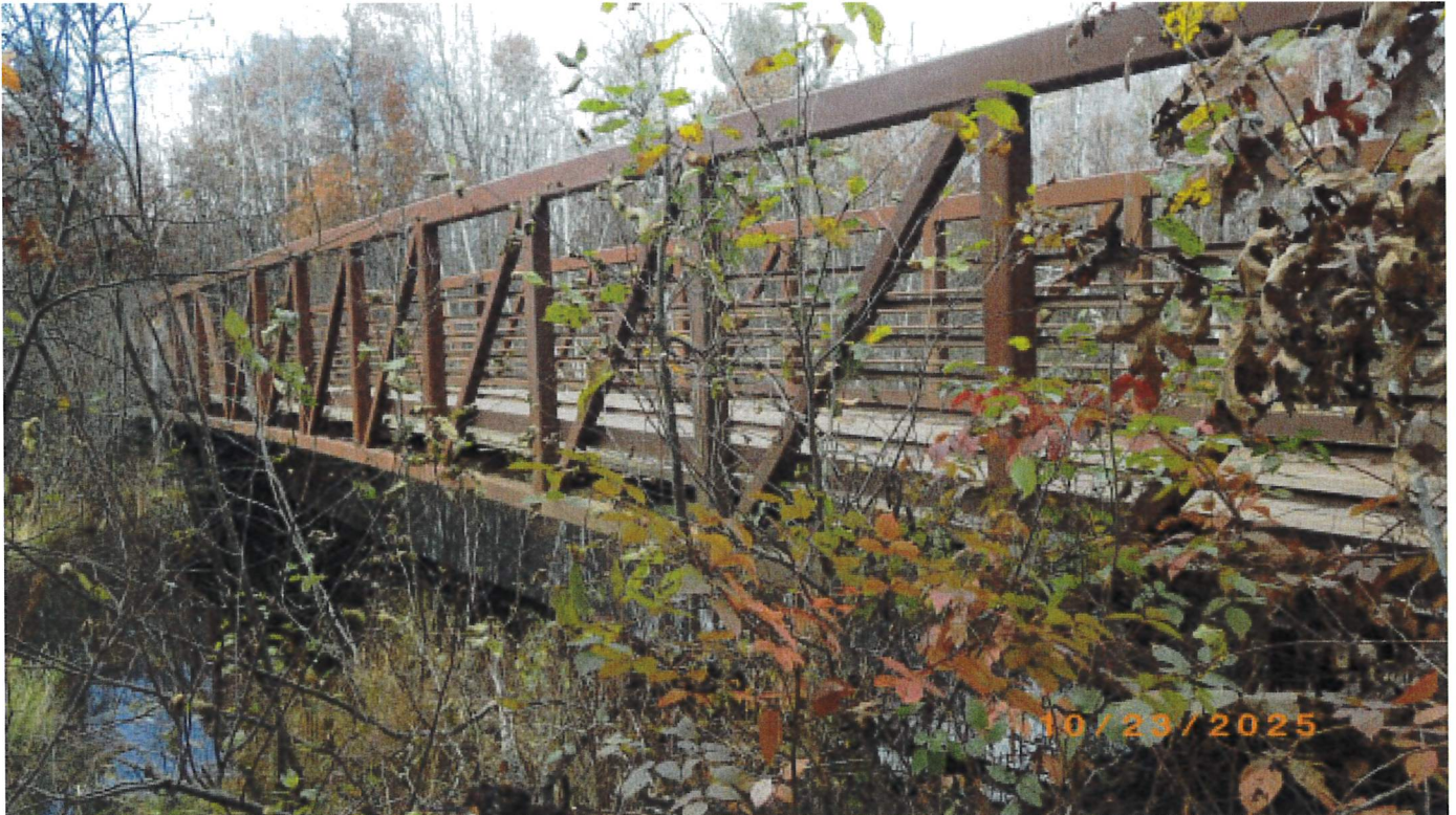
Upstream elevation view
