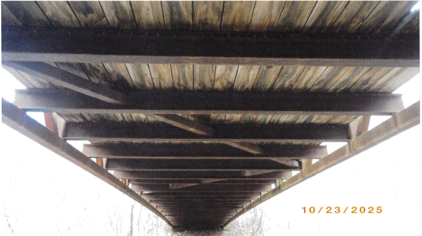
Typical deck / superstructure underside
