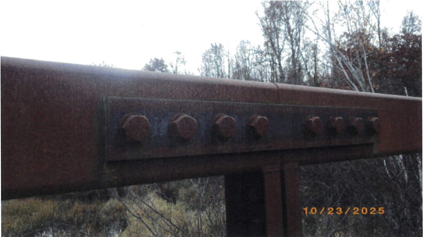
Upstream splice in good condition
