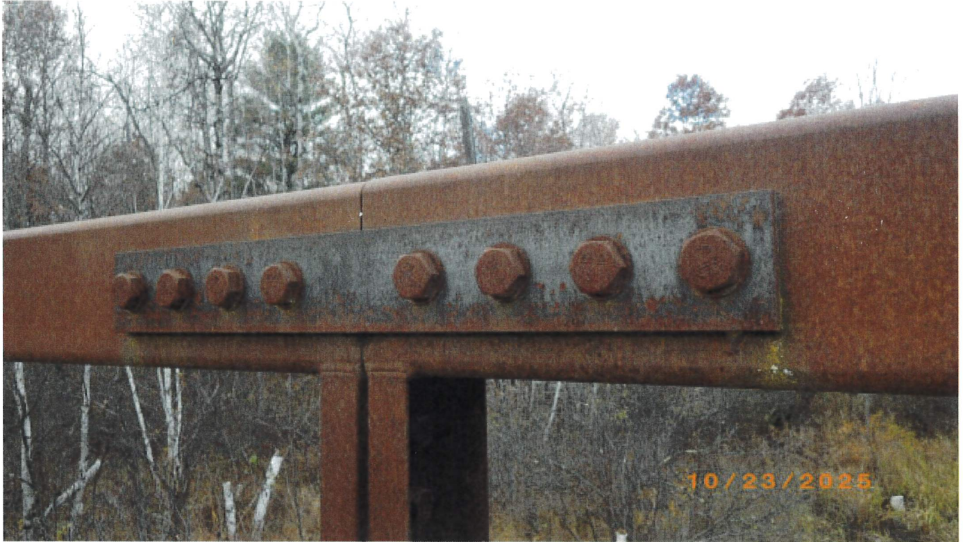
Downstream splice in good condition
