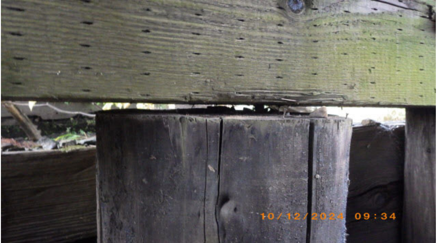
Pier 2 center pile, no bearing
