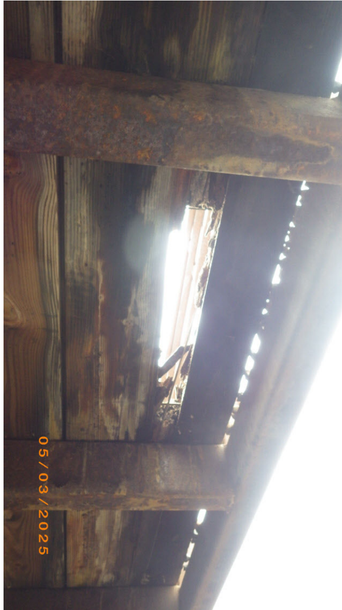
Decking rotted through, NE corner
