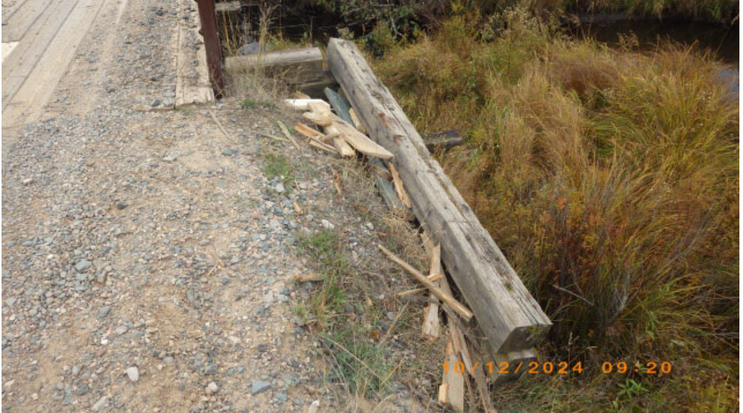
All wingwalls tipping, rotten, unstable shoulders
