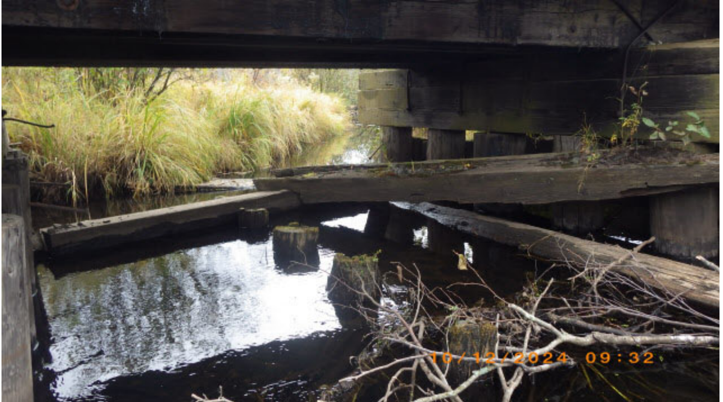
Old piling / beams catching debris in channel
