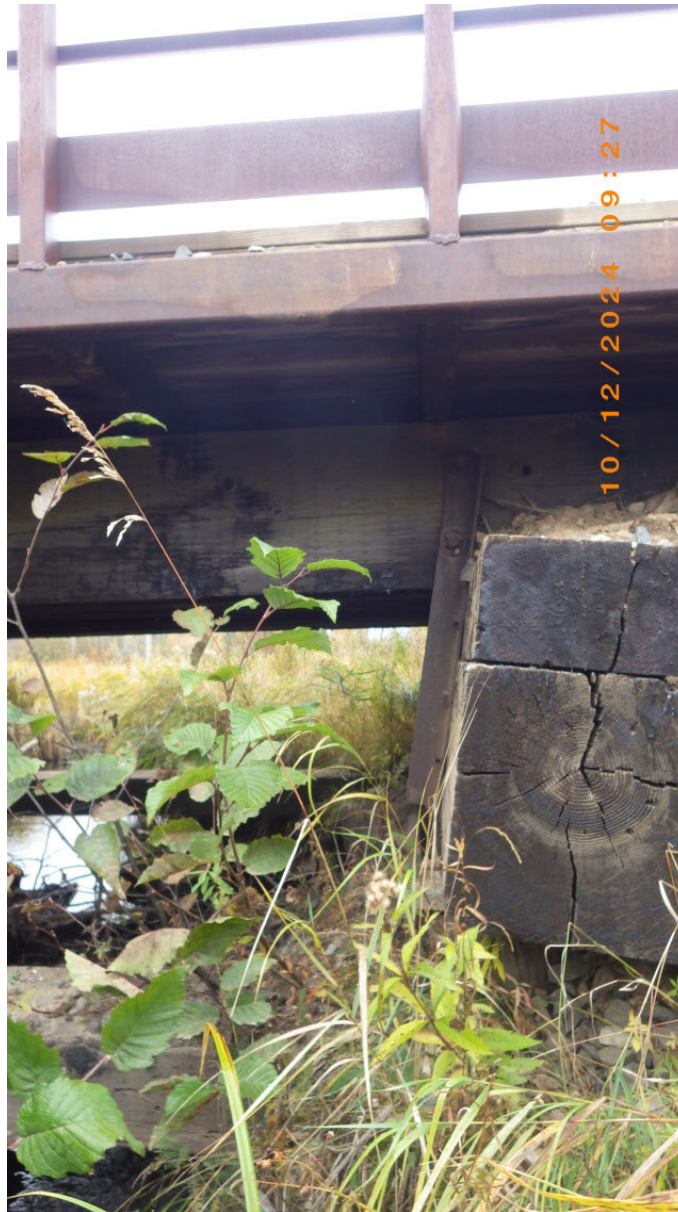
North abutment pile cap tilted back
