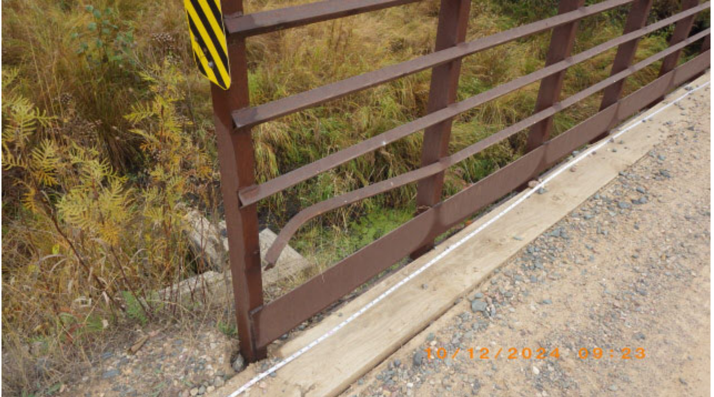
Bent lower rail, SW corner
