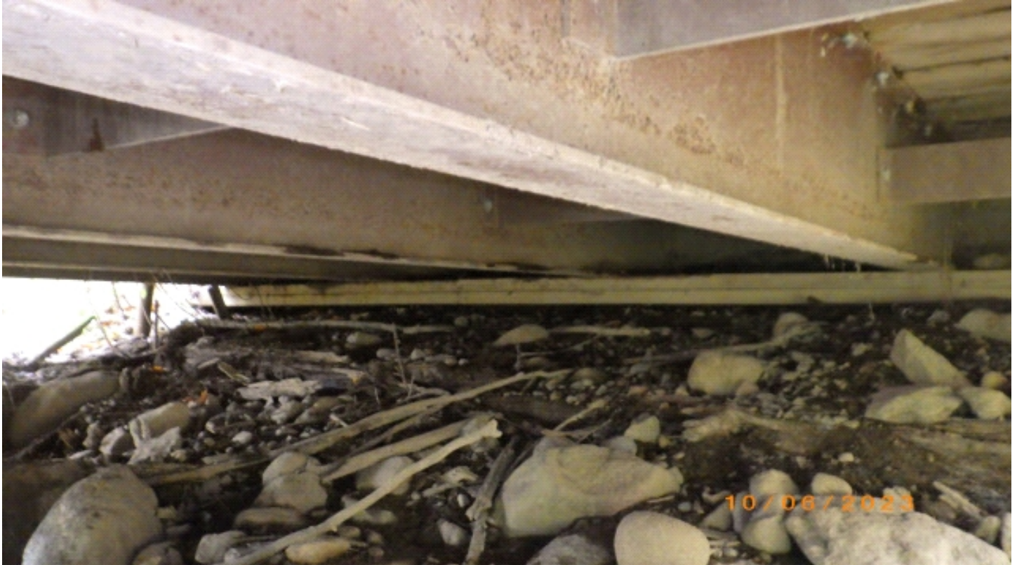
Stacked timber sill
