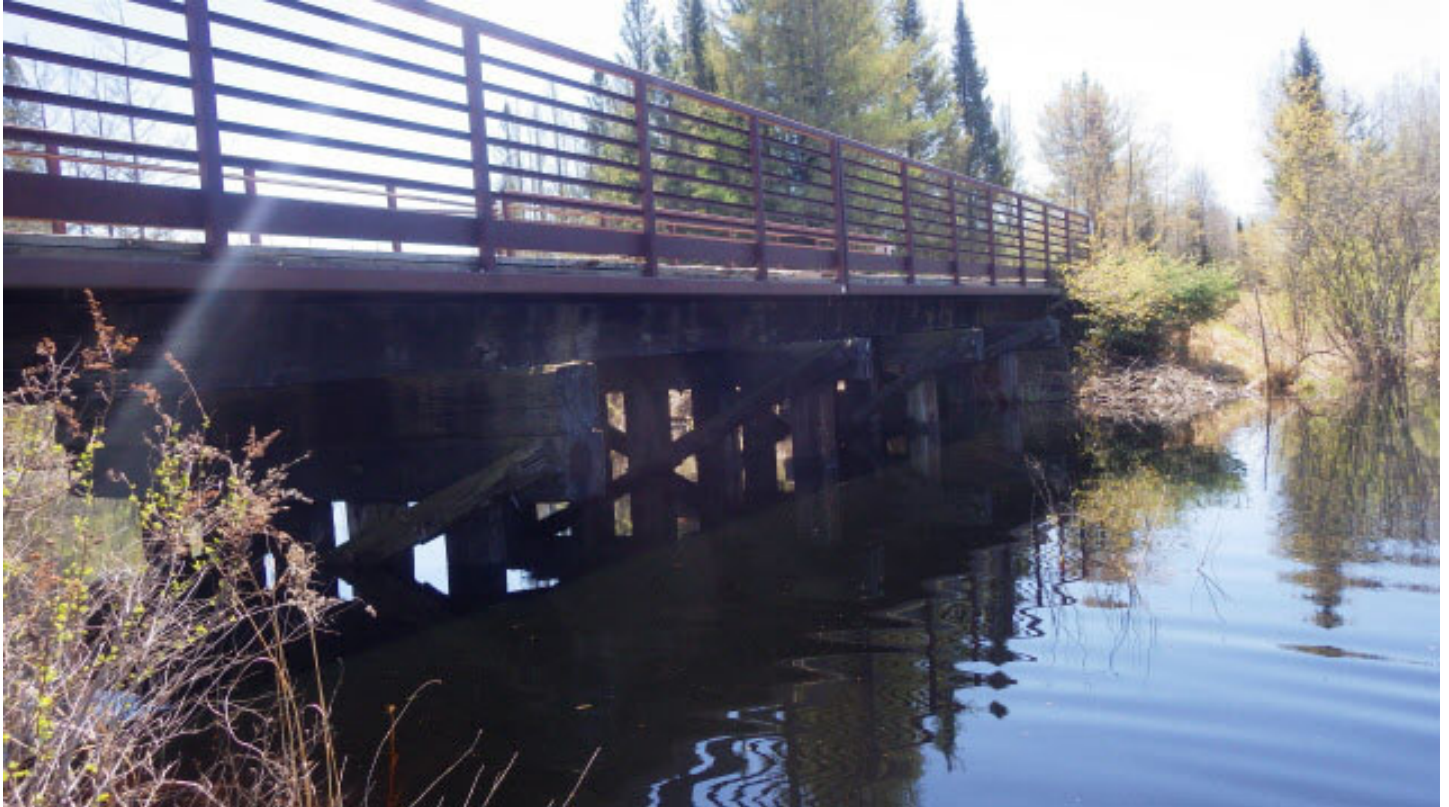
Upstream elevation view
