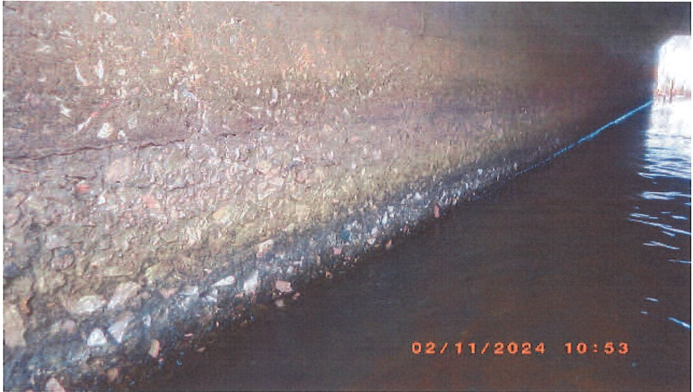
CS2 scaling on wetted perimeter of box
