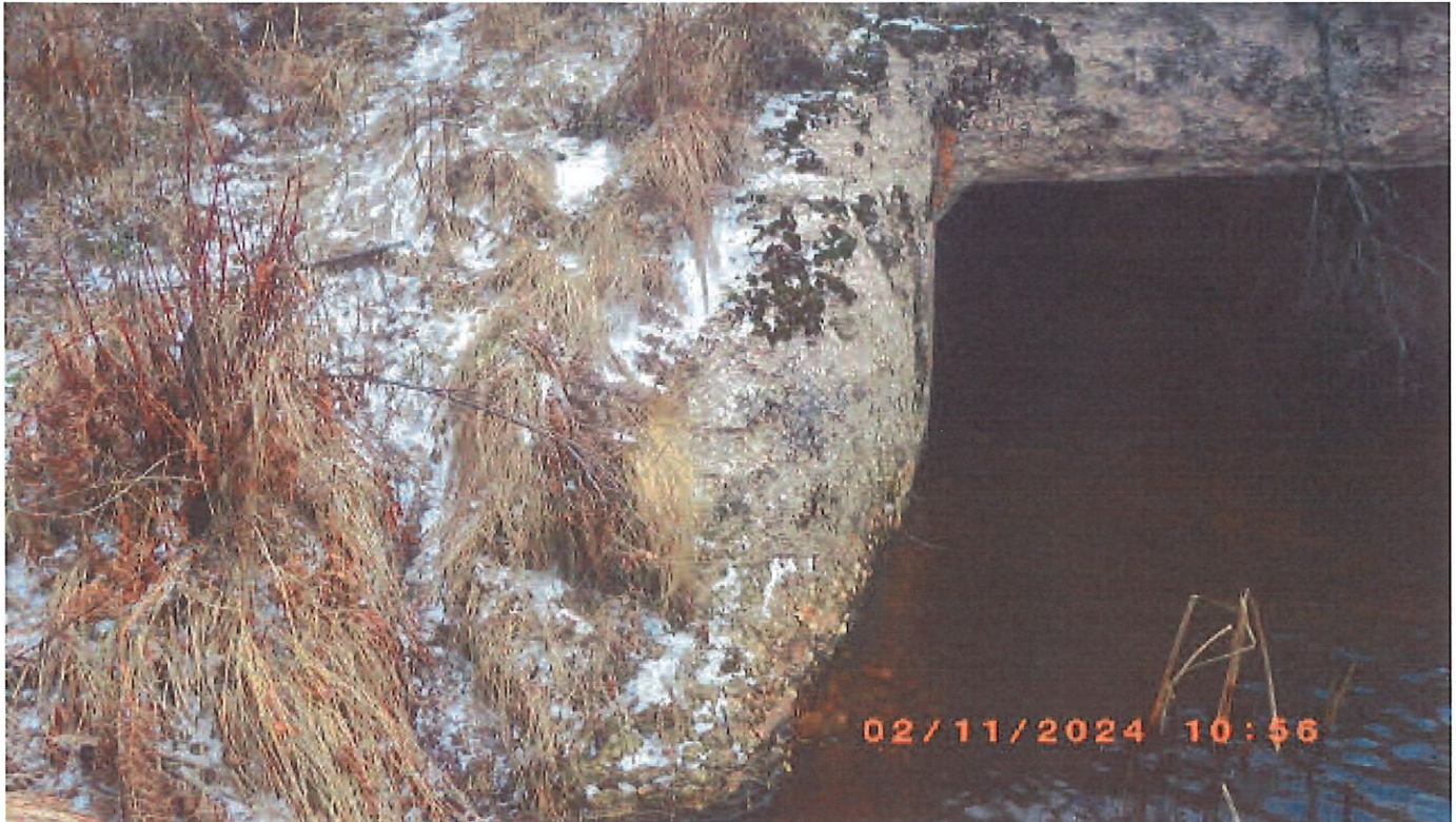
NW wingwall section loss
