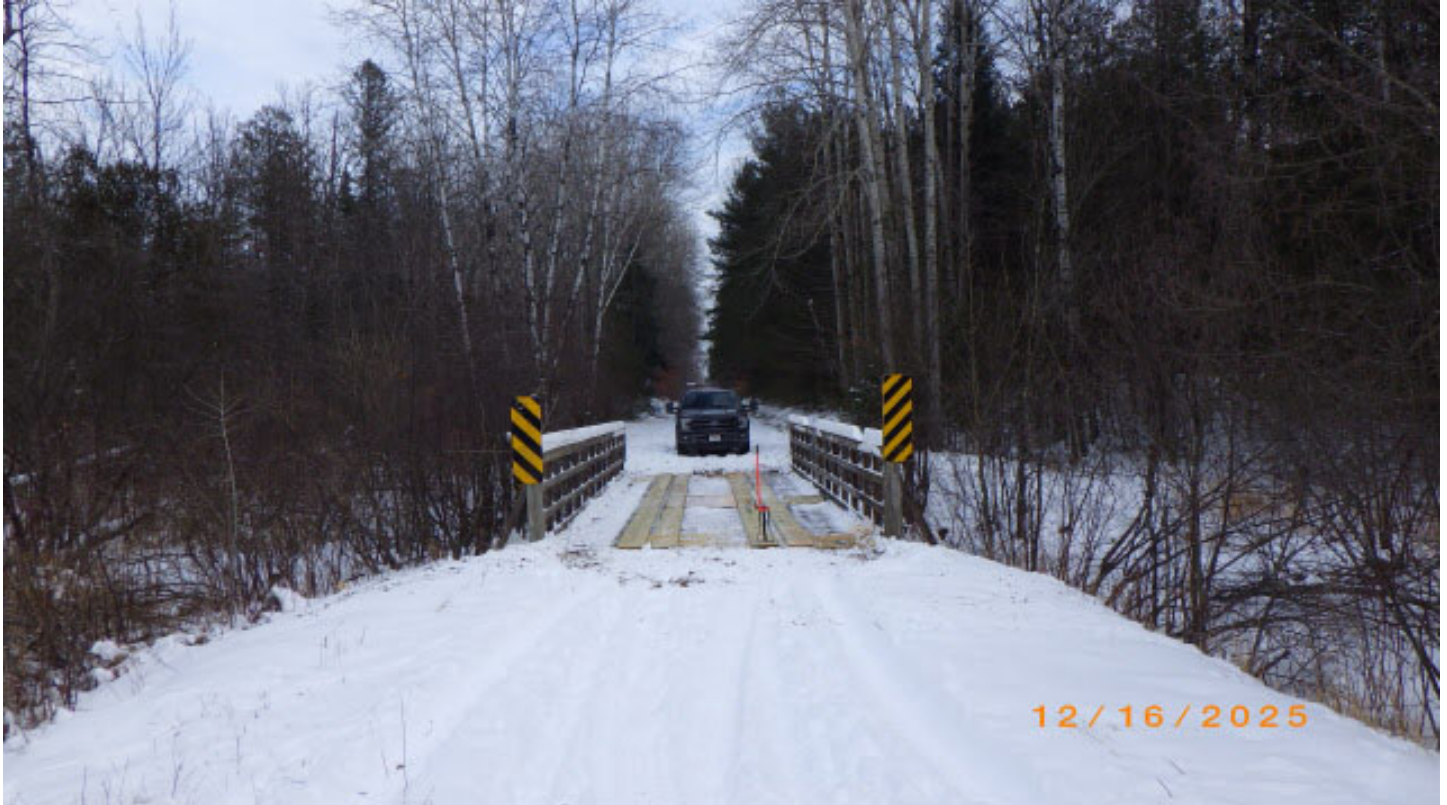
West approach / top of deck
