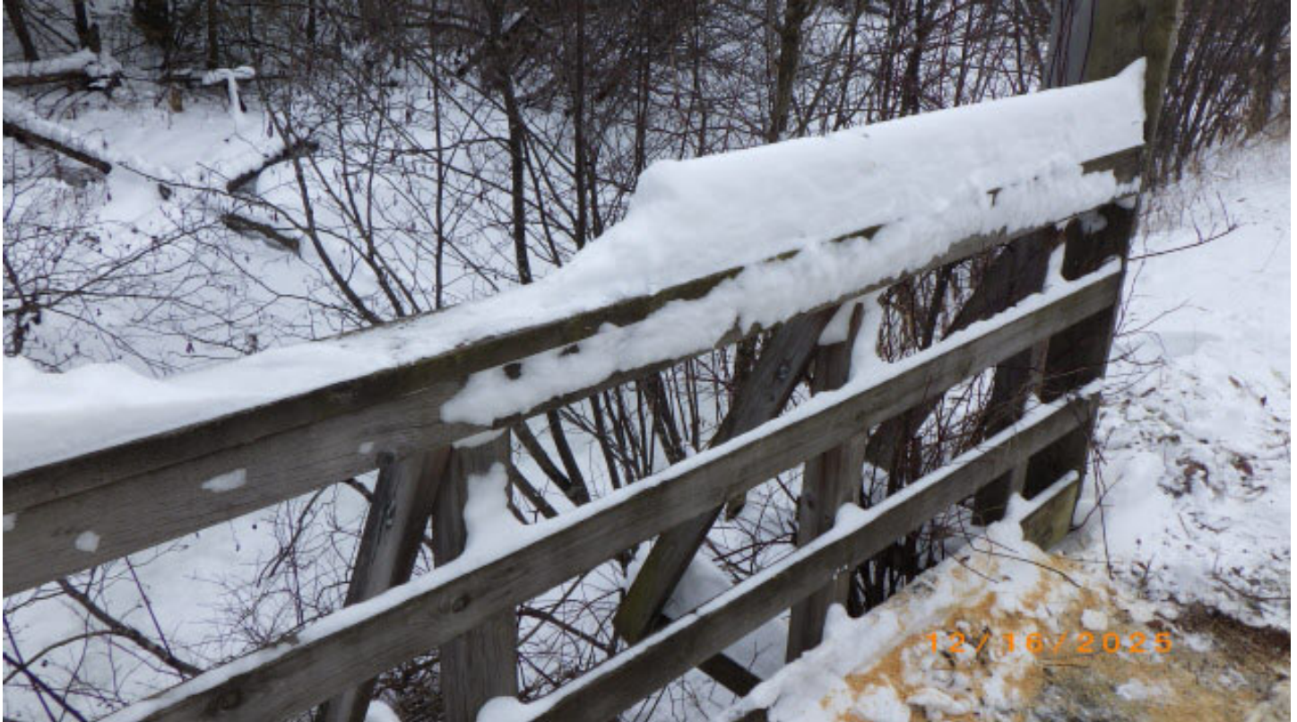
Brush around bridge ends
