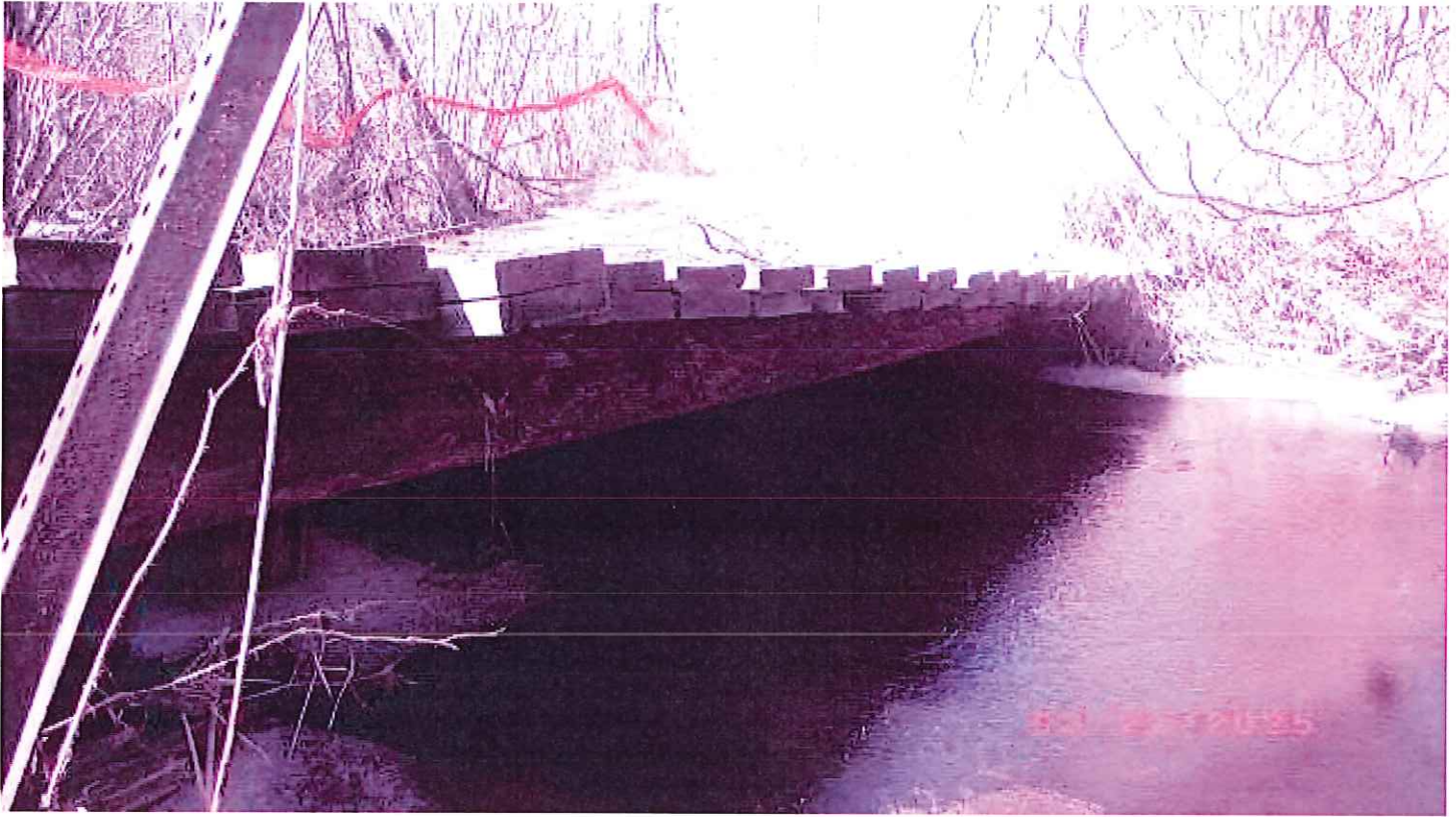
Downstream elevation / rotten log stringers
