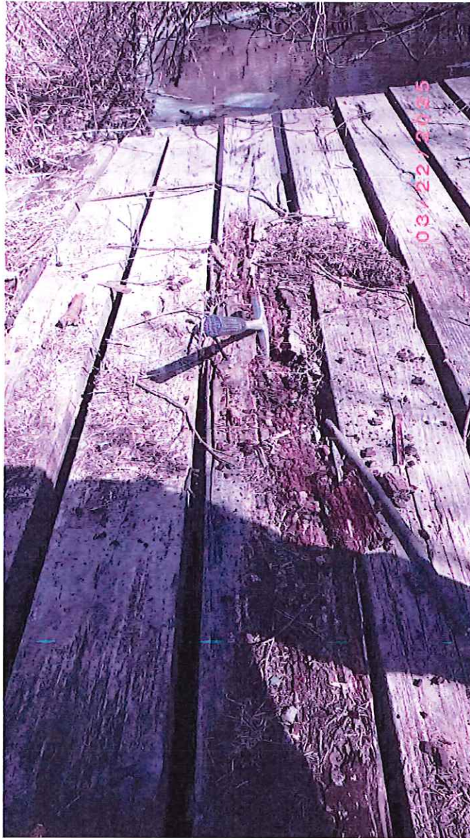
CS4 rotten deck planks
