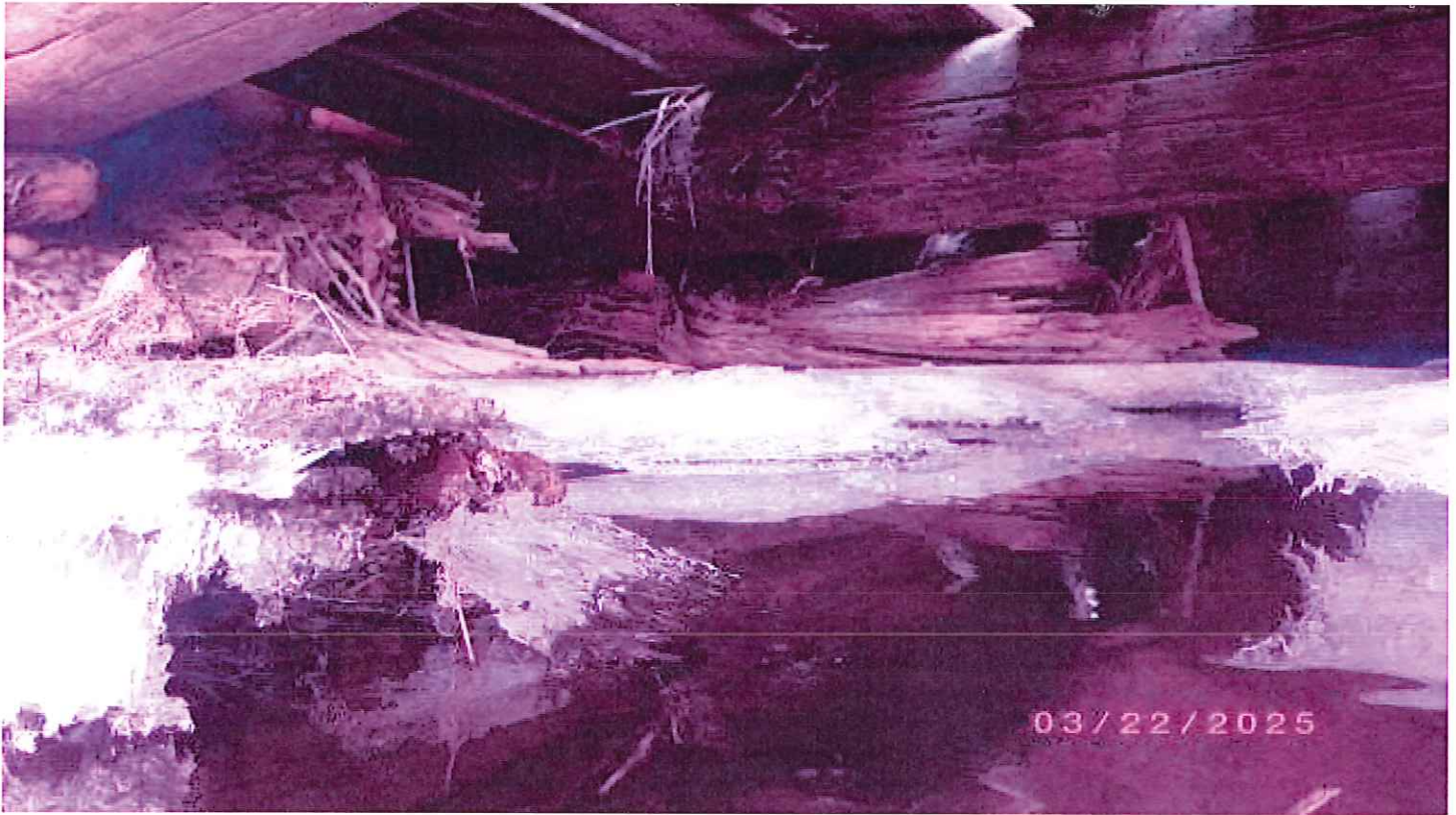
East abutment missing
