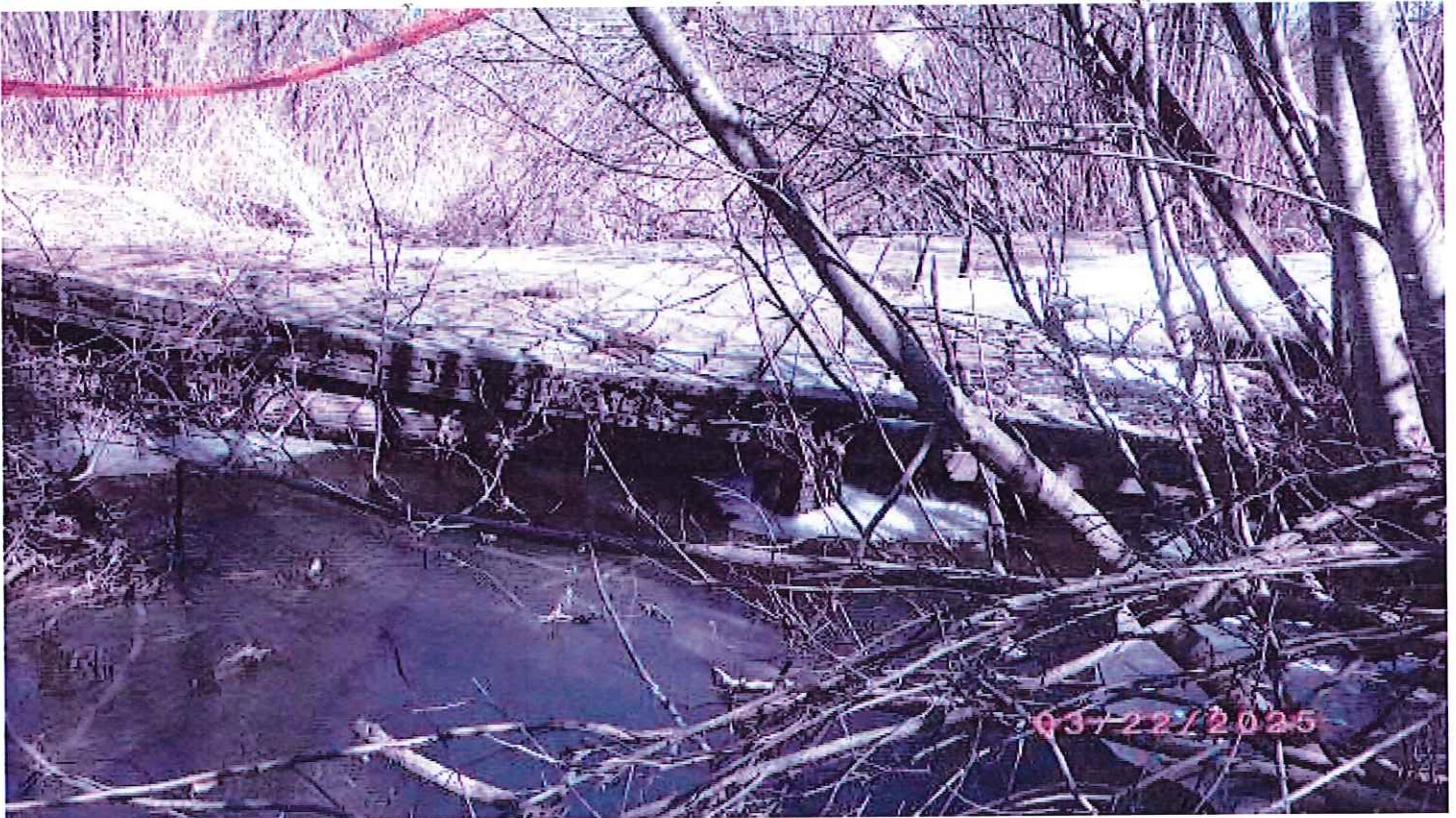
Upstream elevation view. Note severe distortion in superstructure / deck.
