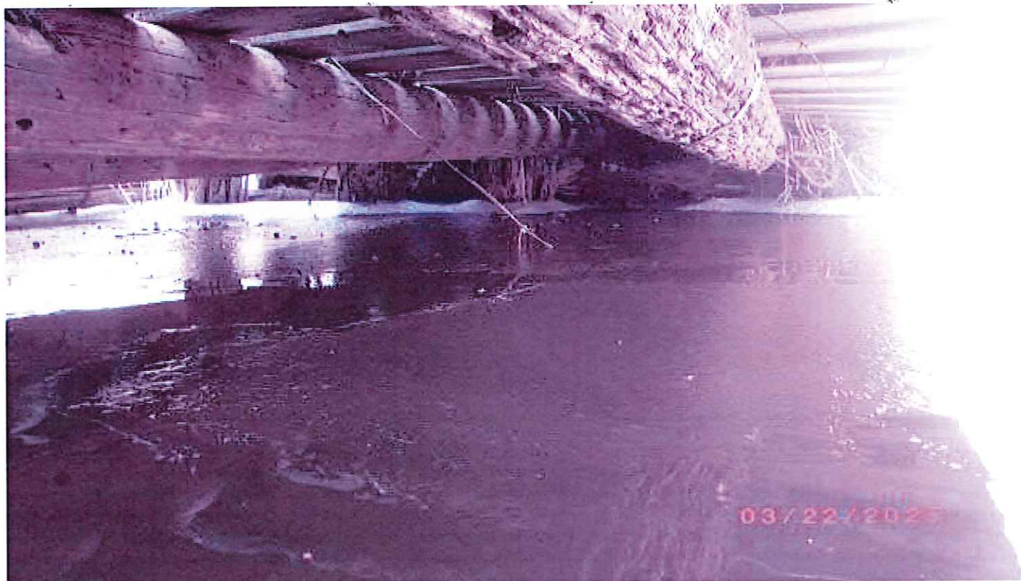
Typical bridge under side / west abutment missing
