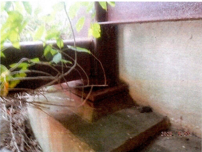
Typical Bearing Condition
