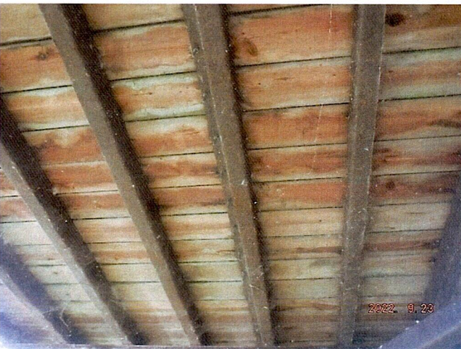
Typical Deck Underside
