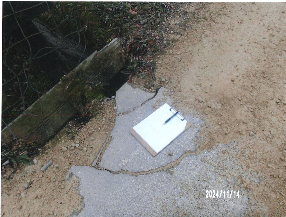
Figure 6: NW Deck Corner Failed Due to Loss of Support– SE similar
