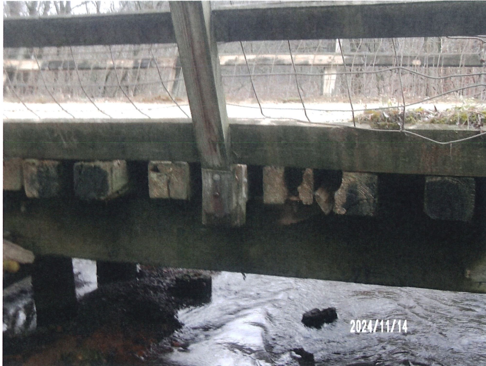
Figure 7: Timber Stringer Splitting
