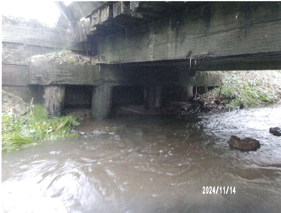
Figure 9: Typical Abutment
