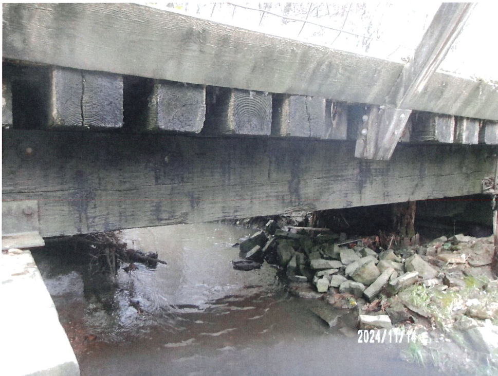
Figure 8: Narrow Split and Debris Damage on Girder
