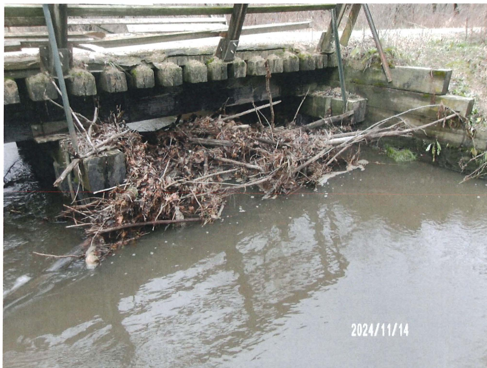
Figure 14: Debris at Upstream side
