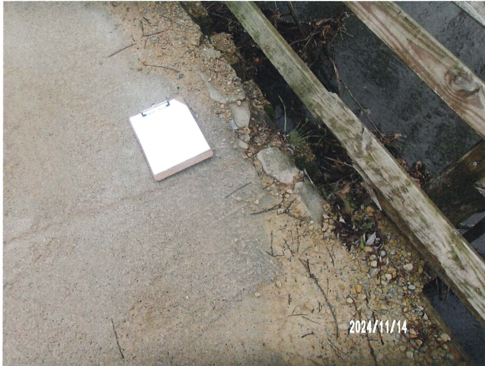
Figure 7: Deck Edge Starting to Spall Off
