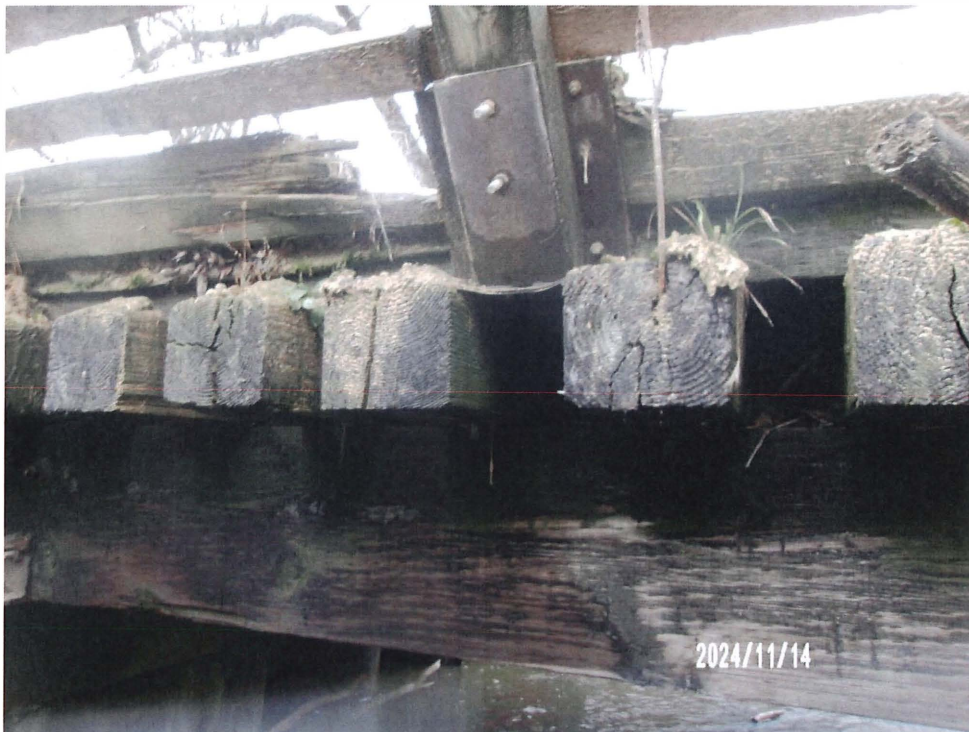
Figure 8: Typical Floor Beam Splitting
