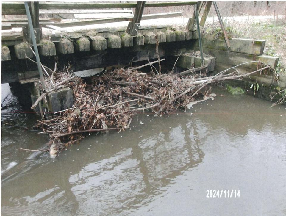
*Figure 14: Debris at Upstream side*
