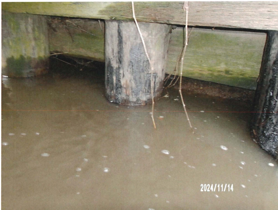
Figure 12: Undermining at North Abutment
