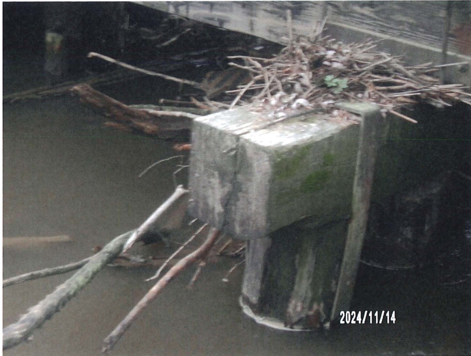
Figure 11: East End of Cap Split
