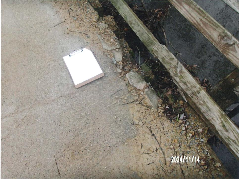
*Figure 7: Deck Edge Starting to Spall Off*
