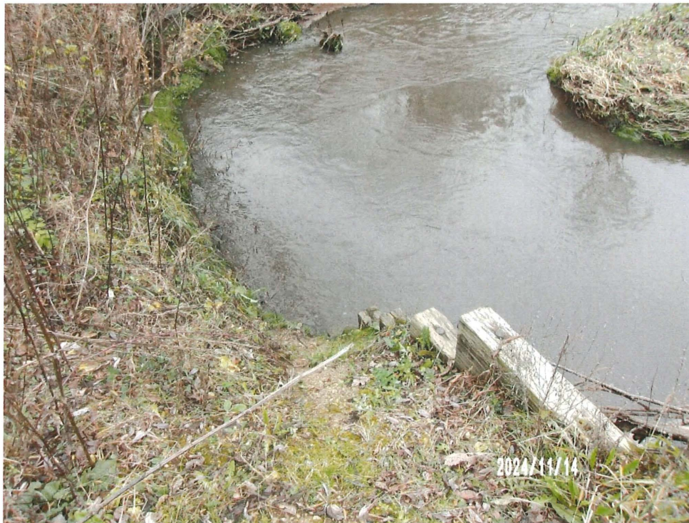
Figure 13: Stream Migrating Behind South Abutment
