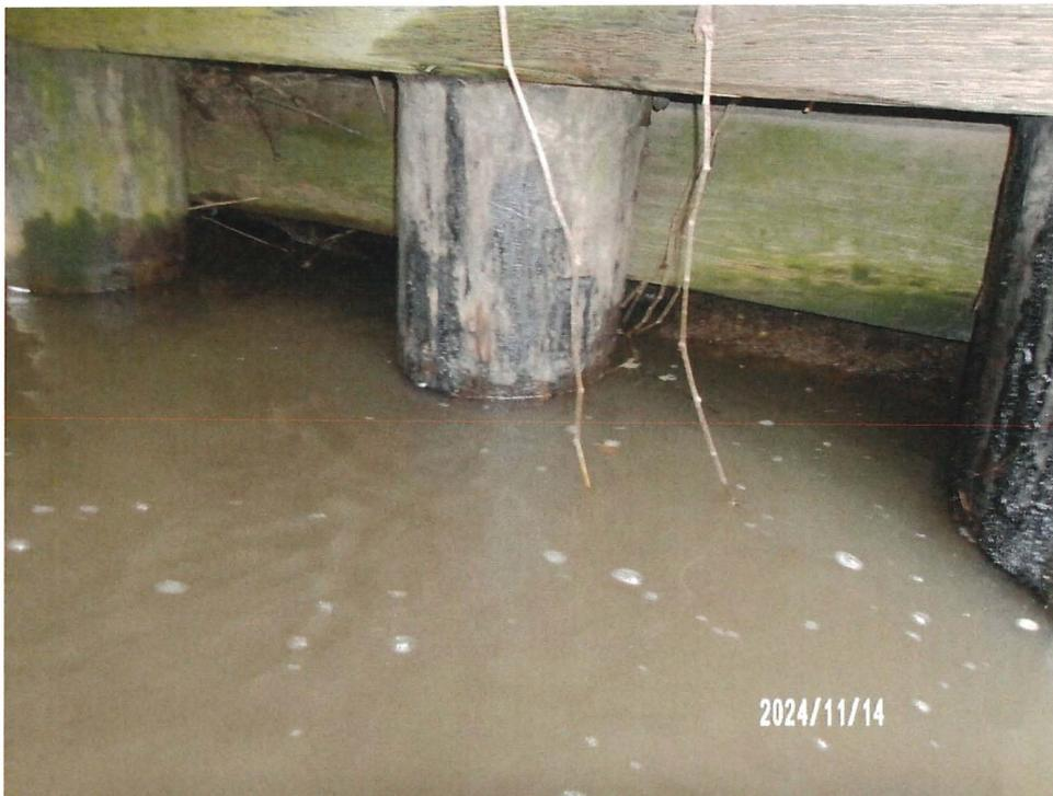
*Figure 12: Undermining at North Abutment*
