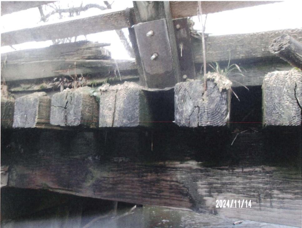
*Figure 8: Typical Floor Beam Splitting*
