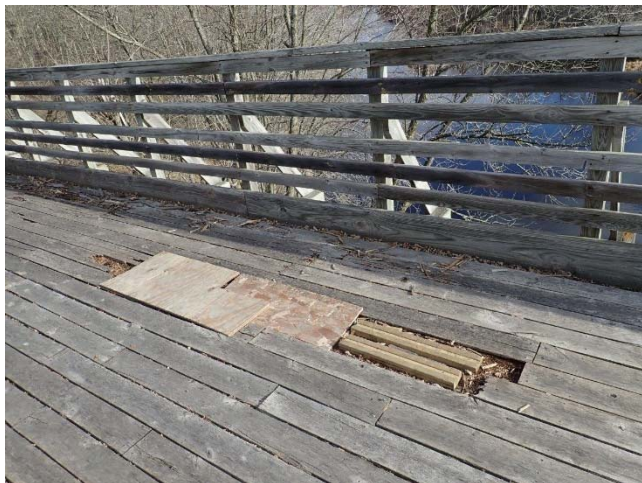
Wearing surface is aging but mostly intact. Several locations need proper replacements or repairs.
