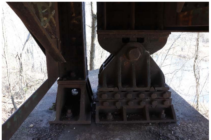
Cracked bearing at pier 3, east side
