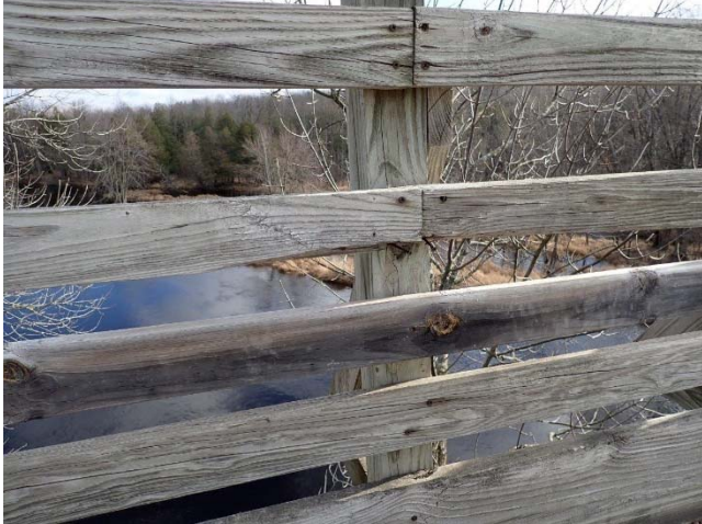
Railing shows signs of age but also has several damaged or decaying locations.
