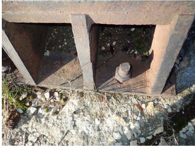
Cracked bearing at pier 3, east side
