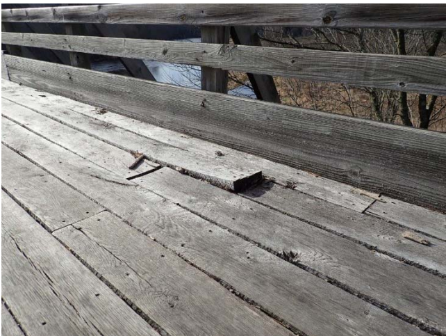
Wearing surface is aging but mostly intact. Several locations need proper replacements or repairs.
