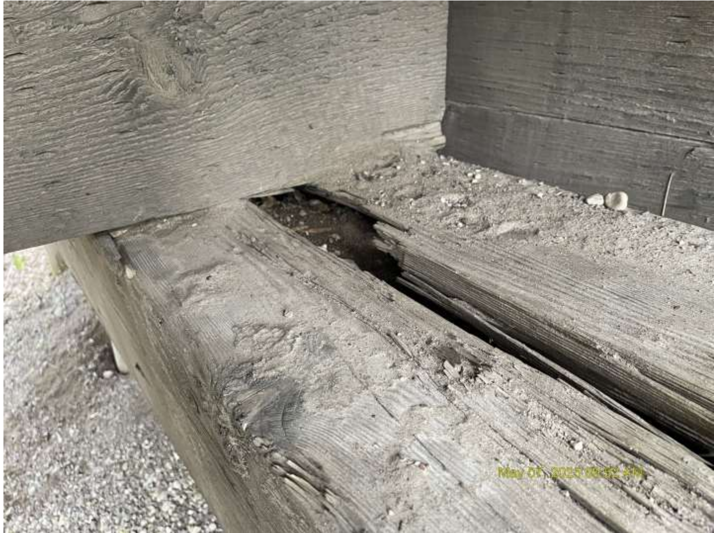
West pier cap north side
