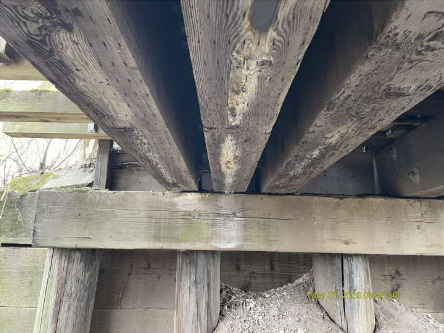
Looking east – north girders
