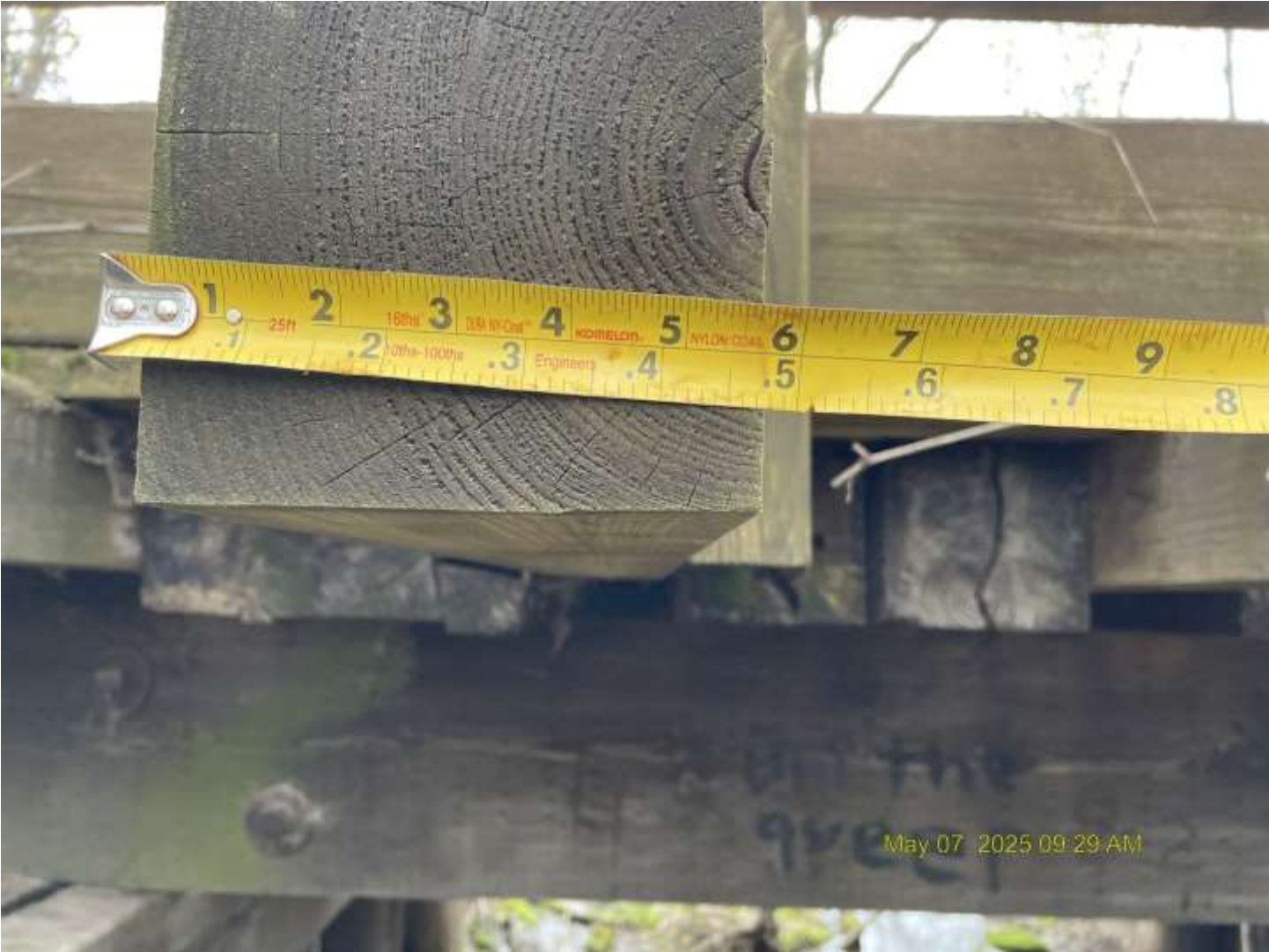
Fence ties measurement
