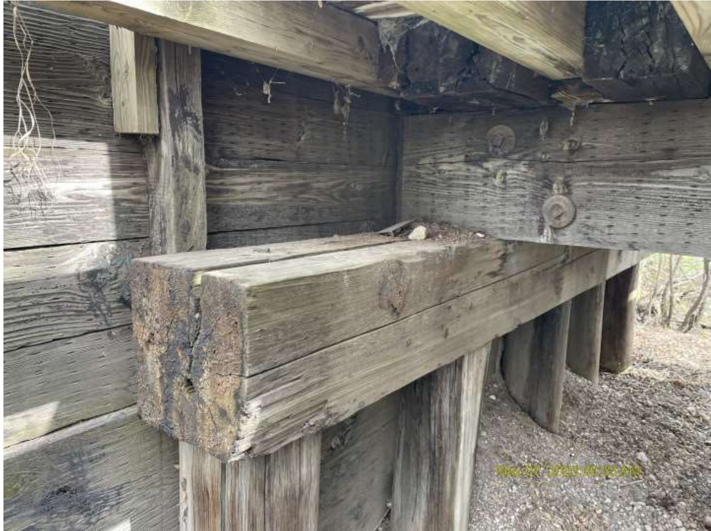
West pier cap south side
