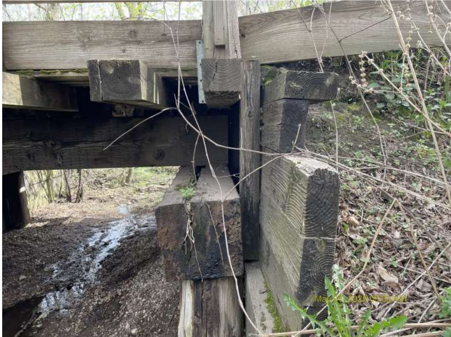
East pier cap south side
