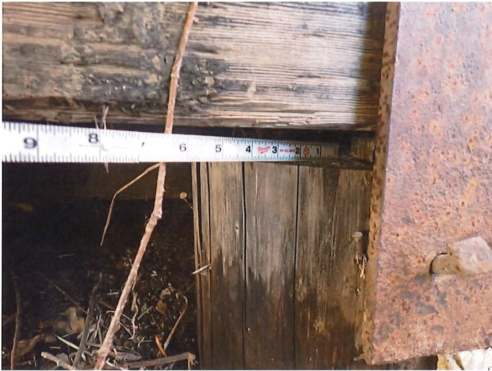
View of pile not bearing on east abutment pier cap, looking east.
