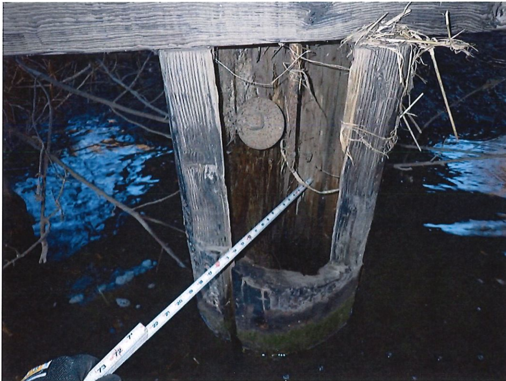
View of typical heavily decayed pile, looking west.
