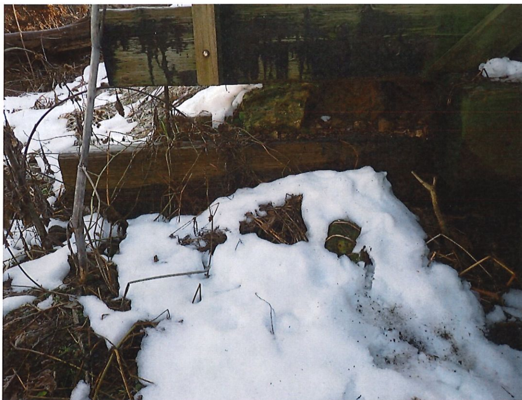
View of gap in east abutment backwall, looking east.
