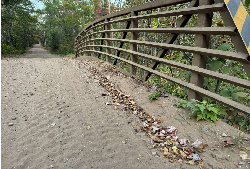
Downstream side. Sand windrow at edges
