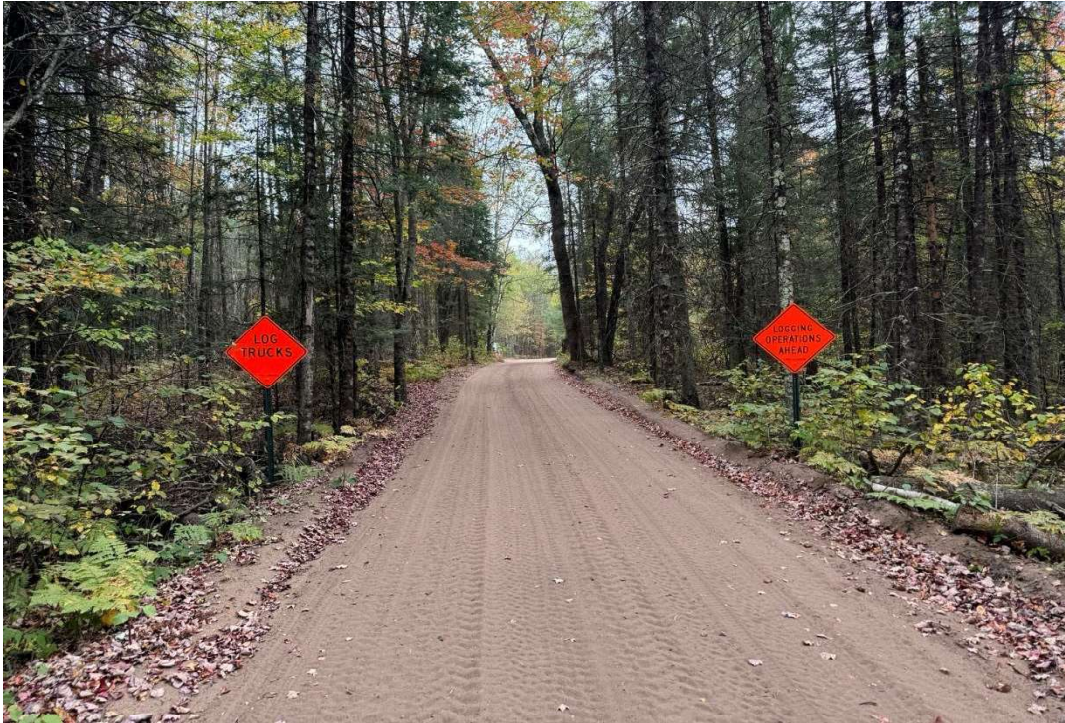
Signs looking south. Log trucks should not use this bridge
