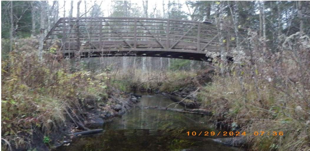
Looking Upstream - Elevation Profile
