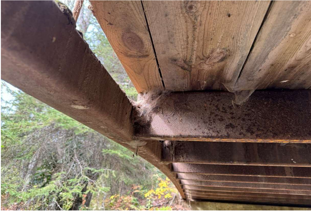
Typical floorbeam connection
