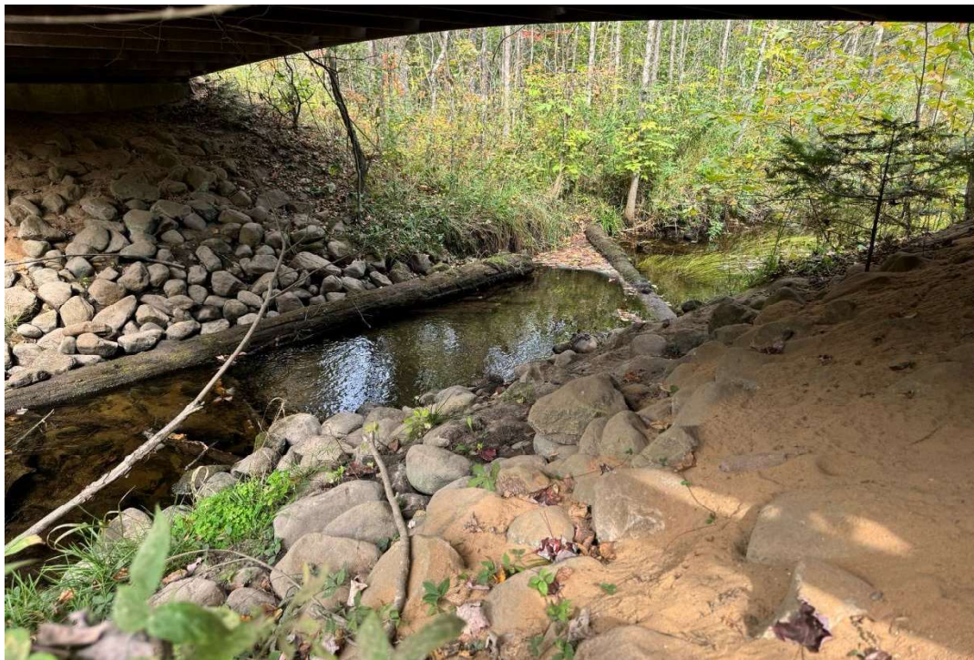
Channel under bridge
