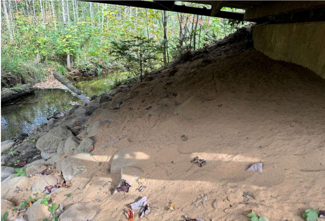
South riprap slope looking DS
