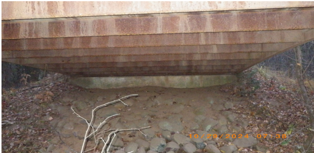
River Left Abutment
