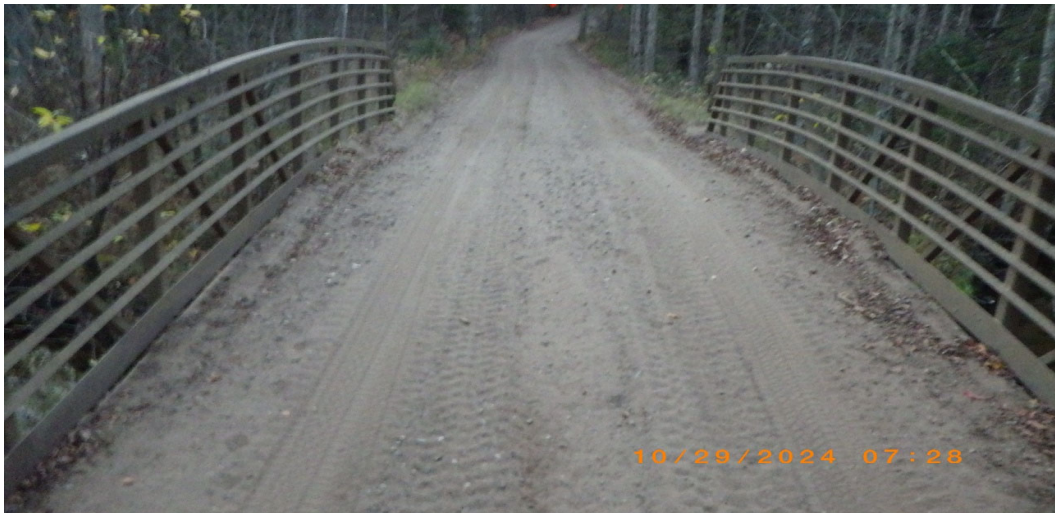
View of Deck and Rails
