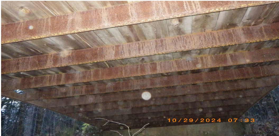
View of Superstructure
