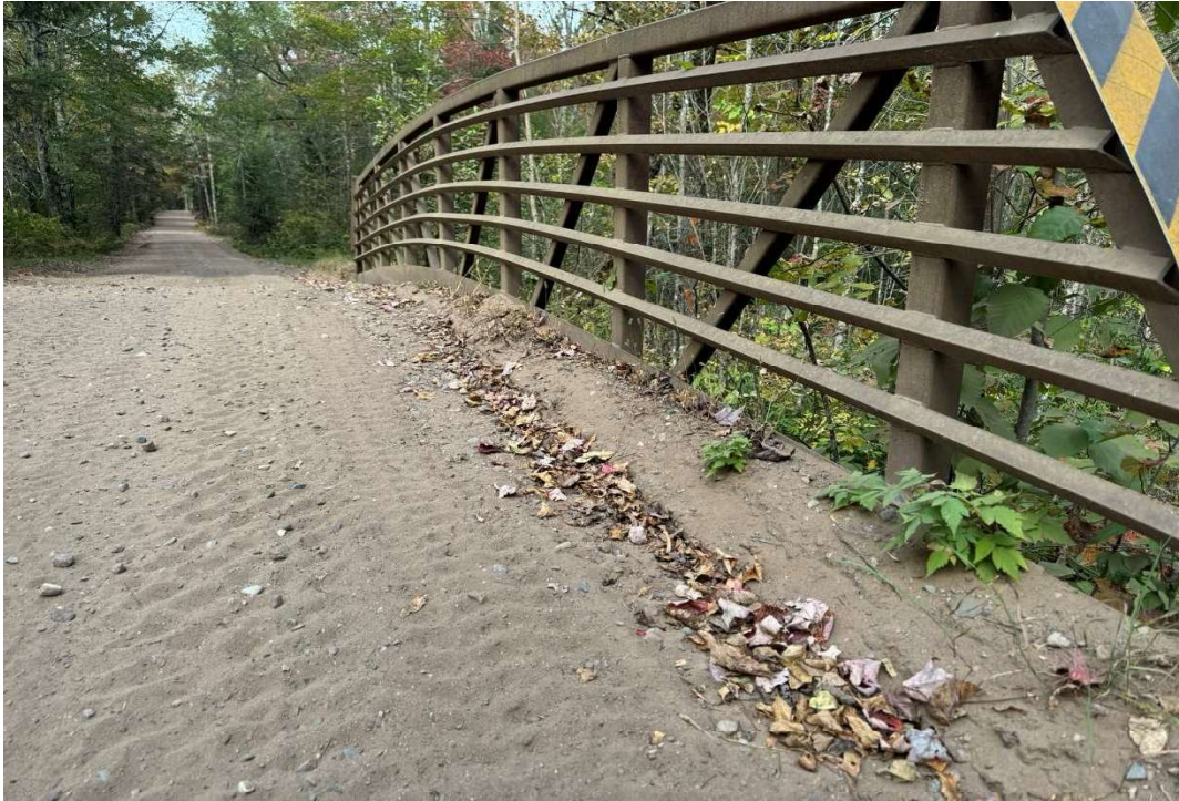
Downstream side. Sand windrow at edges
