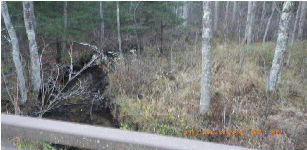
Looking Upstream from the Bridge Deck
