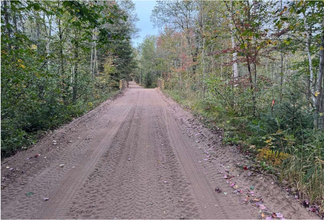
Hay Creek Bridge - looking north
