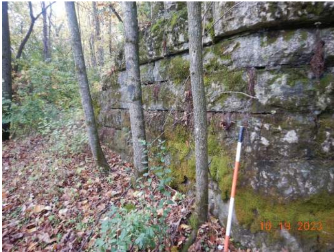
Typical tree growth along wingwalls (fascia similar).
