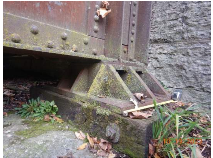
Overview of bearing (NE shown).
