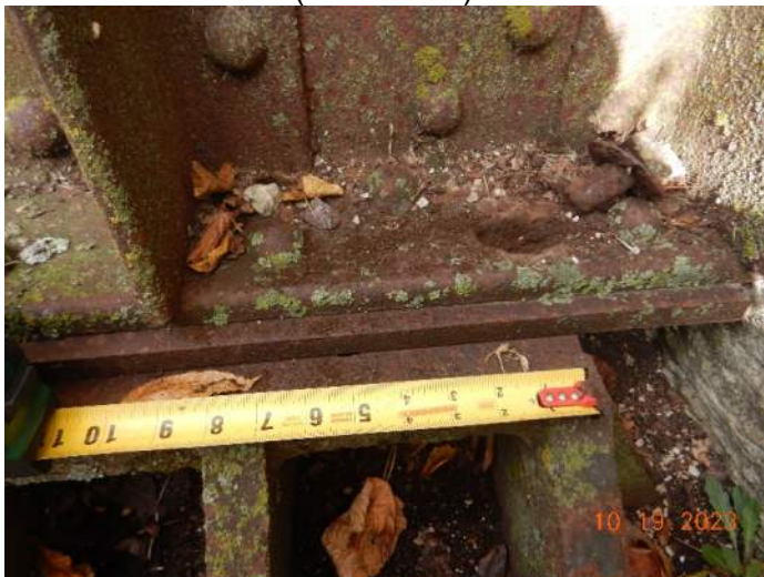
Broken keeper rod at the NE bearing.
