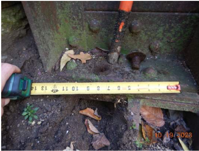
Broken keeper rod at the NW bearing
