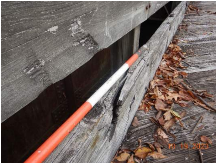
Split toe rail in the NE quadrant.
