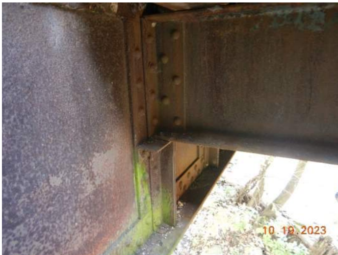
Typical floor beam to stringer connection.
