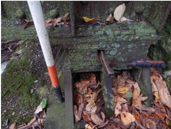
Hole in filler plates at SW bearing.
