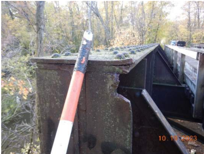
Minor damage to through girder NE quadrant.
