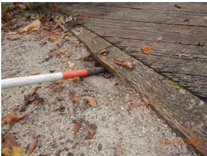
Minor sinkhole at the north approach.
