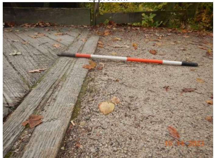
Typical settlement of gravel approaches (south shown).
