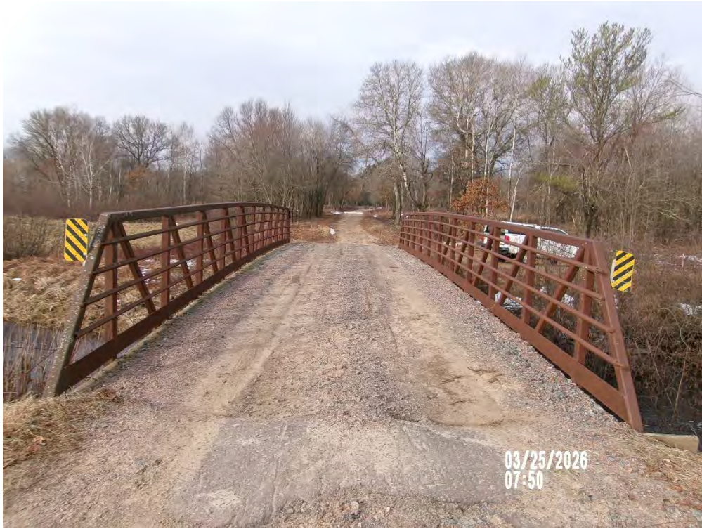
Figure 1 East Approach Looking West
