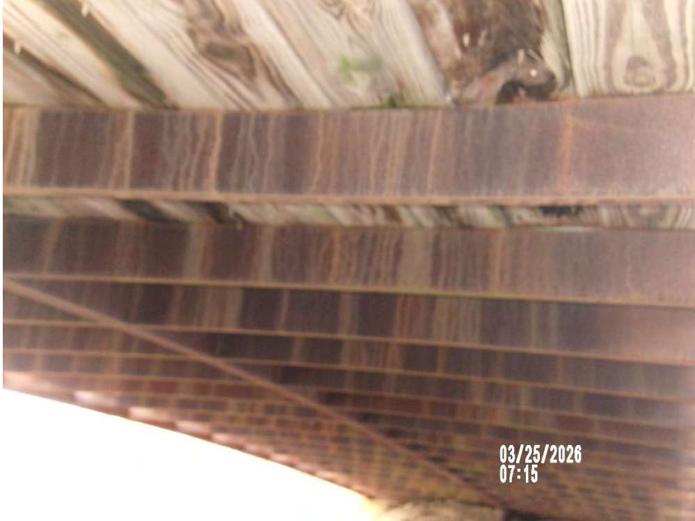
Figure 11: Typical floor beam condition
