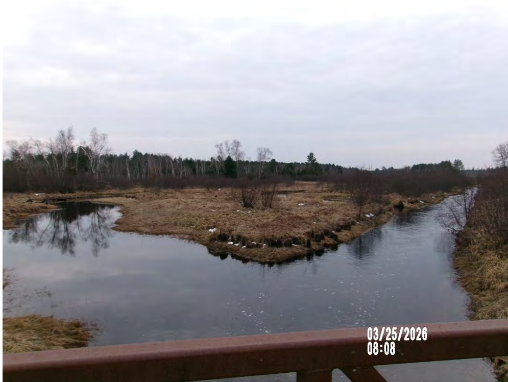
Figure 3: Looking Upstream from Top of Deck
