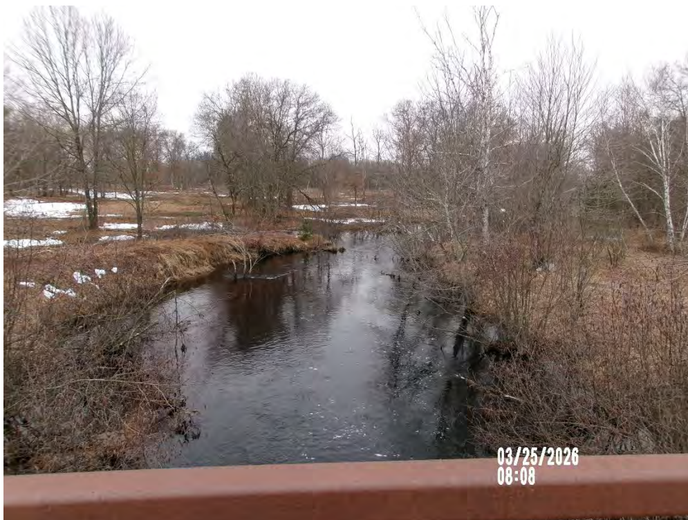
Figure 4: Looking Downstream from Top of Deck
