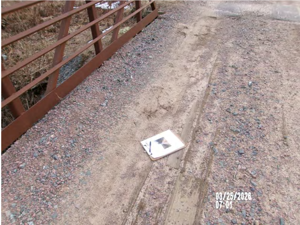
Figure 5: Wearing surface with gravel
