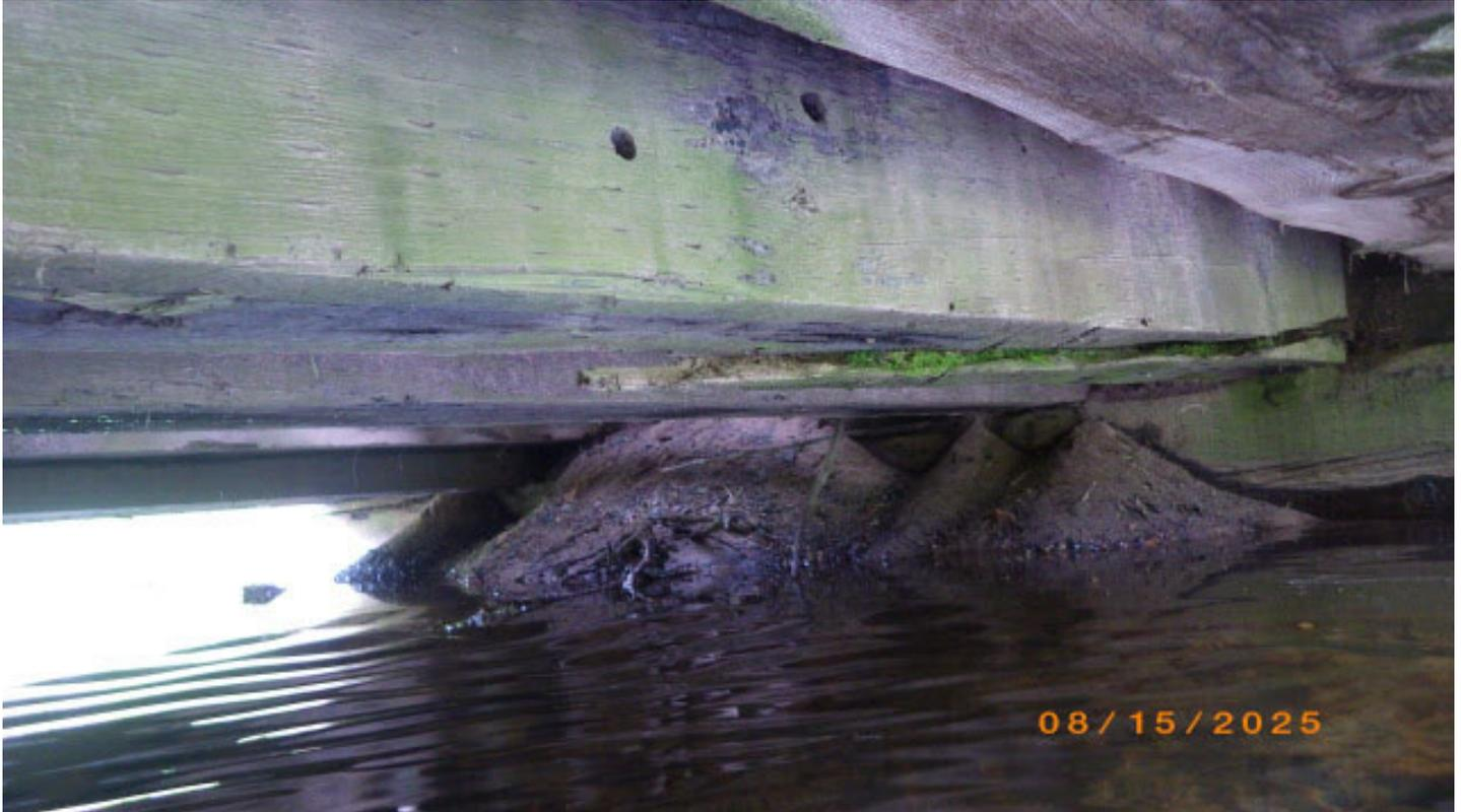
Girder 3 from downstream, completely rotten / cracked (east end)
