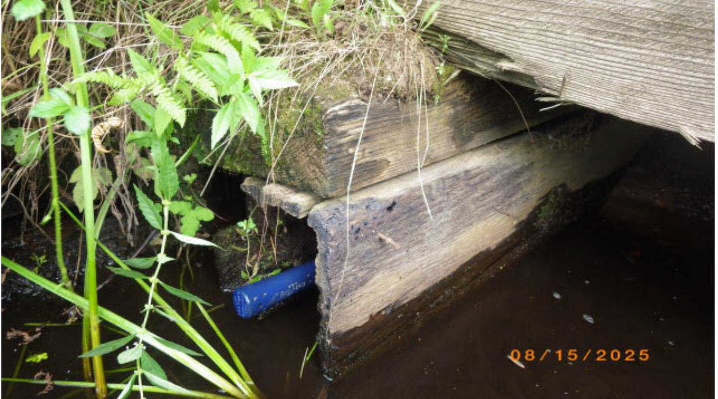
North end of east sill. Completely rotten / hollow but not crushing
