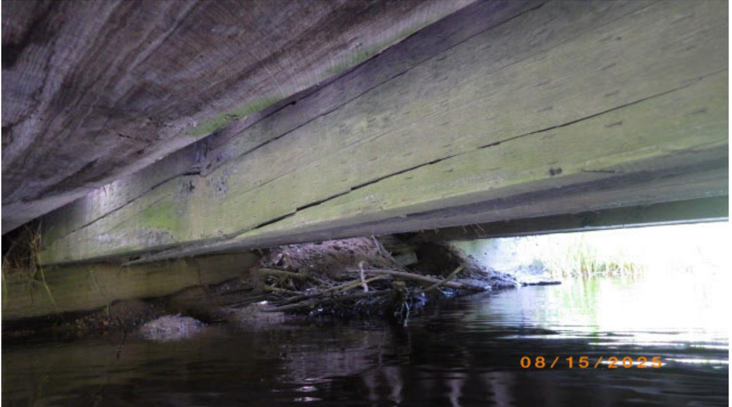
Girder 3 from downstream, completely rotten / cracked (west end)
