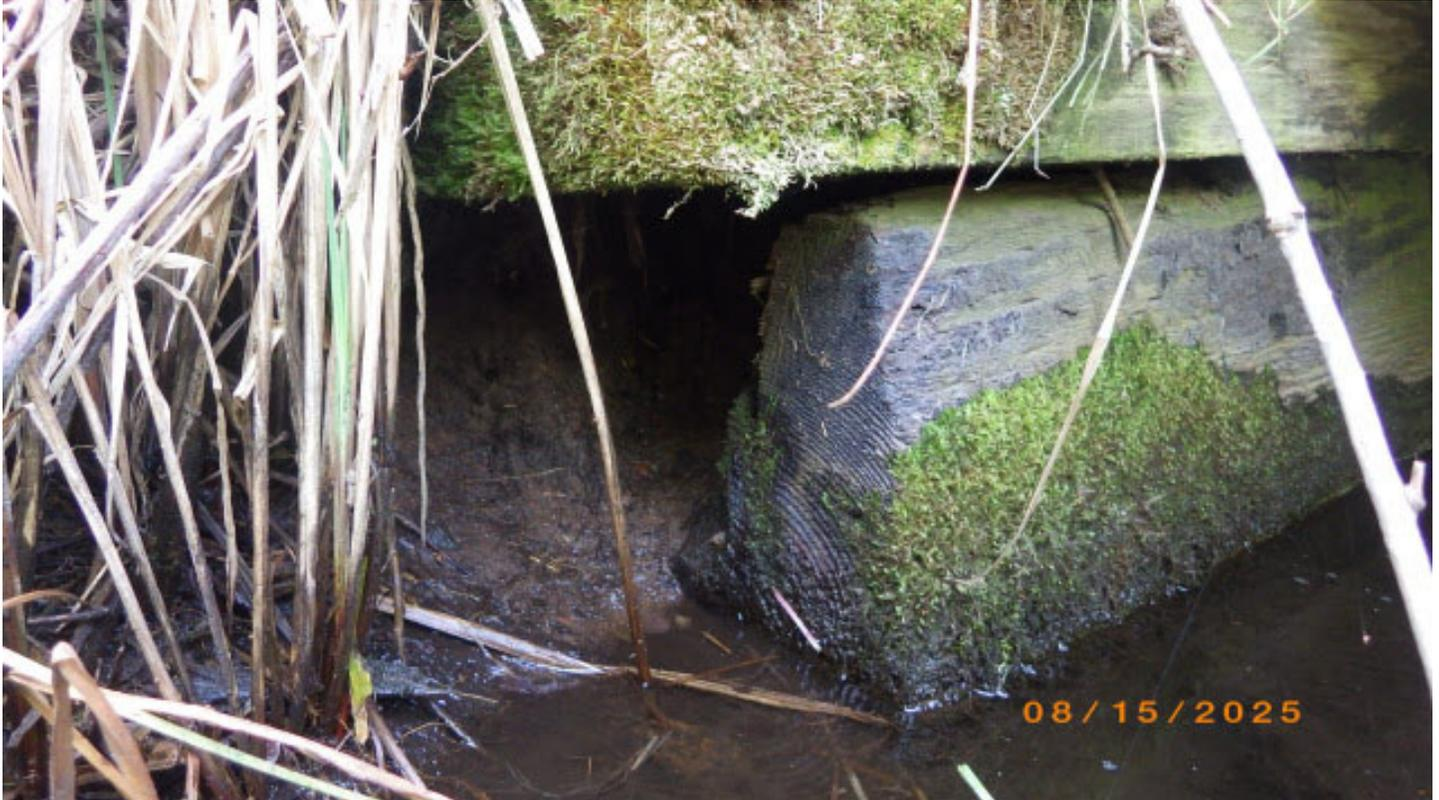
South end of west sill, completely rotten and hollow, but not crushing
