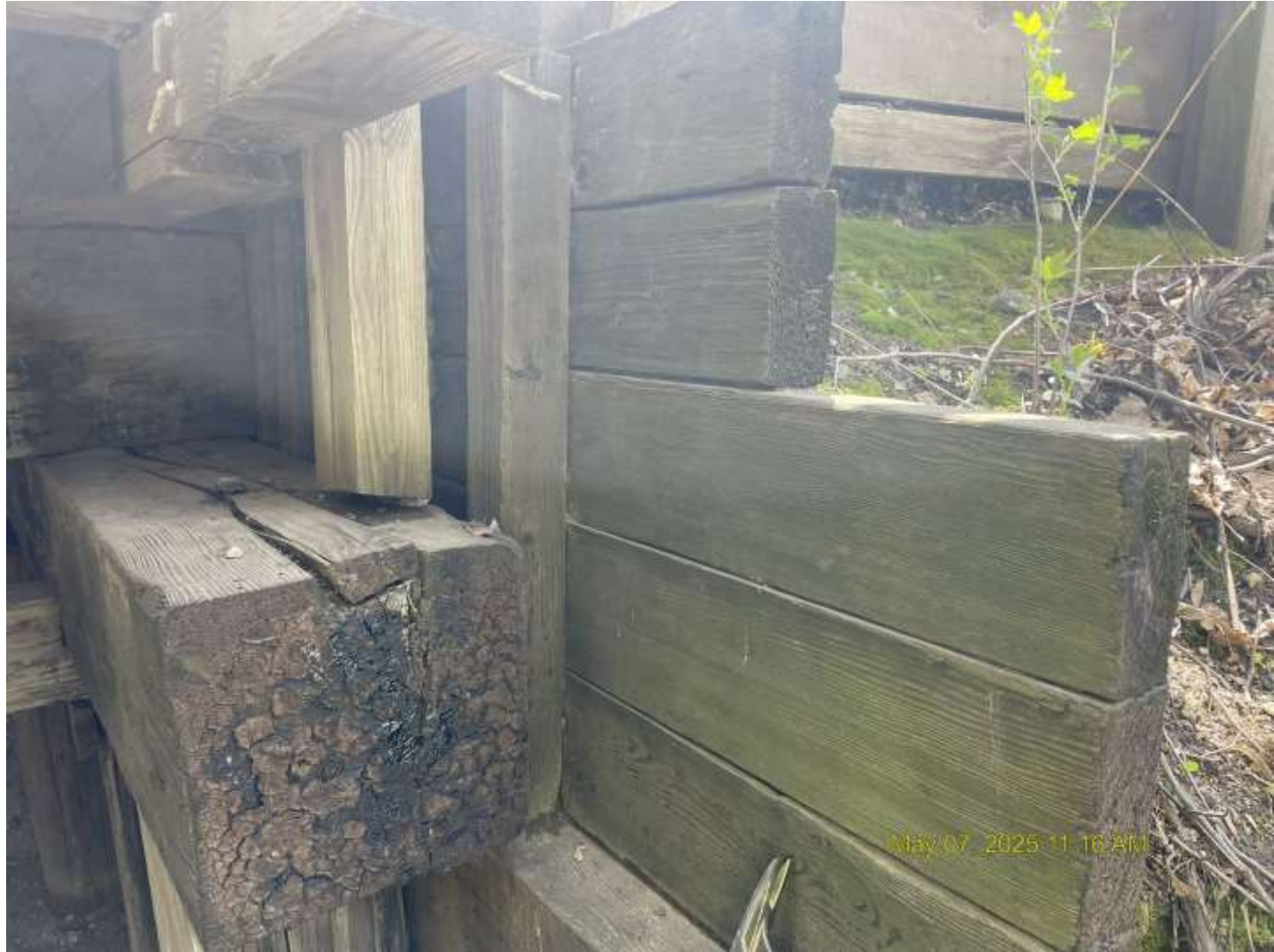
Looking at S. Abut. west side
