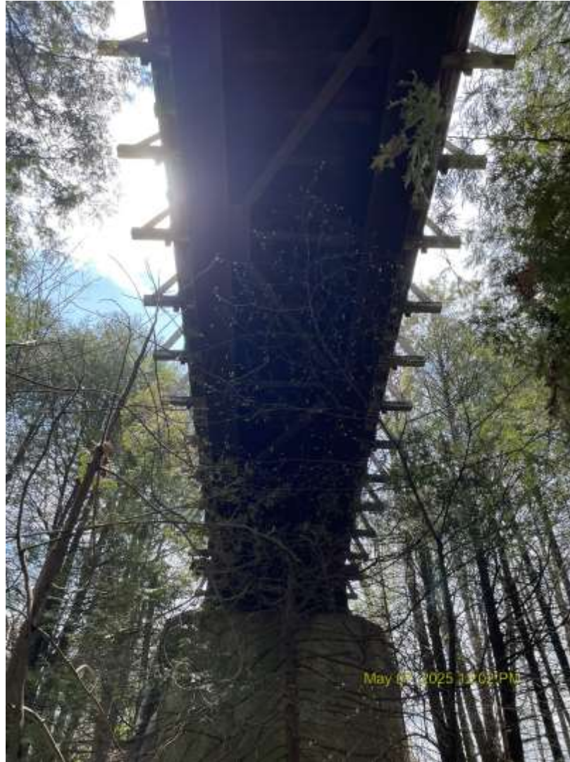
Looking up (south) at Pier 3
