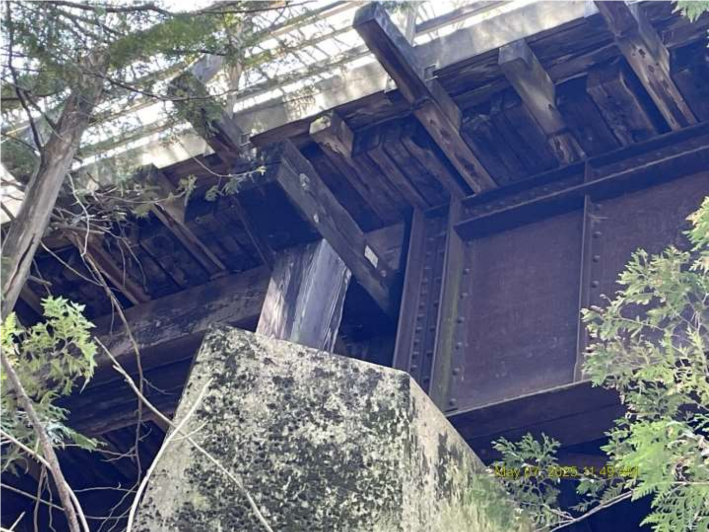
Pier 3 detail east side at girders
