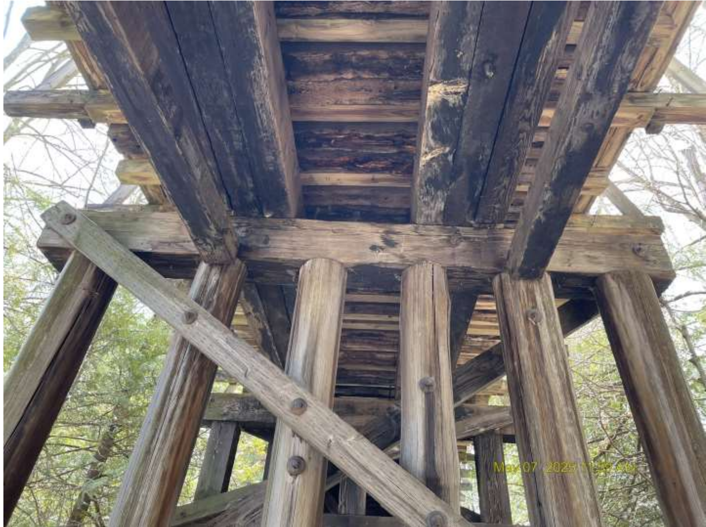
Looking south at Pier 5
