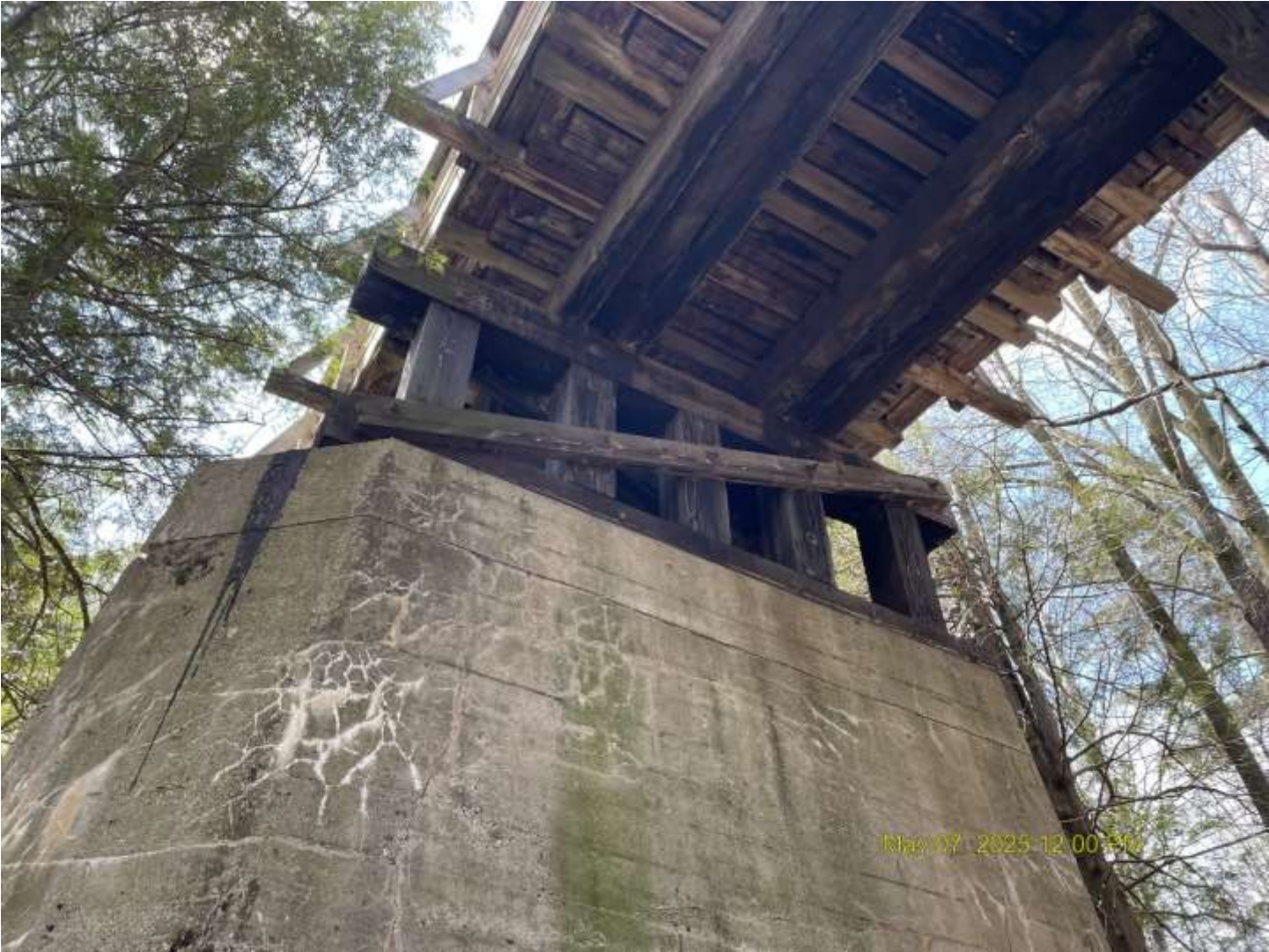
Looking up (south) at Pier 4
