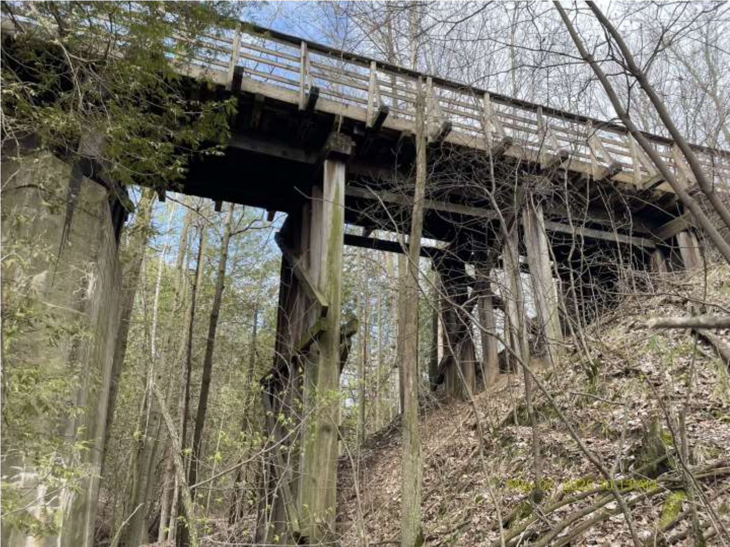
Looking west between Pier 4 and N. Abut.
