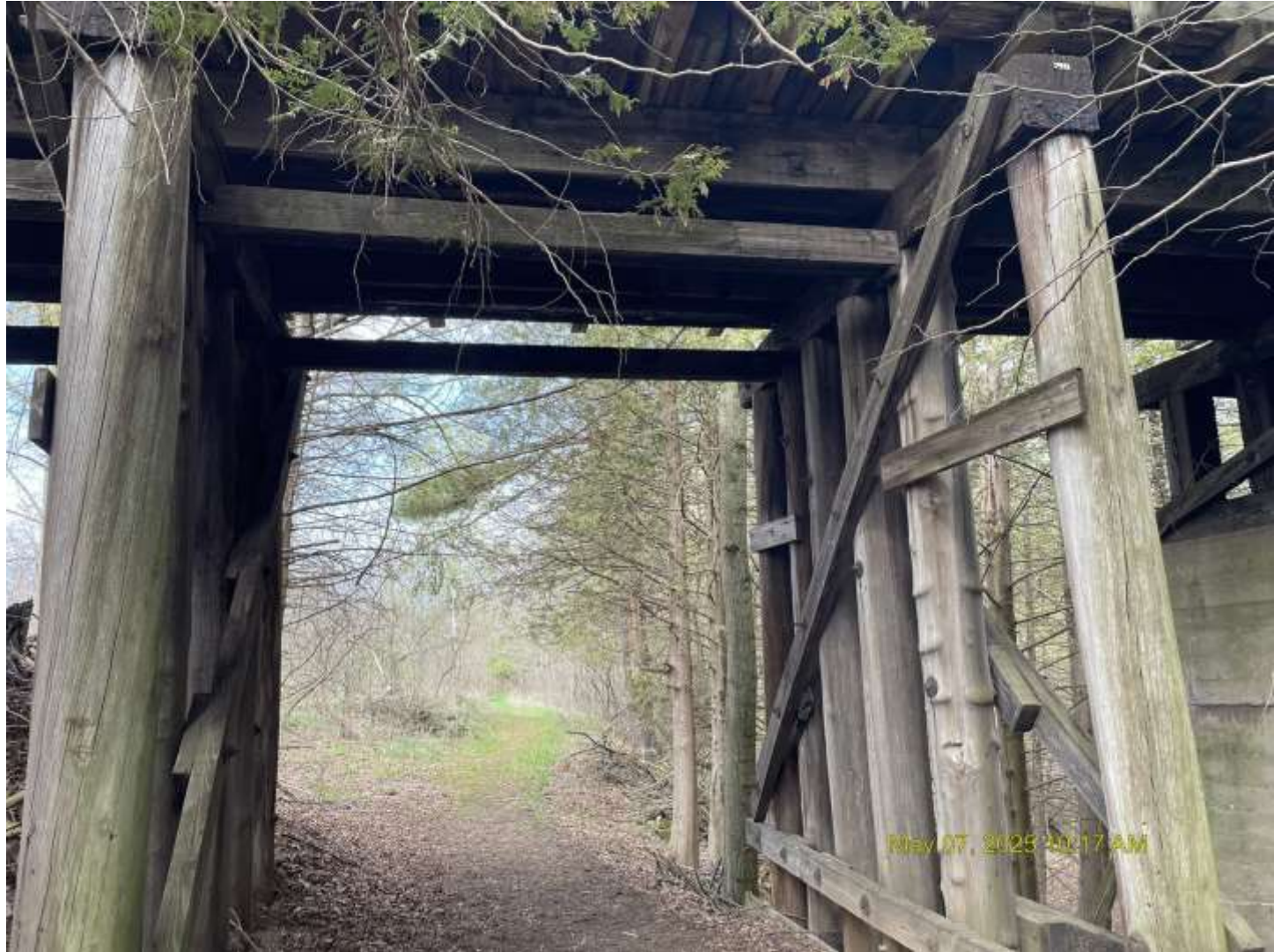
Looking west between Pier 1 & Pier 2
