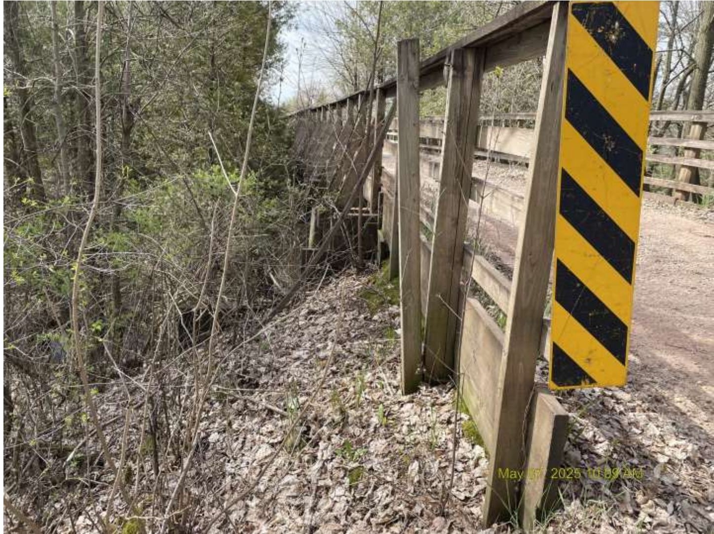
Looking south, east side of bridge
