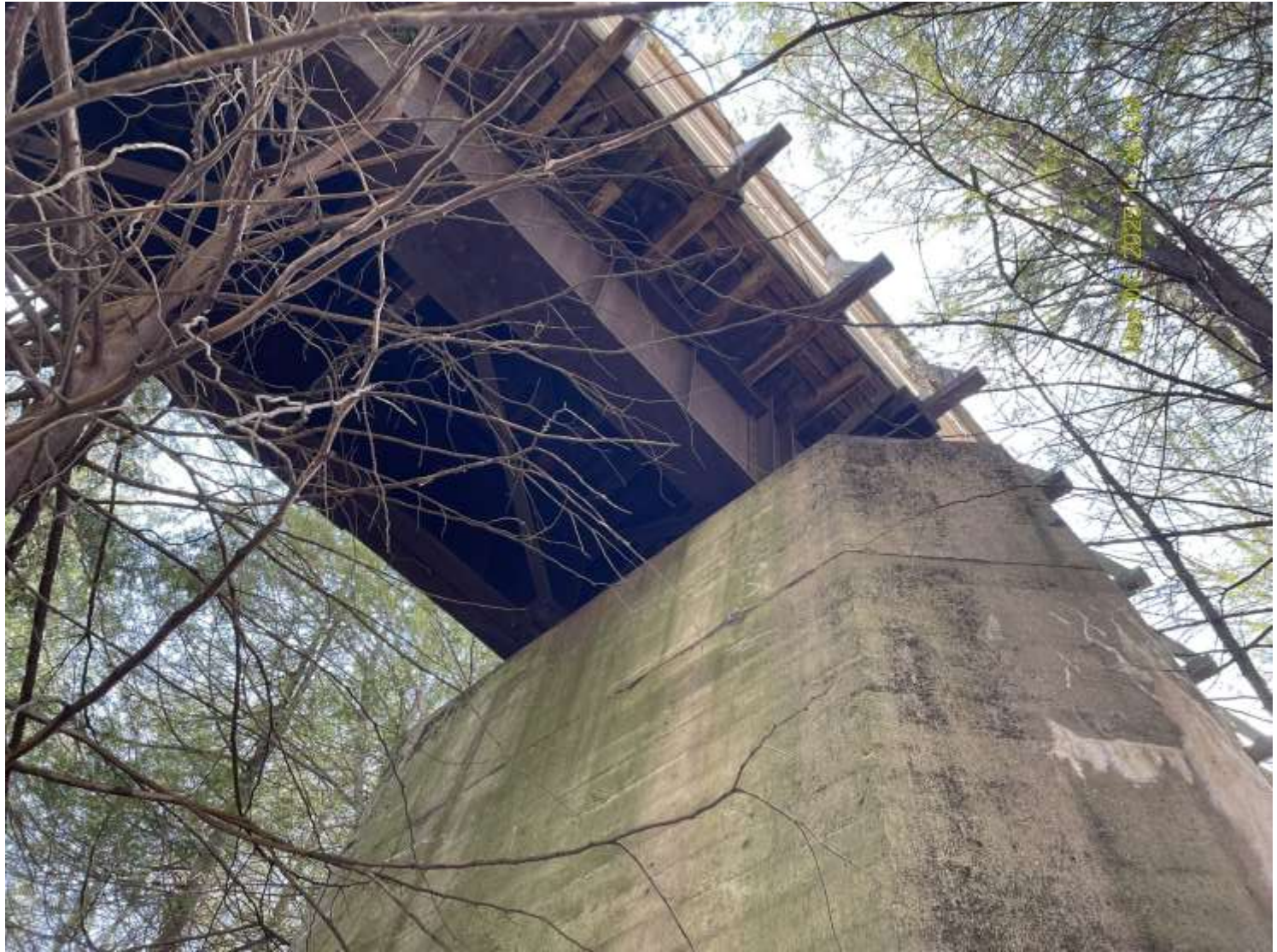
Looking up at Pier 3 (north side)
