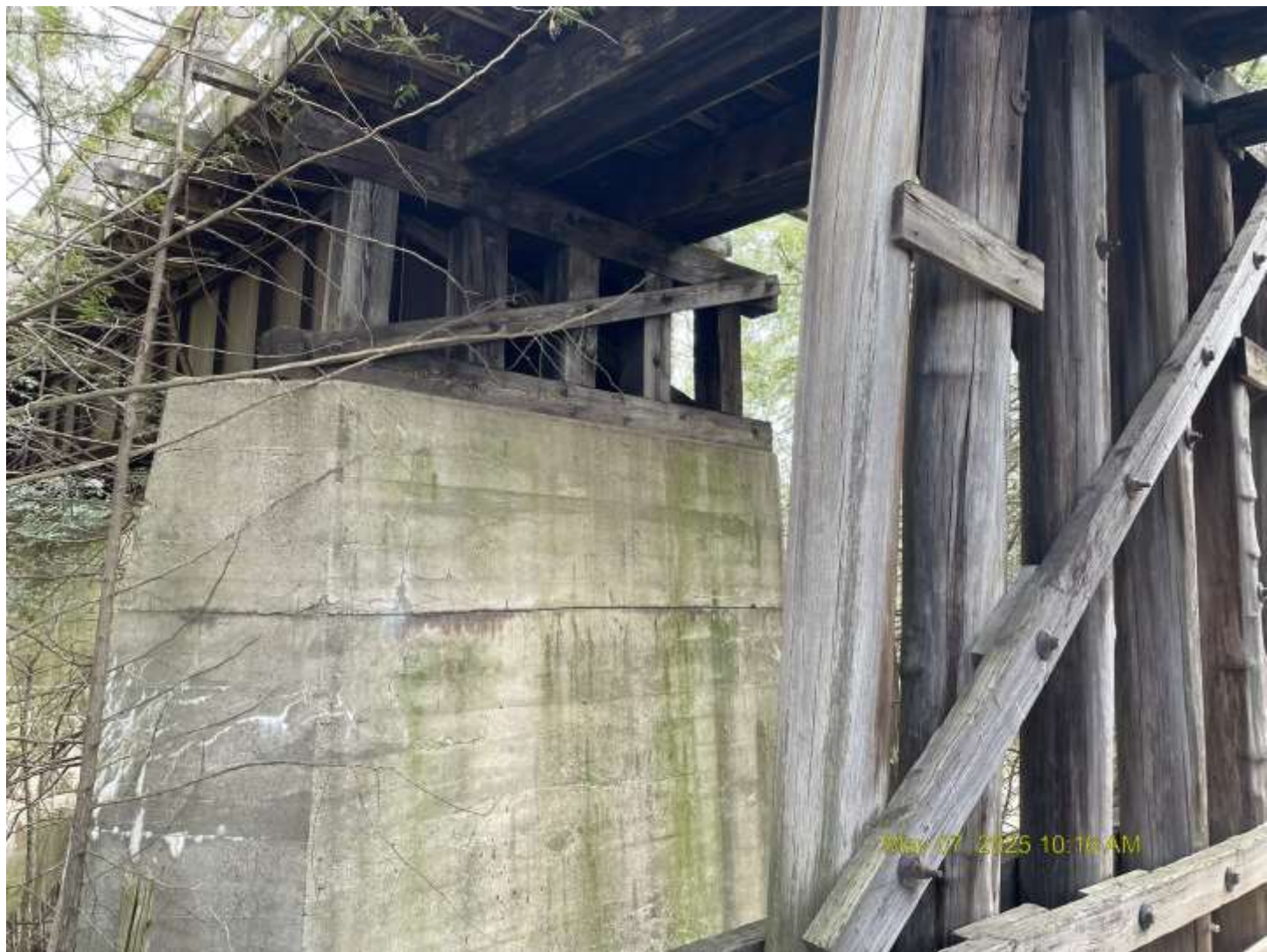
Looking NE between Pier 2 and Pier 3
