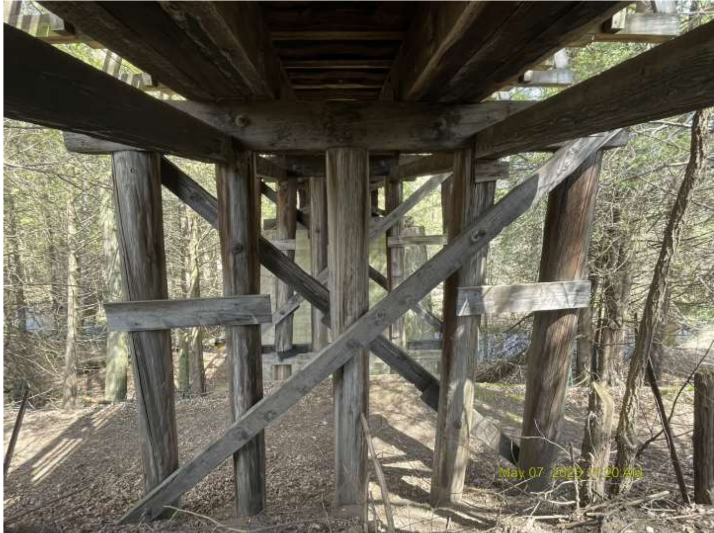
Looking north from south abutment
