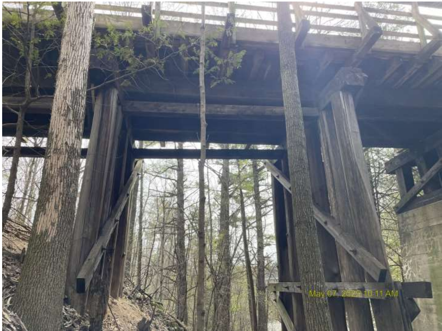
Looking east between Pier 6 and Pier 5
