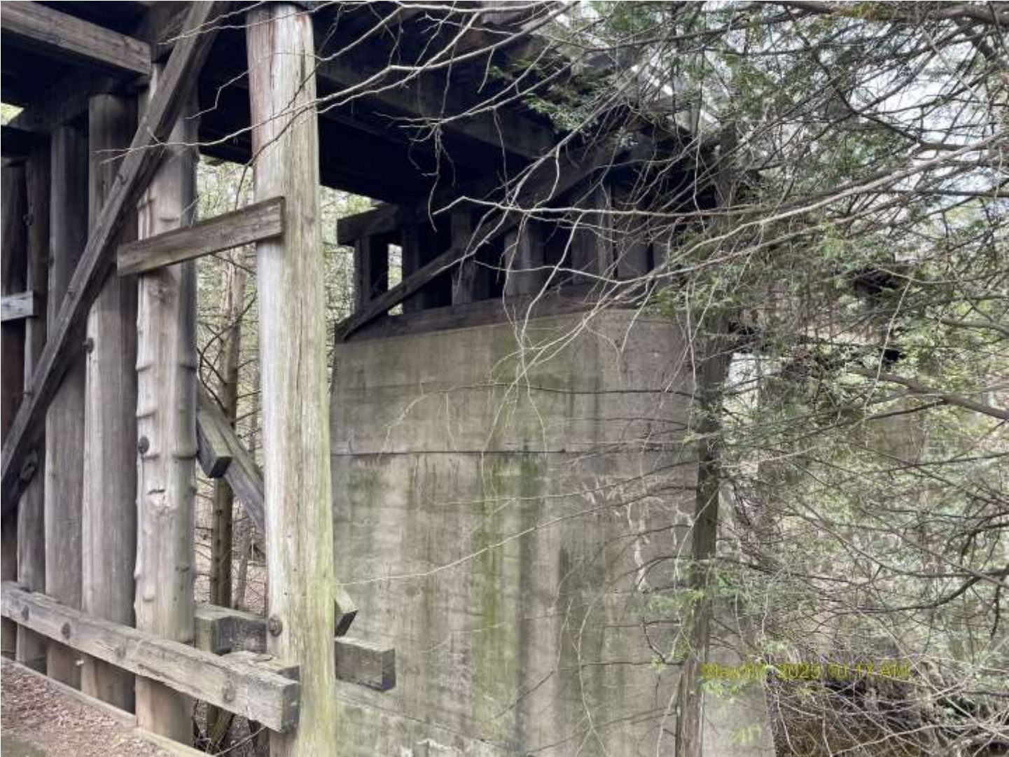
Looking NW between Pier 2 and Pier 3
