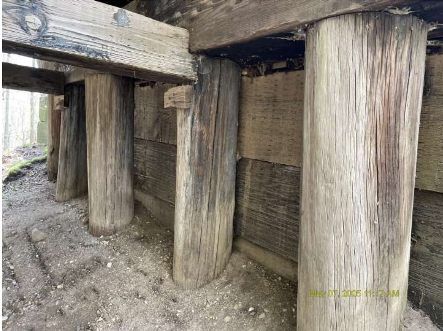
Looking at south abutment
