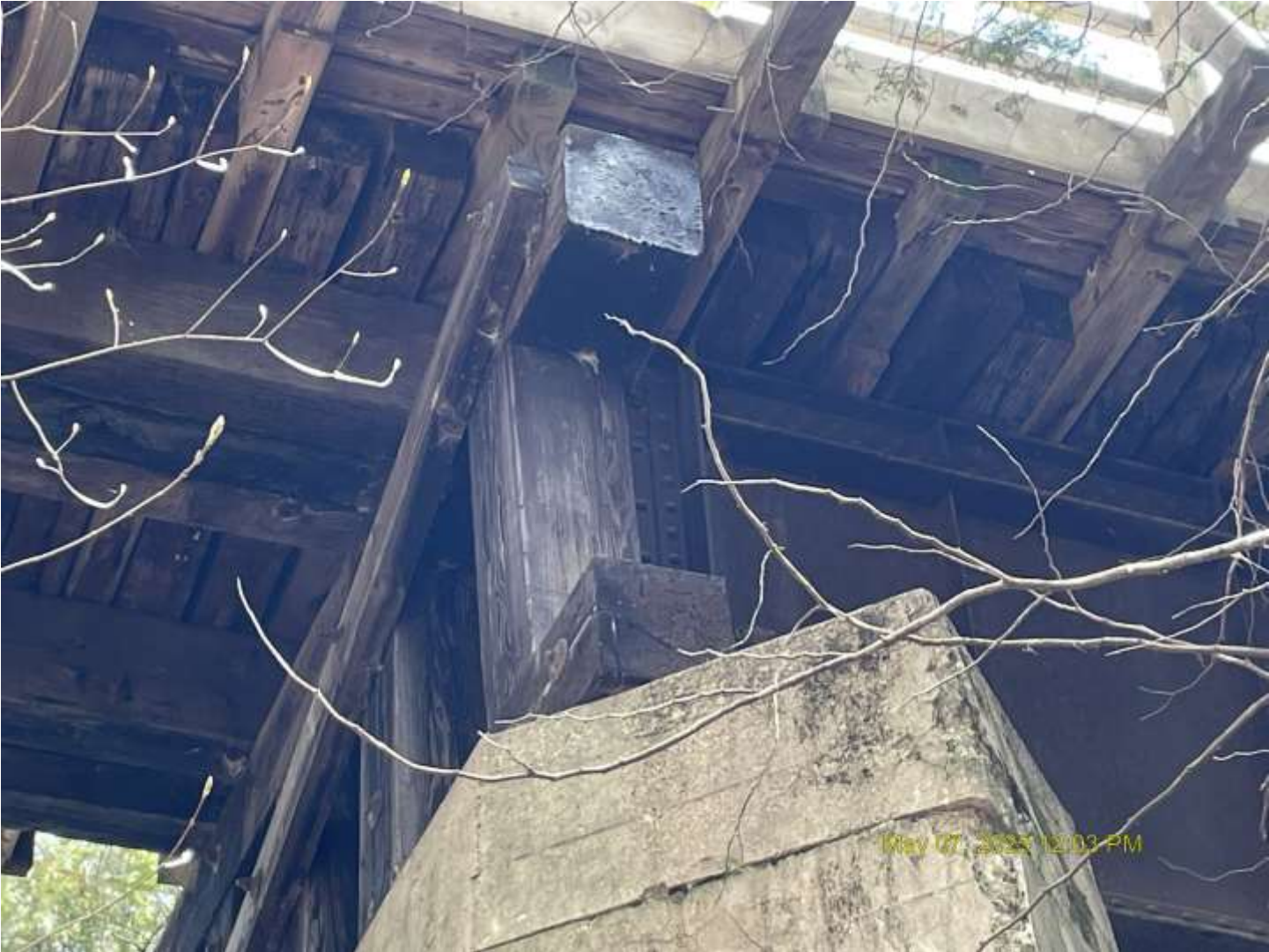
Looking up (east) at Pier 4
