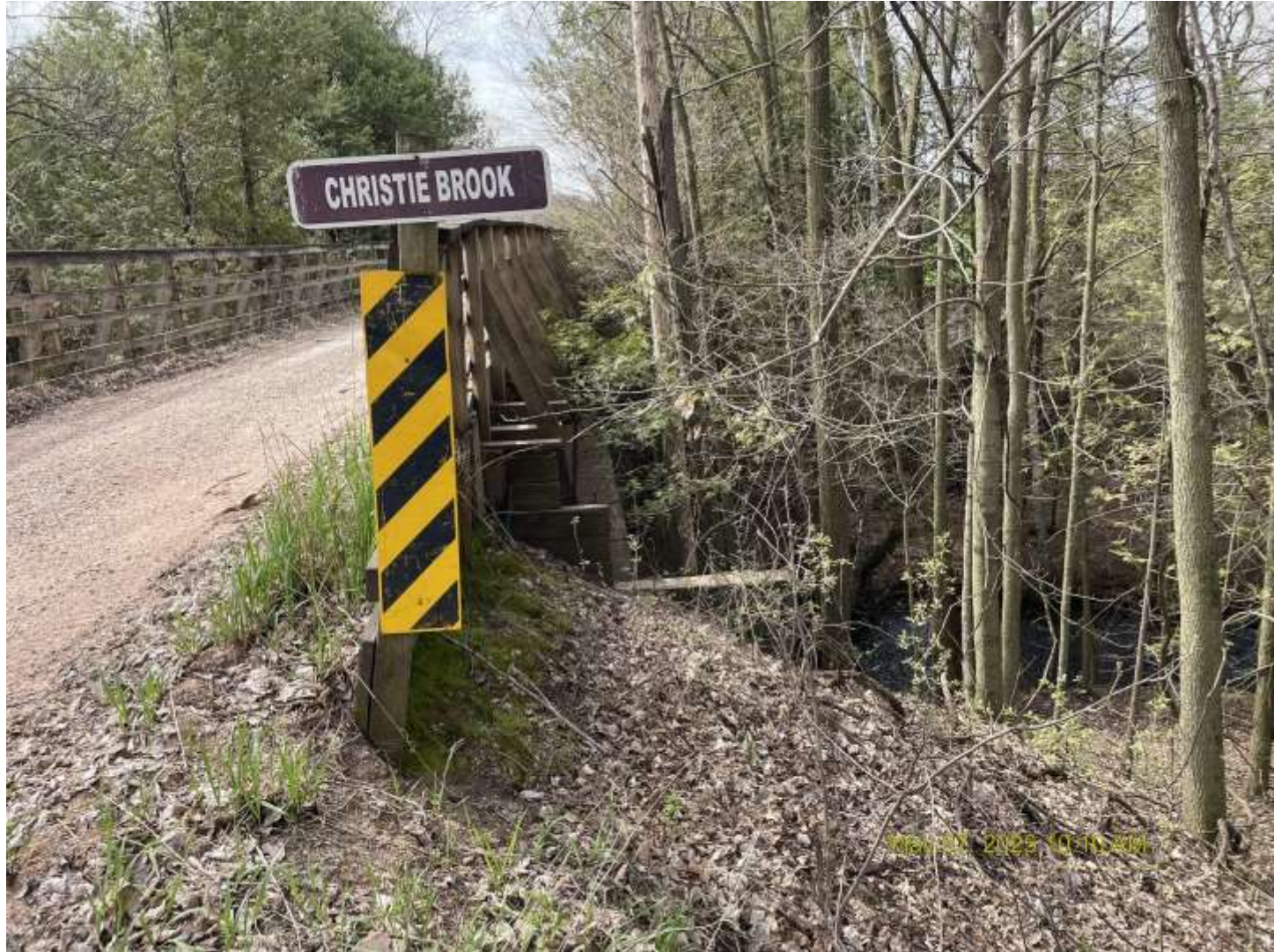
Looking south, west side of bridge
