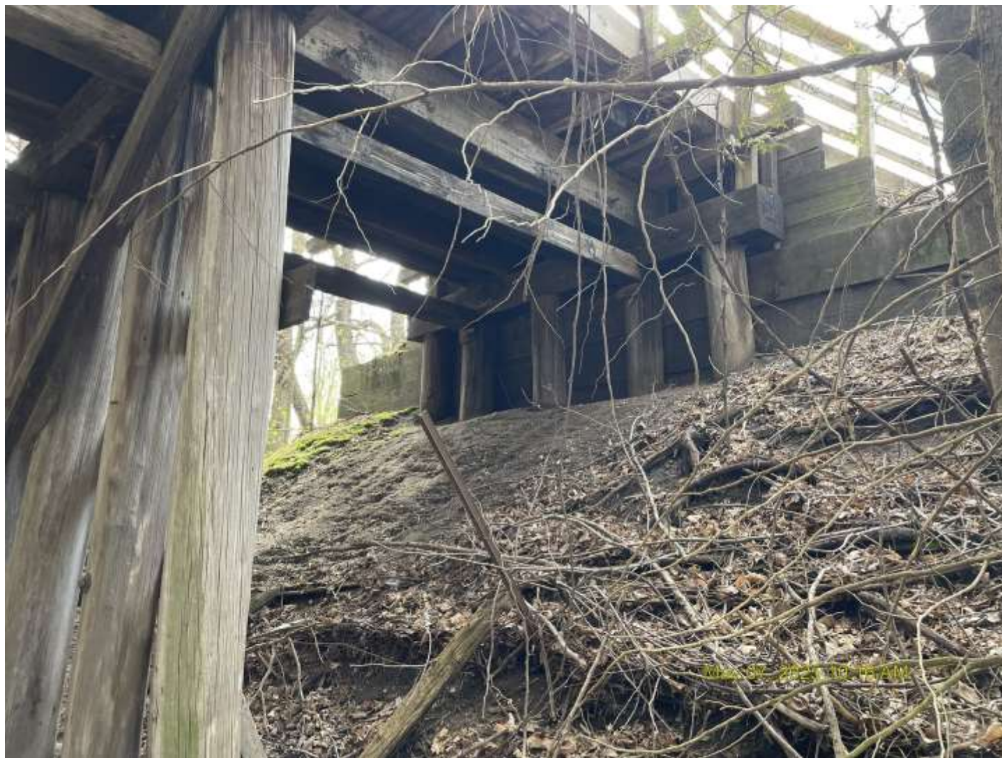
Looking SE between S. Abut. & Pier 1
