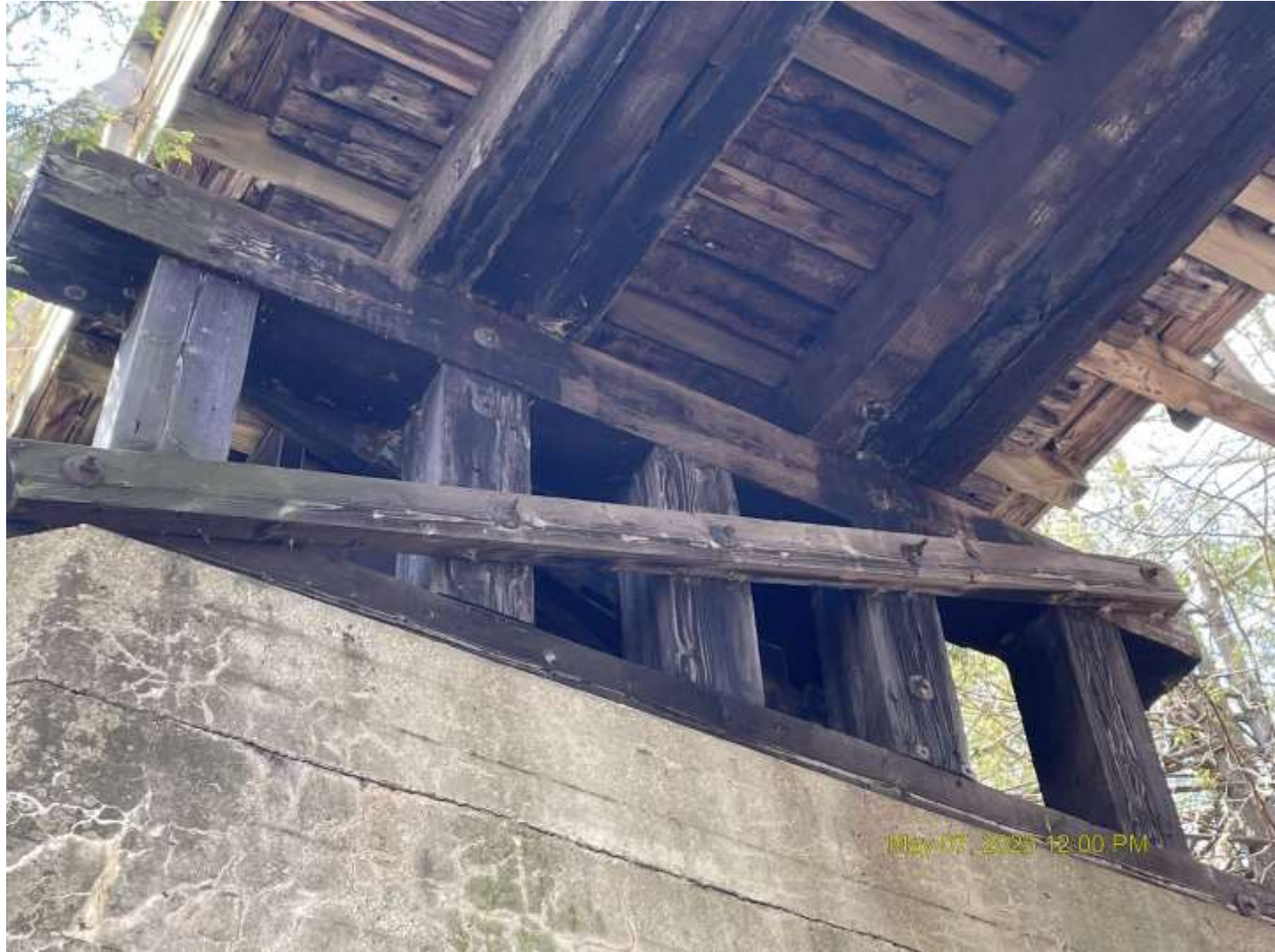
Looking up (south) at Pier 4 detail
