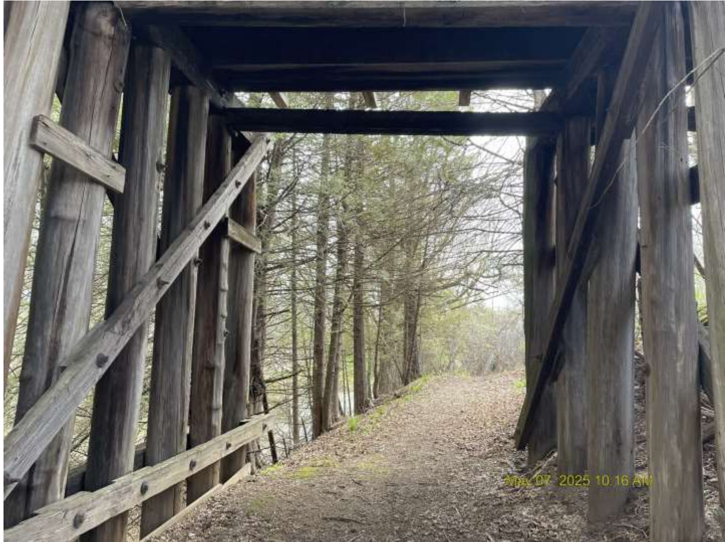
Looking east between Pier 1 & Pier 2
