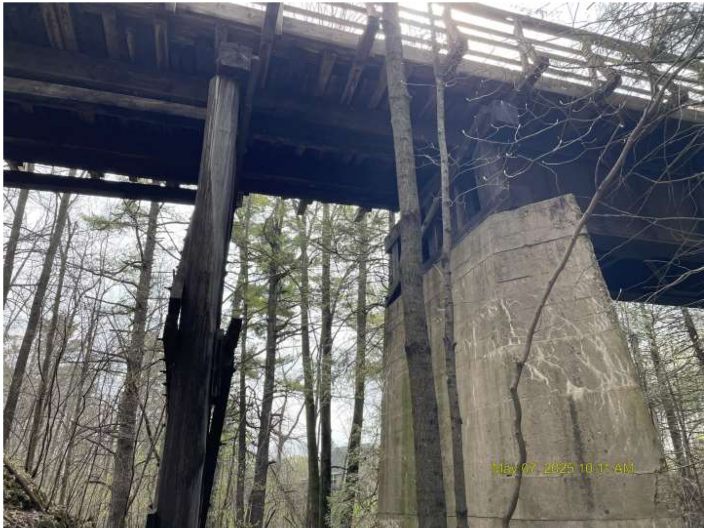
Looking east between Pier 5 and Pier 4
