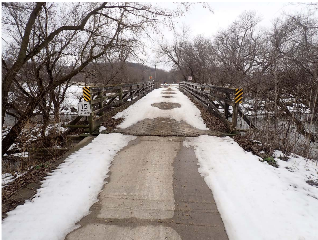
View of east approach, looking west.
