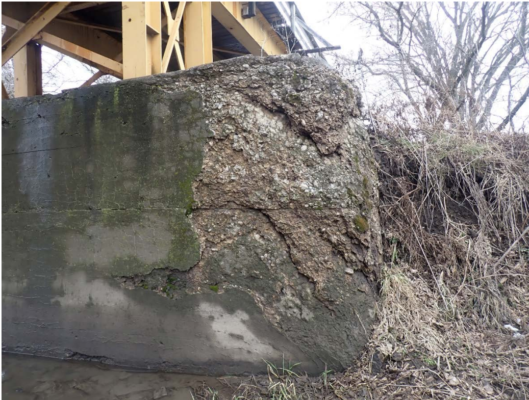
View of spalling on south pier nose, looking east.
