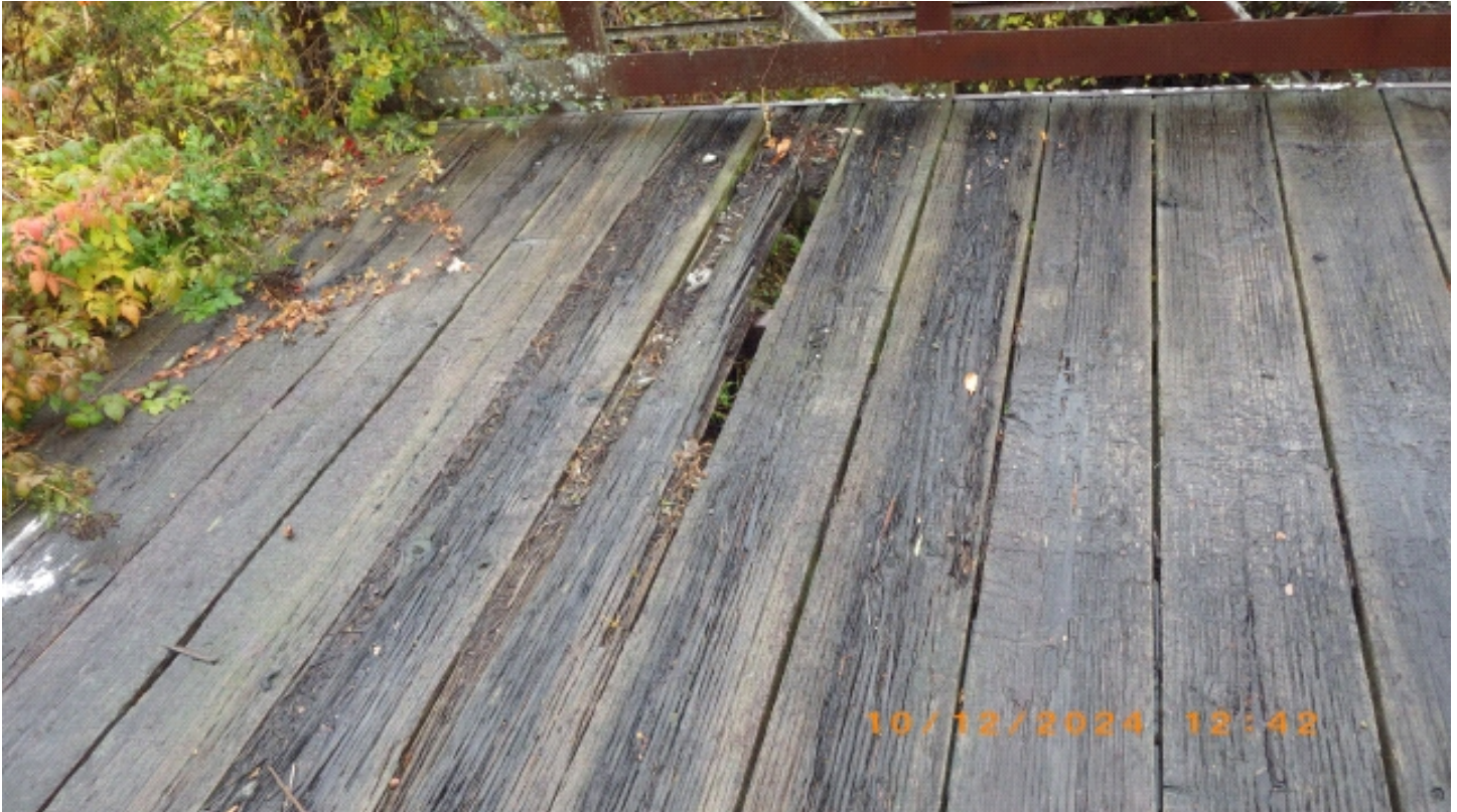
CS4 rotten deck planks
